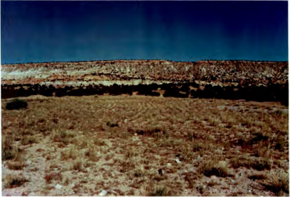
PHOTO 9 - Surface of Hope Mine site looking northwest. Note lines of revegetated grasses in center, earth mound over shaft at left center of view.
