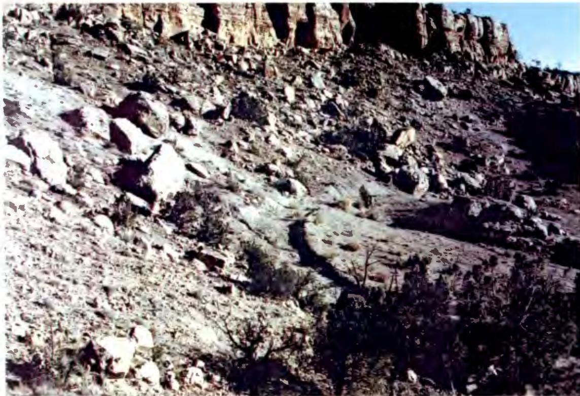
PHOTO 4 - Access road to Doris main decline, regraded to divert runoff from mesa slope.
