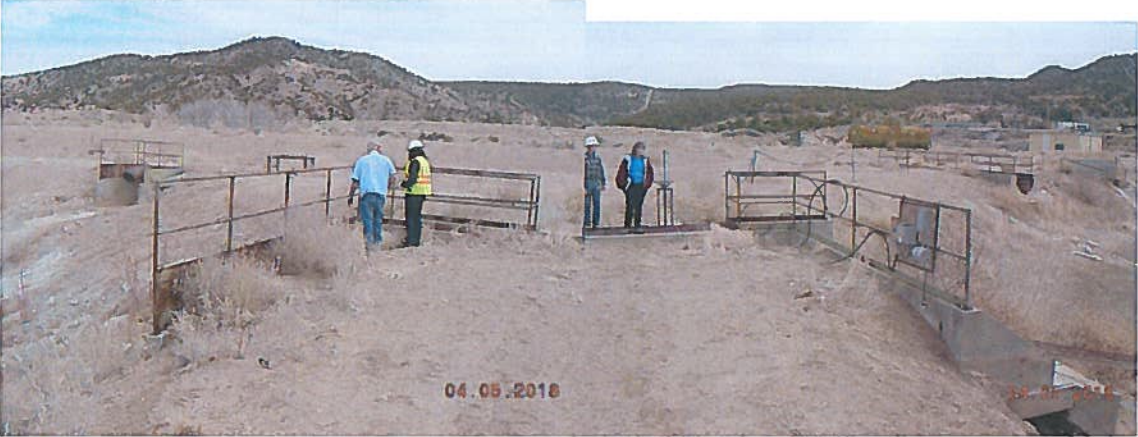
Concrete Connection Culvert between Pond 2 and 3
