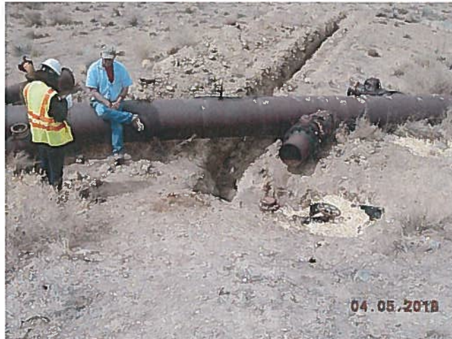
Pipelines and Excavated Interconnection to Ponds
