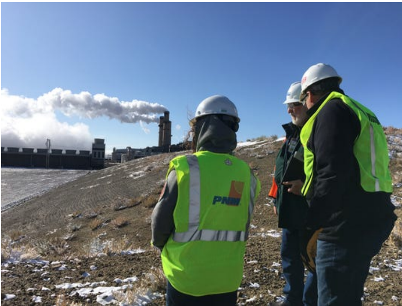
Marcel Nanasi, Mark Hutson and Norman Norvelle look at a sealed pond, Monday, Oct. 28, 2019, at San Juan Generating Station in Waterflow. (Photo: Hannah Grover/The Daily Times)
