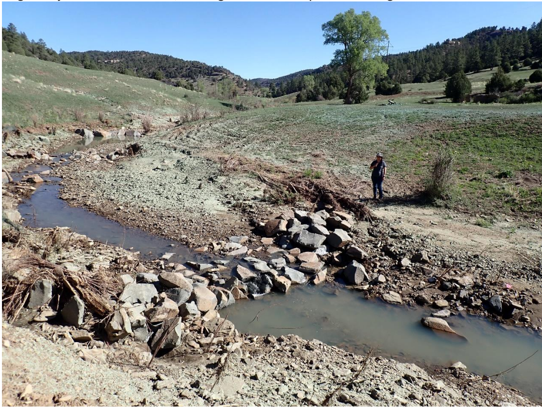
Structures doing their job after rain events, moving the flows away from eroding banks
