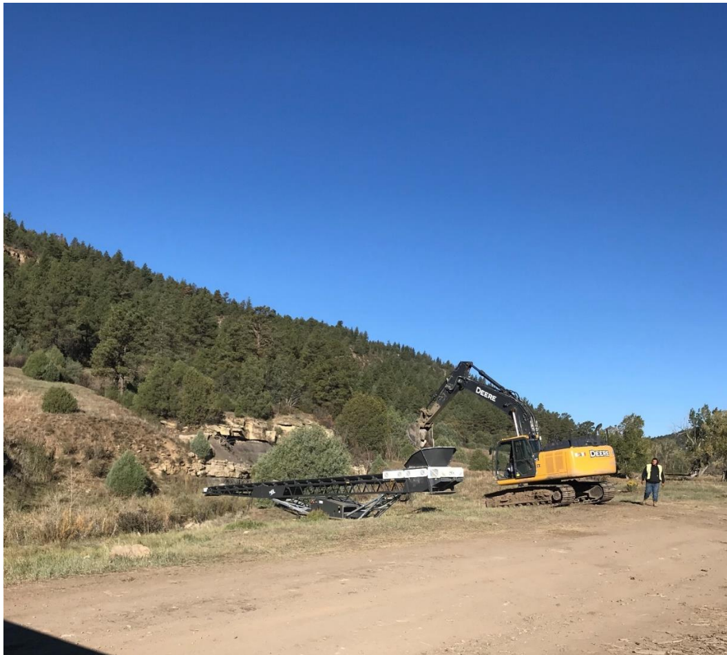
Figure 7. Conveyor belt being used to drop boulders into place in the stream channel across an archaeological avoidance area.
