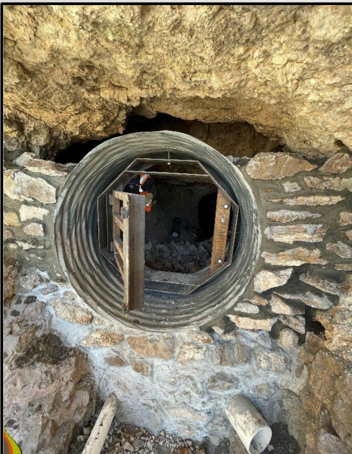
Construction of a culvert with bat gate in a rock bulkhead design. A 48" culvert was utilized on this feature to maximize the airflow for bats.
