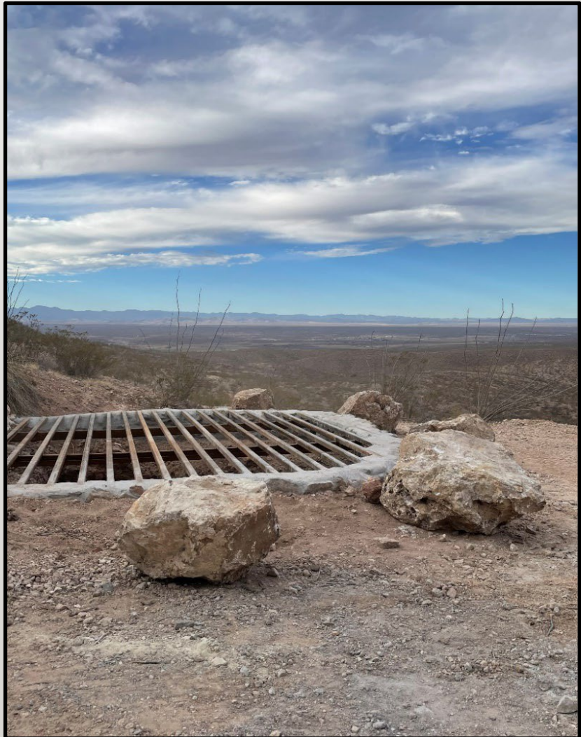
Vertical shaft safeguarding located immediately adjacent to popular off-road trail.
