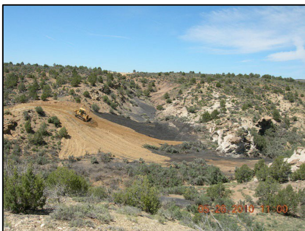
Photo 1.) Previous AML Program Abatement at Jones Mine Looking South (2010)
