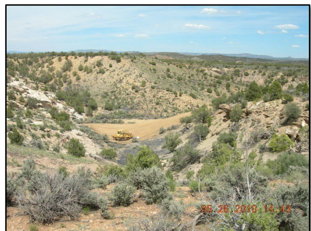
Photo 2.) Previous AML Program Abatement at Jones Mine Looking North (2010)
