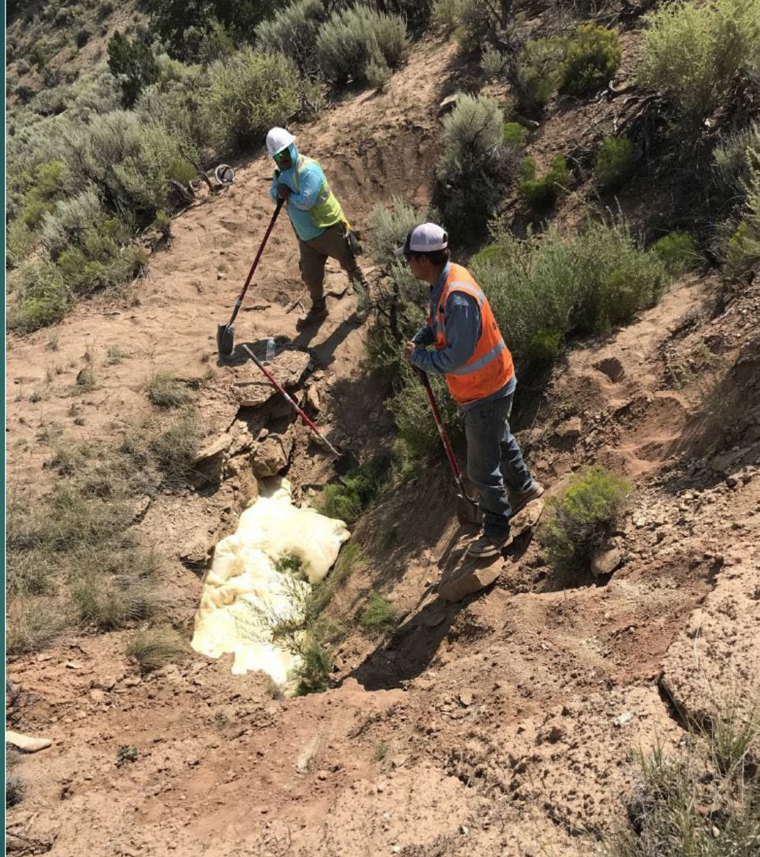
Three small coal subsidence openings were filled with PUF and then backfilled. Only one of the three is pictured above. Features were then mulched, and a native seed mixture was broadcast over the disturbed area.
