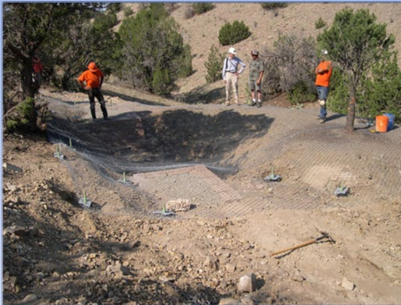
Installation of high-strength steel mesh with rock anchors. Note the partially completed bridge abutments on two sides of the shaft opening.
