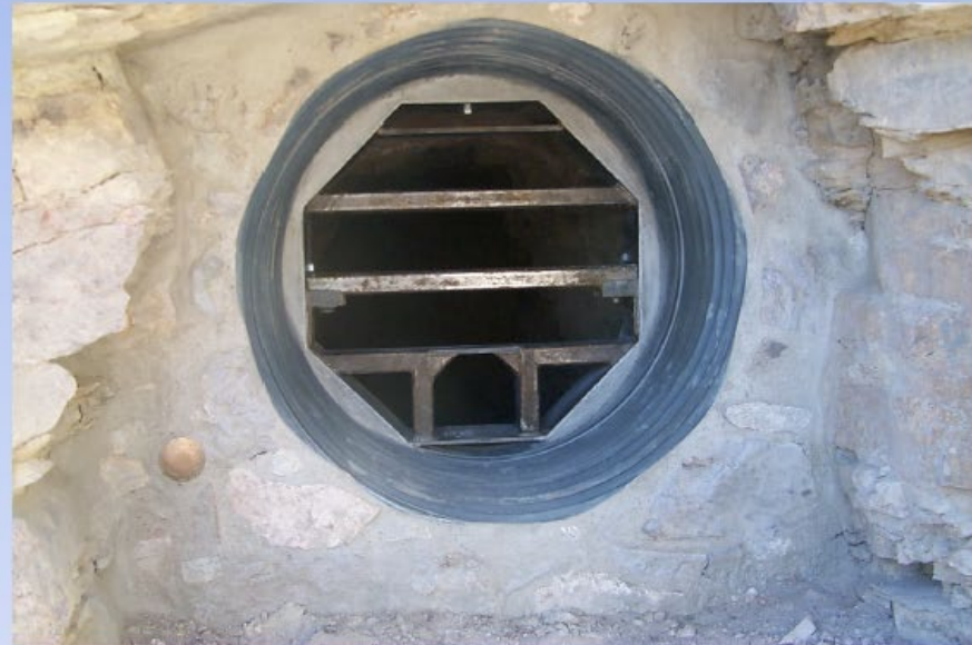
Culvert with bat and wildlife-friendly gate
