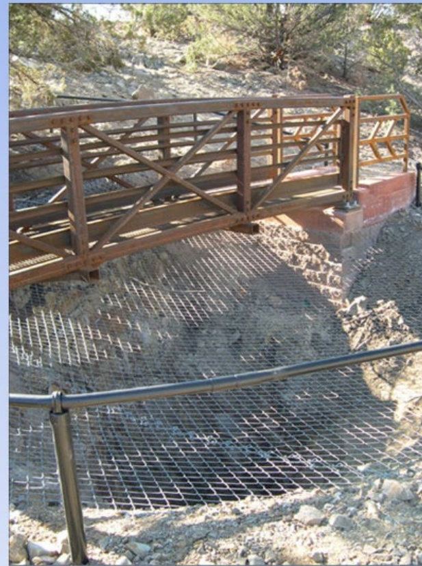
The completed mesh and bridge installation over a shaft (Cerrillos Hills State Park)
