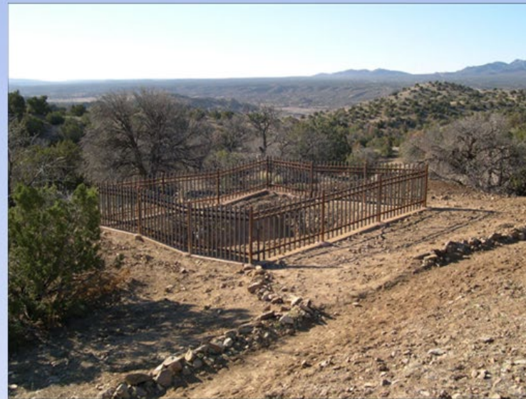
Weathered steel picket fence enclosure around a partially filled shallow shaft (Cerrillos Hills State Park)
