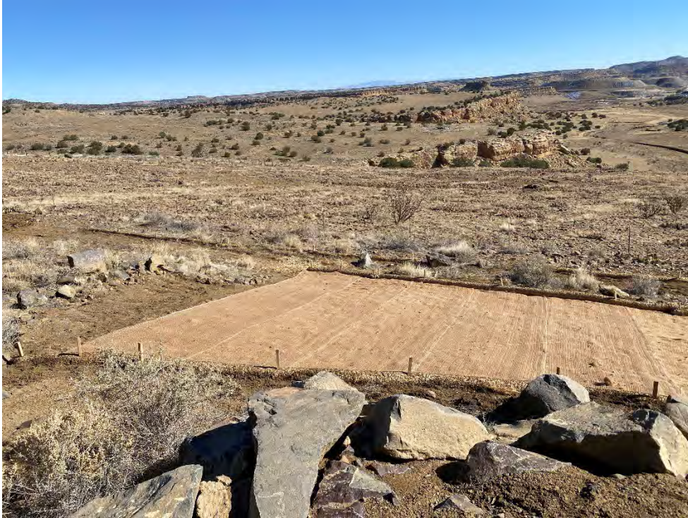
Photograph 29. View of installed biodegradable seed mat at Reclaimed VS-6.
