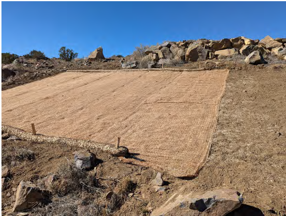
Photograph 17. View of biodegradable erosion control blanket and Eco Log, as installed down slope from VS-6 (11-05-2024).
