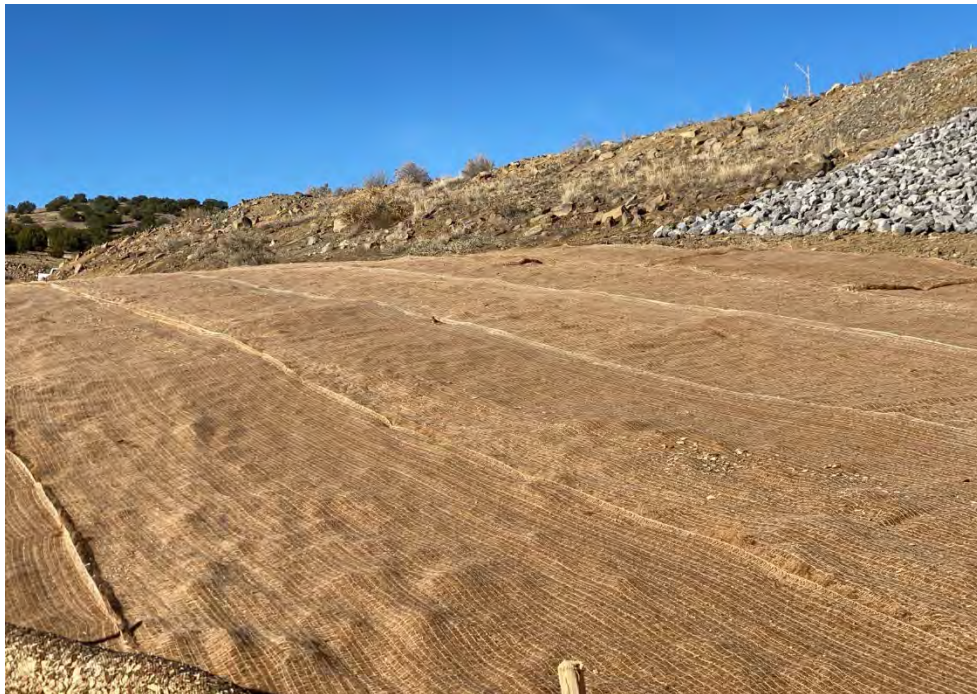
Photograph 49. View looking northwest from the area reseeded below the armored slope at the reclaimed VS-10 area. The area was roughened, reseeded, then covered with the biodegradable matting. Eco Log fiber rolls were placed on the downslope edge of the matting.
