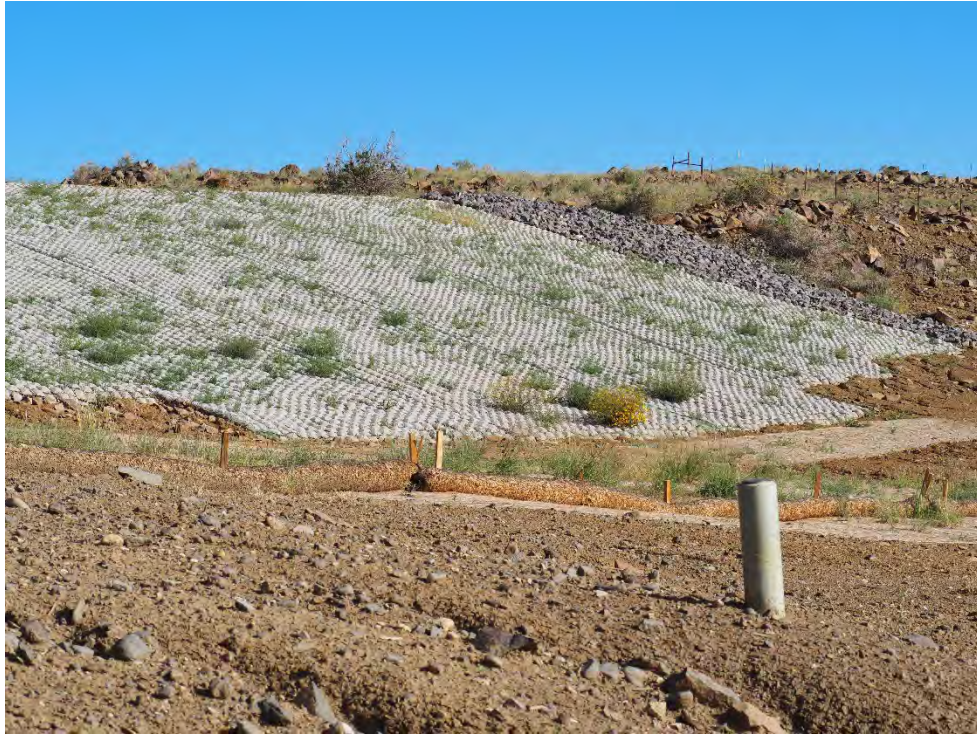
Photograph 90. Northwestern view, from the VS-10 monument, of the regraded, armored slope located at the transition from the reclaimed former borrow area to the reclaimed VS-10 (September 2025).
