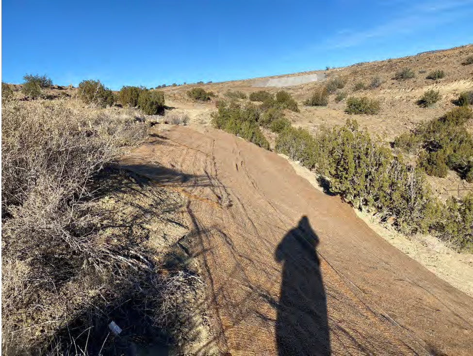
Photograph 54. View looking northwest from the reseeded lower slope at the reclaimed VS-12 area. The area was roughened, reseeded, then covered with the biodegradable matting.
