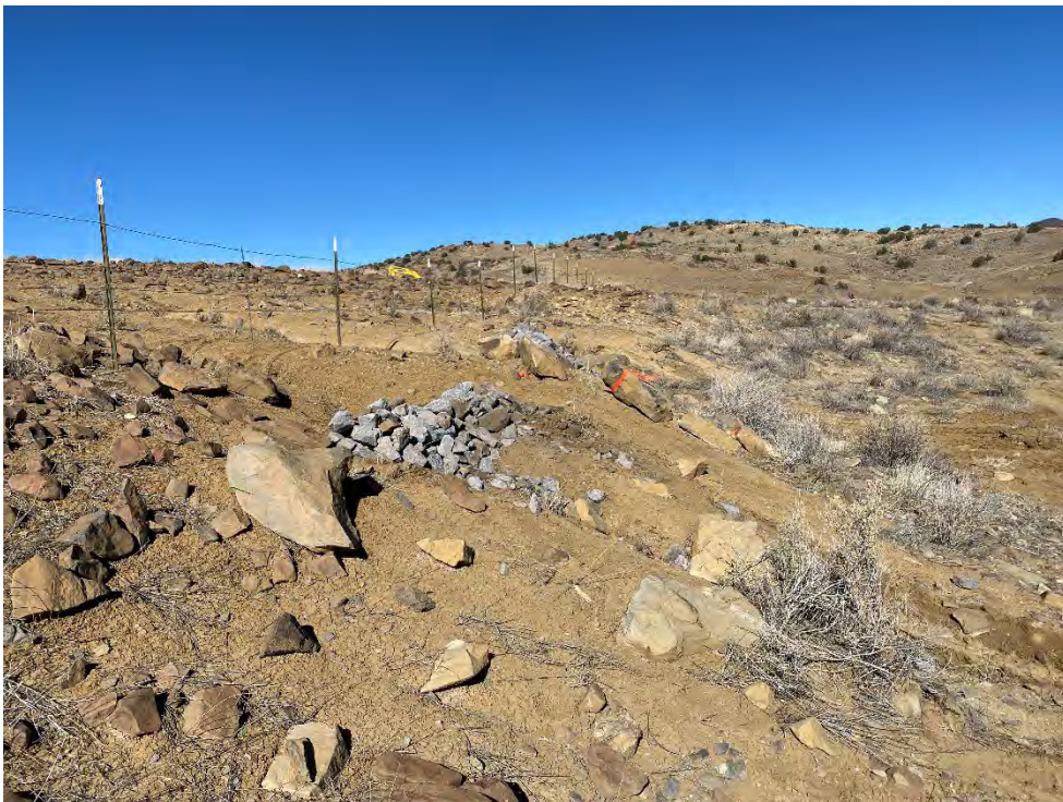
Photograph 30. View of installed biodegradable seed mat at Reclaimed VS-6.
