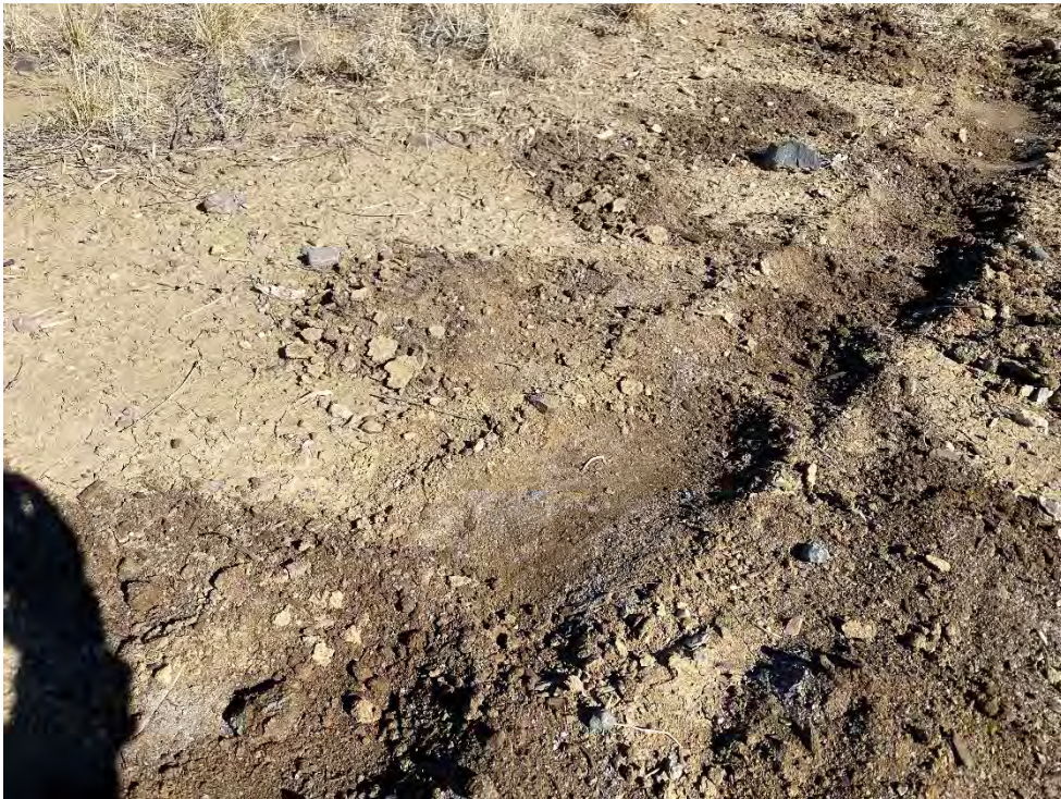
Photograph 69. Eco Log fiber rolls were keyed into the surface and installed along the contours of the slope.
