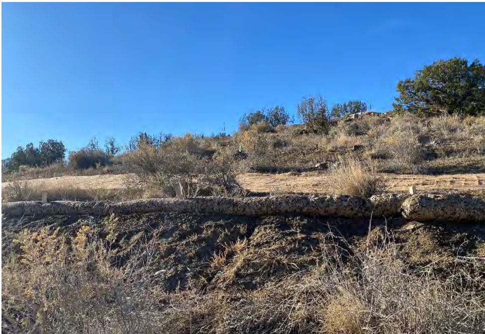
Photograph 55. Eco Log fiber rolls were placed on the downslope edge of the matting at the reclaimed VS-12 area.
