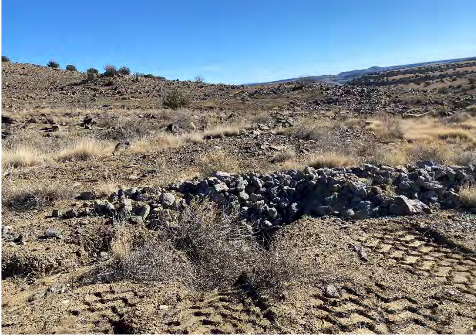
Photograph 64. Rock check dam maintenance utilizing on-Site available materials at reclaimed VS-10 area.
