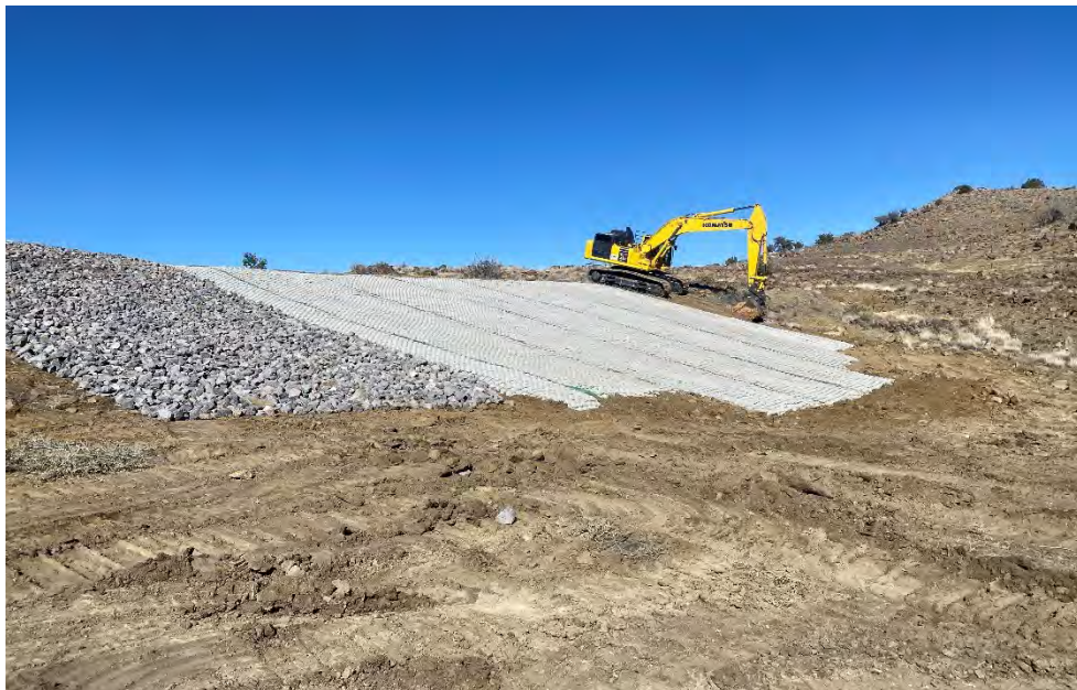
Photograph 46. Regrading was accomplished utilizing existing on-Site material present on the western edge of the slope. Due to the movement of this material, additional rock was installed to armor the exposed slope following reseeding methods. View looking to the north-northeast.
