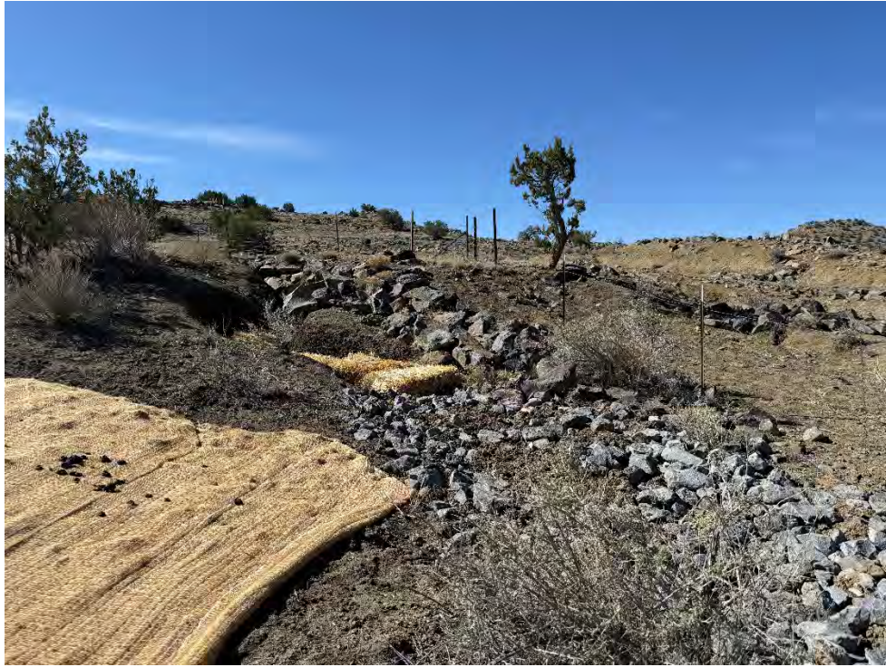
Photograph 74. View of slope armored channel at reclaimed VS-4, with strawbale and biodegradable matting (April 2025).
