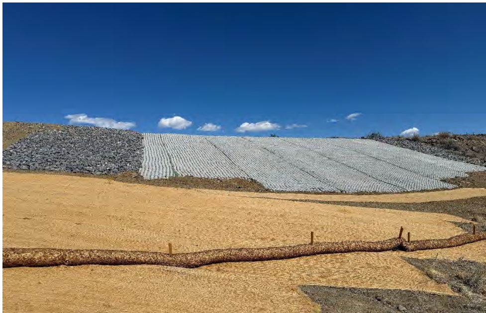
Photograph 79. Northwestern view, upslope, of the regraded, armored slope located at the transition from the reclaimed former borrow area to the reclaimed VS-10 (April 2025).
