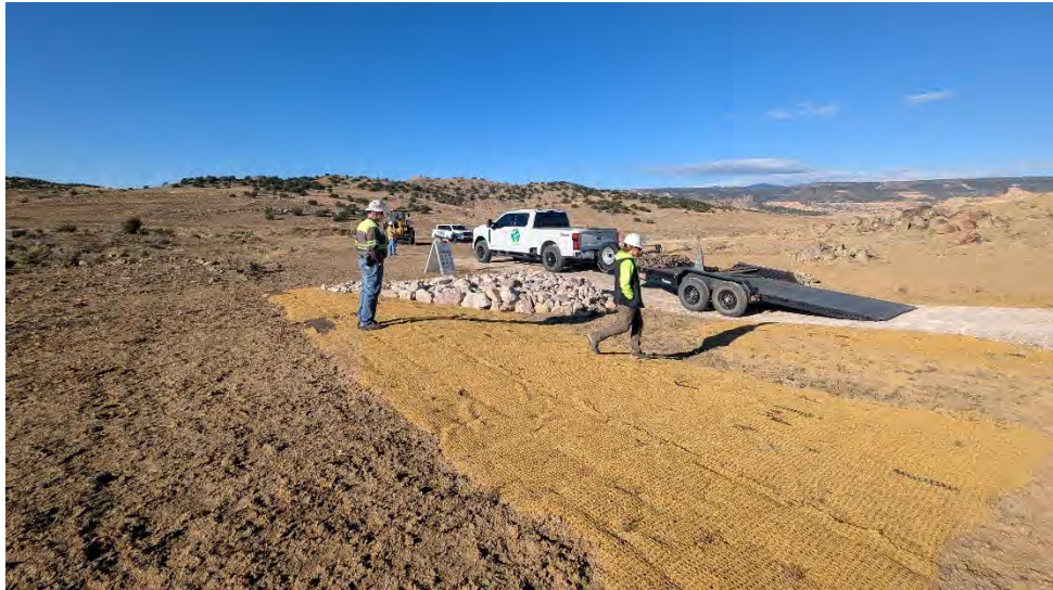
Photograph 1. Start of mobilization activities, October 29, 2024. Low Water Crossings—installed by the Department of Energy, which manages the L-Bar Site—impacted equipment transport to the staging area, near the No. 1 mine shaft.
