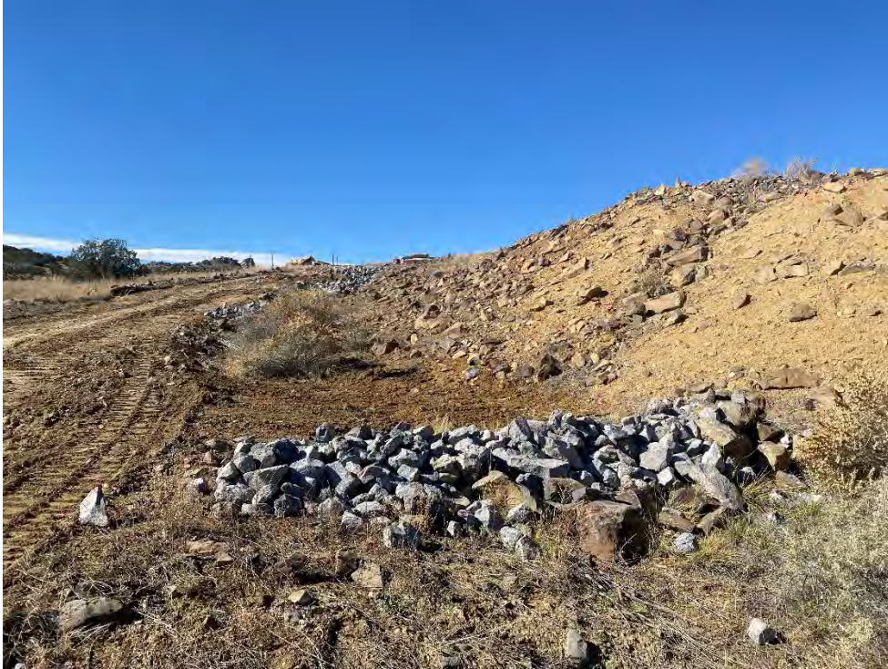
Photograph 47. View of bolstered rock check dams, installed and repaired at Reclaimed VS-10.
