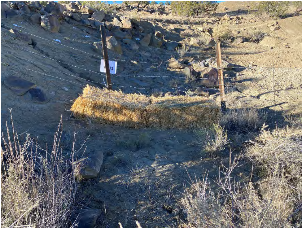
Photograph 57. Strawbales were placed within channels along the drainage on the eastern side of the Reclaimed VS-12 area.
