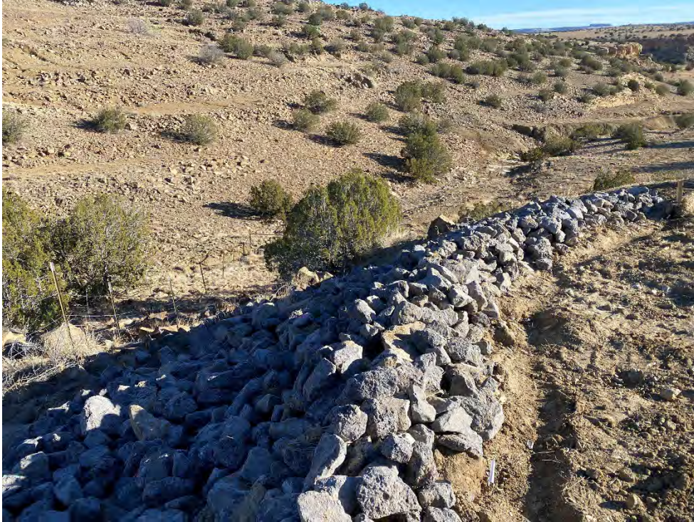
Photograph 58. View looking east-northeast from the armored channel at the reclaimed VS-12 area.
