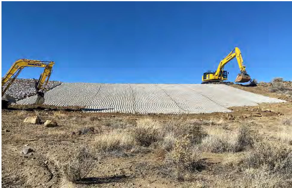
Photograph 44. View of the concrete ECB installation, looking northwest, upslope.
