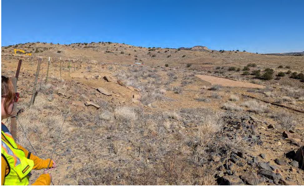
Photograph 18. View of biodegradable erosion control blanket and Eco Log, as installed at VS-5 (11-05-2024).
