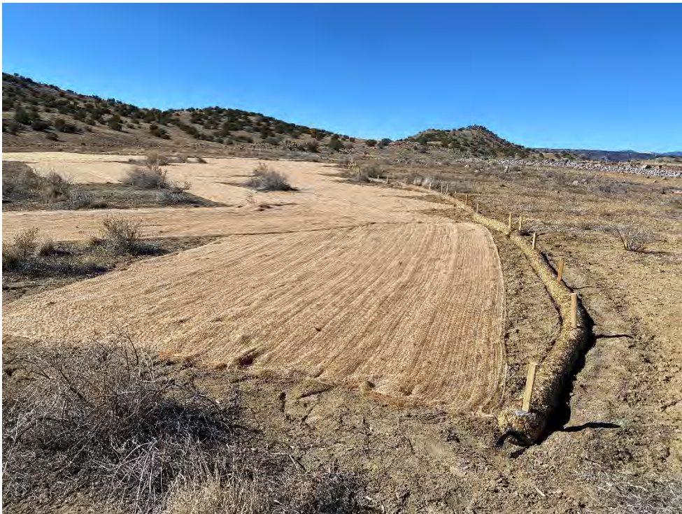
Photograph 65. View looking west from the area reseeded in the reclaimed Borrow Area. The area was roughened, reseeded, then covered with the biodegradable matting. Eco Log fiber rolls were placed on the downslope edge of the matting. Established woody shrubs were left in place.
