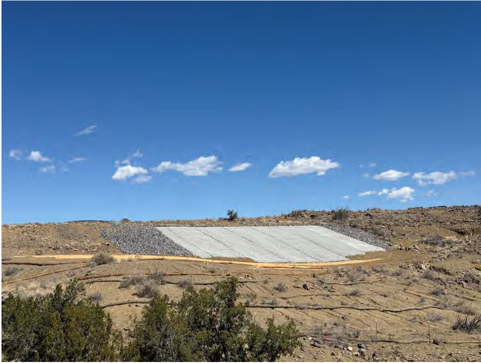
Photograph 82. Northwestern view, upslope, of the regraded, armored slope located at the transition from the reclaimed former borrow area to the reclaimed VS-10 (April 2025).
