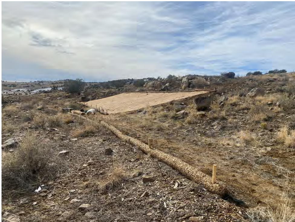
Photograph 22. Installation of biodegradable erosion control matting, below the hardscaping armor at Reclaimed VS-12 area.
