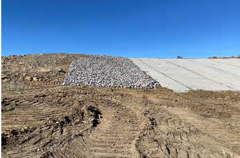
Photograph 45. Regrading was accomplished utilizing existing on-Site material present on the western edge of the slope. Due to the movement of this material, additional rock was installed to armor the exposed slope following reseeding methods.
