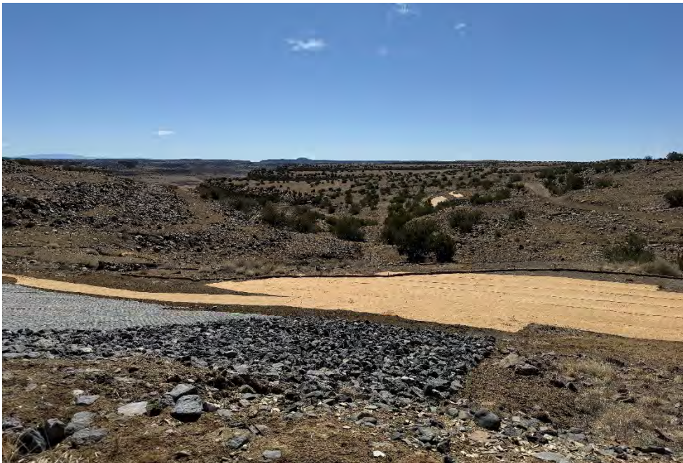
Photograph 77. Southeastern view, downslope, of the regraded, armored slope located at the transition from the reclaimed former borrow area to the reclaimed VS-10 (April 2025).
