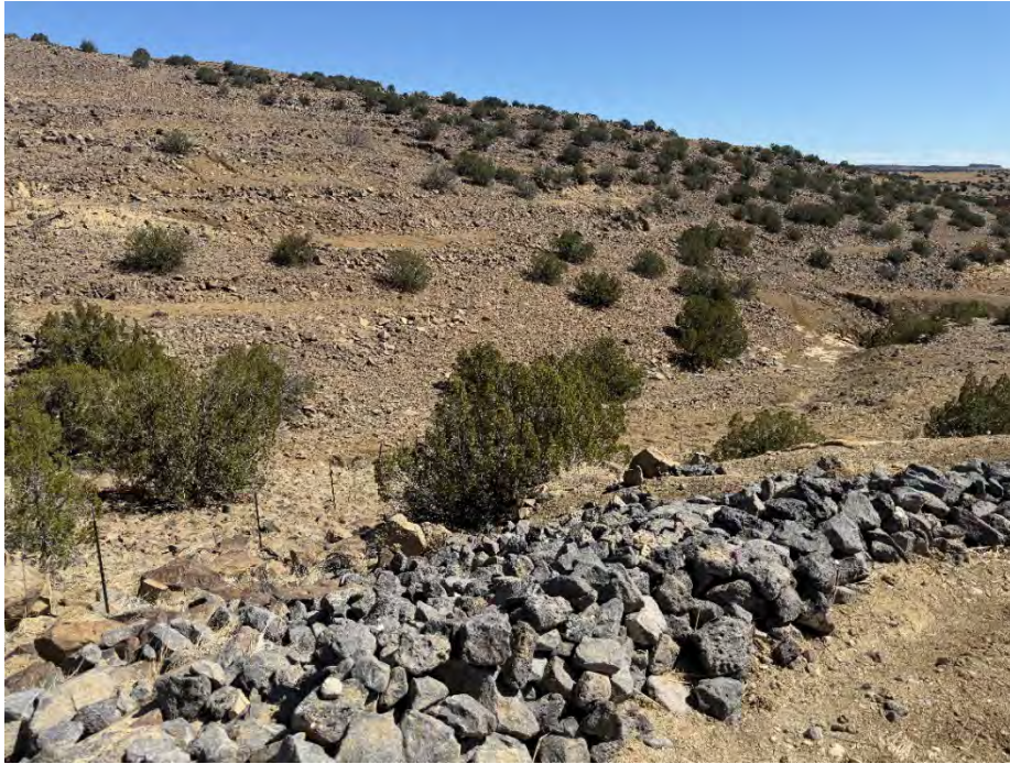
Photograph 80. View looking southeast from the upper slope at the reclaimed VS-12 area. The slope was armored with 6–12-inch rip rap (April 2025).
