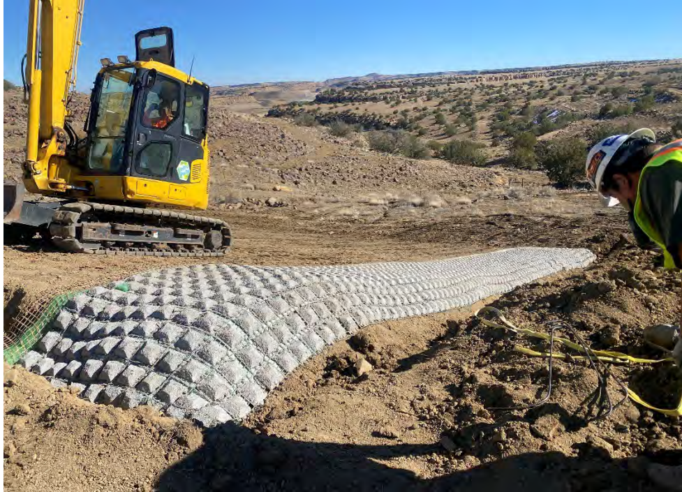
Photograph 39. The concrete ECB was anchored in a 12-inch trench, at a 45-degree angle at the outer edges of the slope.
