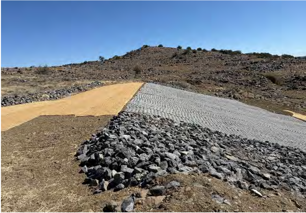
Photograph 76. East-northeastern view of sheet flow spreader, biodegradable matting, and regraded, armored slope located at the transition from the reclaimed former Borrow Area to the reclaimed VS-10 (April 2025).
