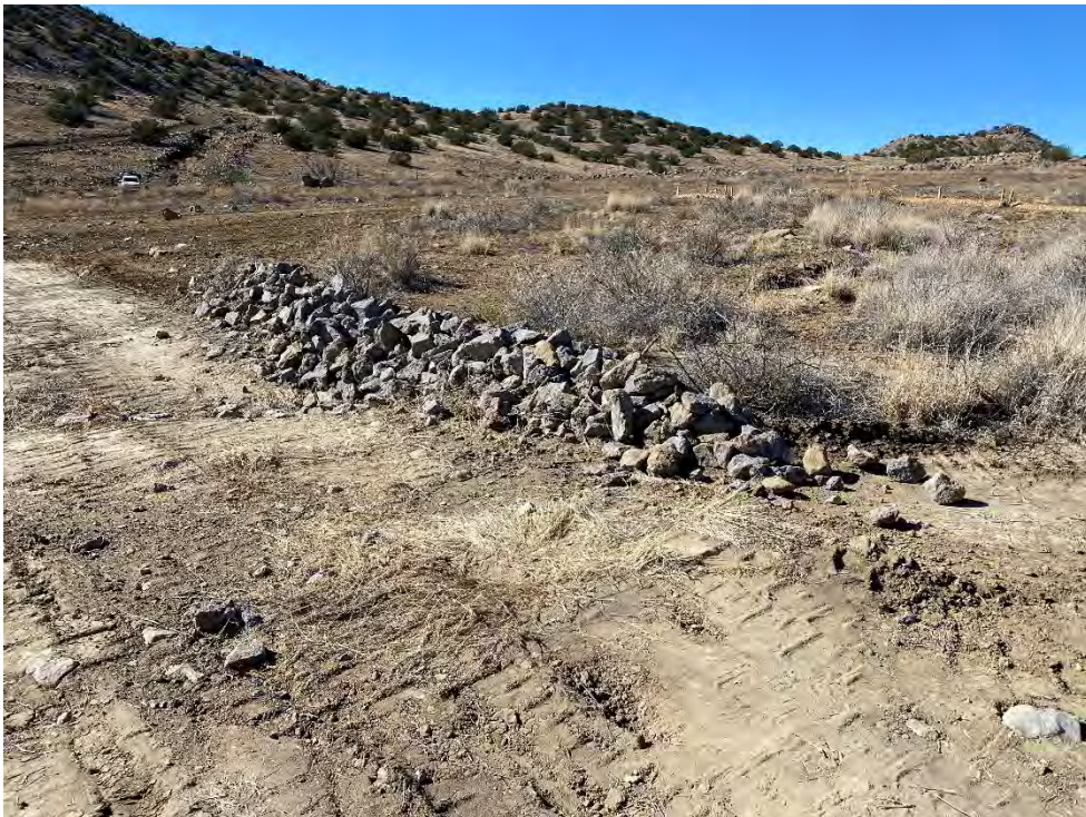
Photograph 67. Rock check dam maintenance utilizing on-Site available materials at reclaimed former Borrow Area.
