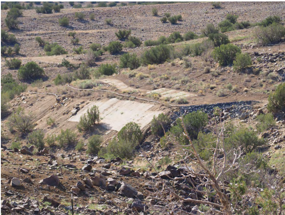
Photograph 97. View looking southeast from the within the VS-10 reclamation area to the reclaimed VS-12 area, including the armored slope, biodegradable matting, and Eco Log fiber rolls (September 2025).
