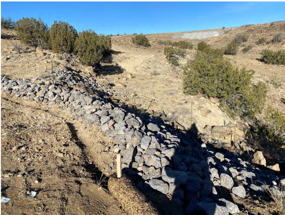
Photograph 59. View looking northwest from the regraded upper slope at the reclaimed VS-12 area. The channel was armored with 6–12-inch rip rap.
