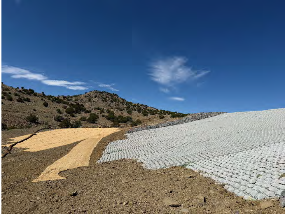
Photograph 78. West-northwestern view of the regraded, armored slope located at the transition from the reclaimed former borrow area to the reclaimed VS-10 (April 2025).
