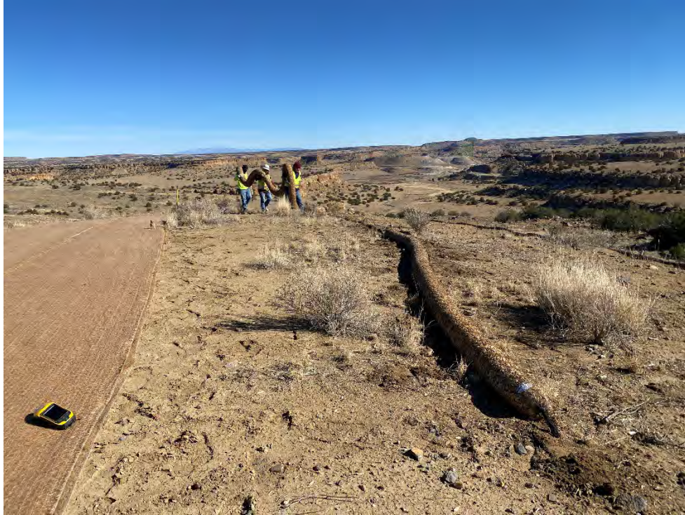
Photograph 70. Eco Log fiber rolls were keyed into the surface and installed along the contours of the slope.
