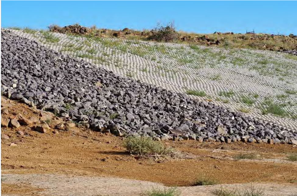
Photograph 88. Northeastern view, of the regraded, armored slope located at the transition from the reclaimed former borrow area to the reclaimed VS-10 (September 2025).
