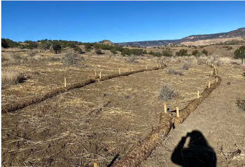
Photograph 50. Eco Log fiber rolls were placed along the contours of the slope at the Reclaimed VS-11 area. Seed was broadcast between the fiber rolls and covered with straw material.
