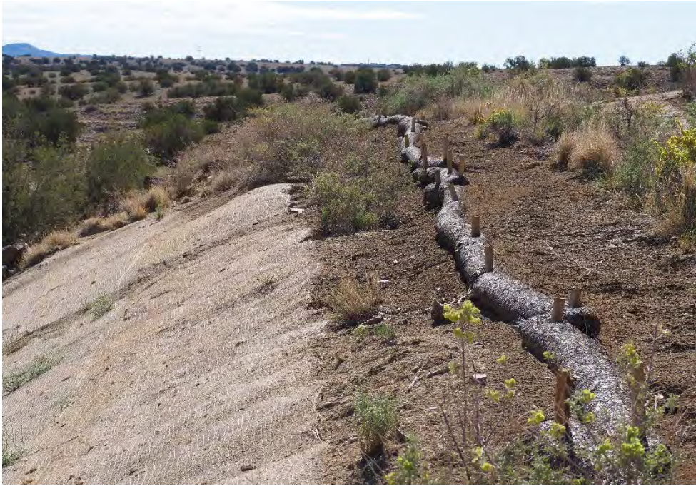
Photograph 96. View looking southeast from the reseeded slope at the reclaimed VS-12 area. The area was roughened, reseeded, then covered with the biodegradable matting (September 2025).
