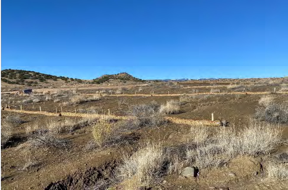
Photograph 25. Eco Log fiber rolls, installed on the eastern portion of the upper catchment area of the Reclaimed Borrow Area.
