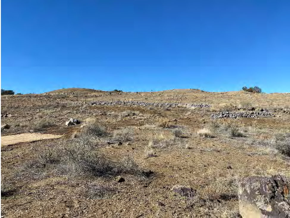
Photograph 27. View of bolstered rock check dams, installed and repaired at Reclaimed VS-6.
