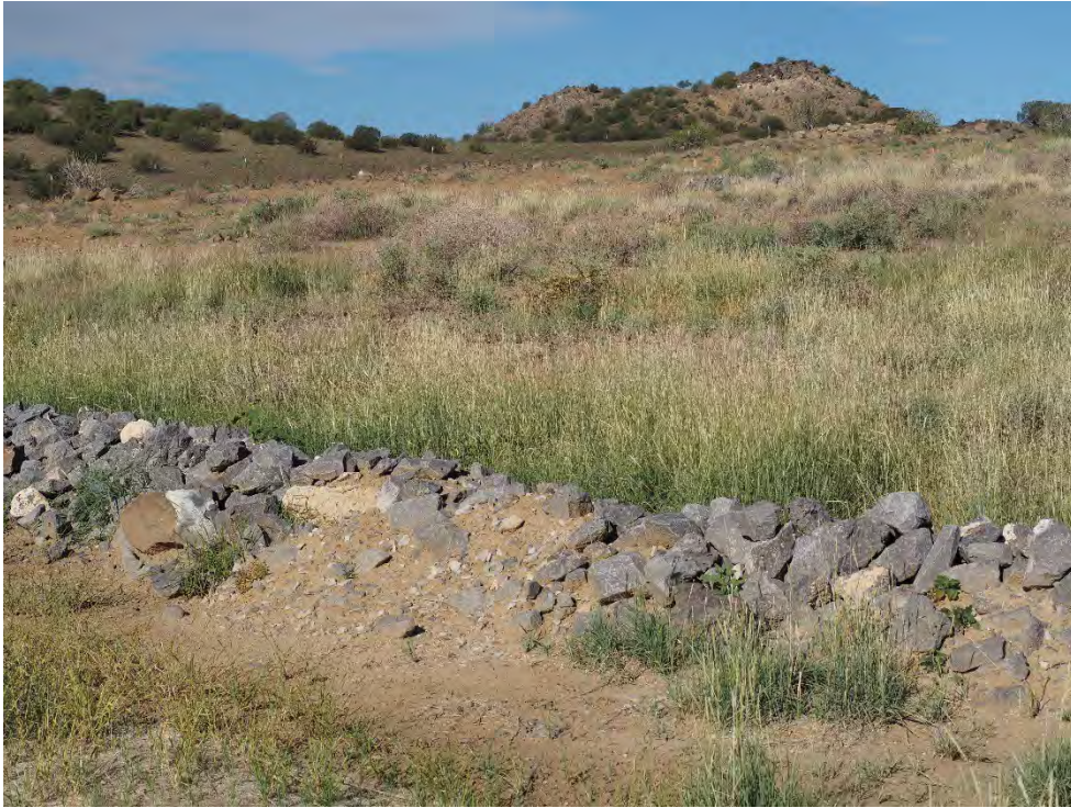
Photograph 94. View of the sheet flow collector media luna at the transition from the reclaimed Borrow Area and reclaimed VS-10 area with established vegetation upslope (September 2025).
