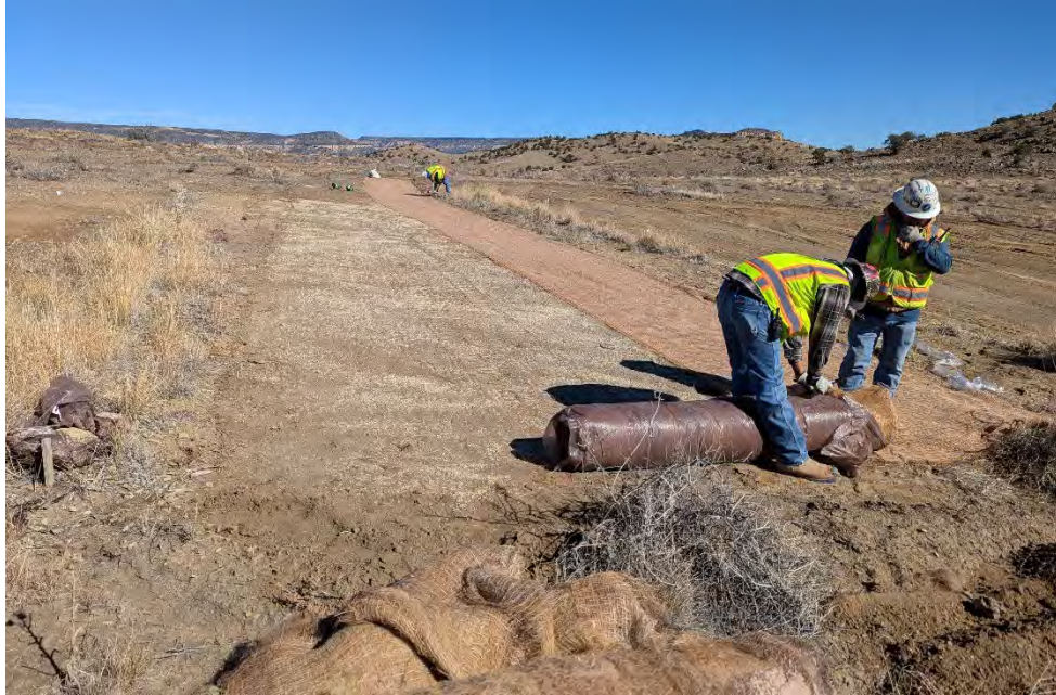
Photograph 16. View of biodegradable erosion control matting installation on prepared subgrade/surface, following broadcast seed application. Established vegetation was left in place (11-05-2024).
