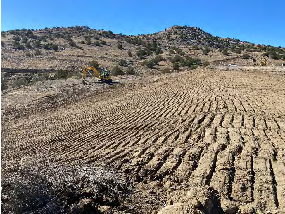
Photograph 37. View of the regraded and prepared slope at the Reclaimed VS-10 Area, looking to the southwest.
