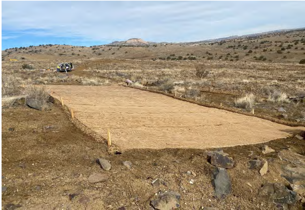
Photograph 23. View looking NNE at a portion of biodegradable erosion control matting, as installed, with the Eco Log wattles along the edges. The matting and wattles were placed parallel to the contour of existing topography onto a prepped surface (rocks removed).
