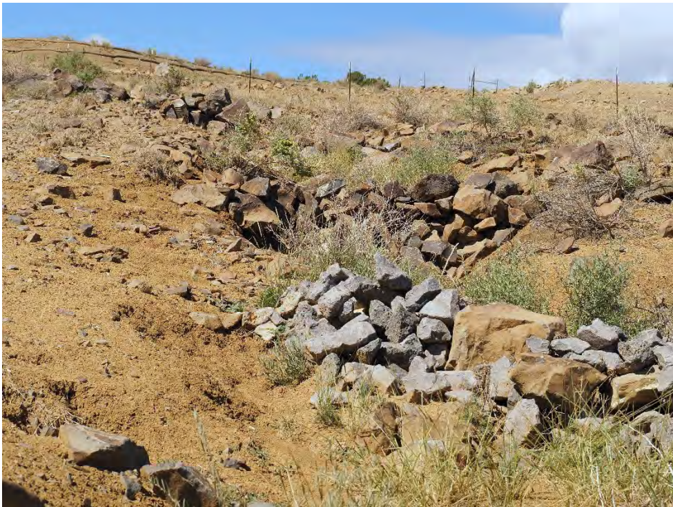
Photograph 99. View of rock check dam bolstering installed at the reclaimed VS-6 area (September 2025).
