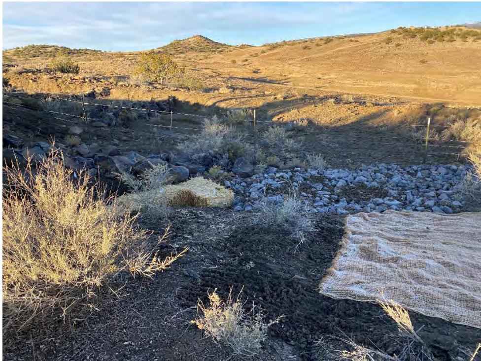
Photograph 34. View of Reclaimed VS-4 Area following seeding and biodegradable mat installation.
