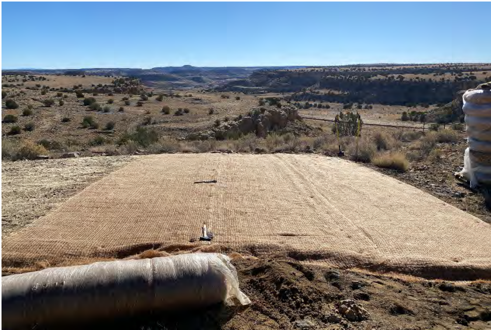
Photograph 12. View of the BioNet® C125BN™ erosion control matting. The matting was placed onto the prepped surface after seeding was completed.
