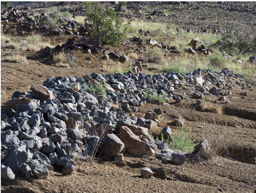
Photograph 85. View of the eastern portion of the sheet flow collector media luna. Some vegetation and rilling (September 2025).
