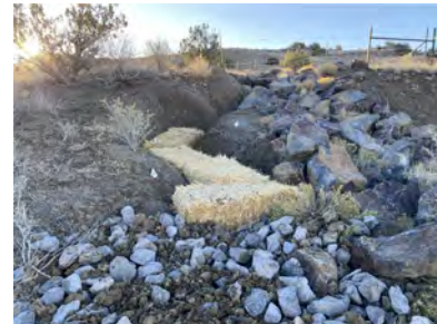
PHOTOGRAPH DEPICTING STRAW BALE INSTALLATION (TYPICAL).
