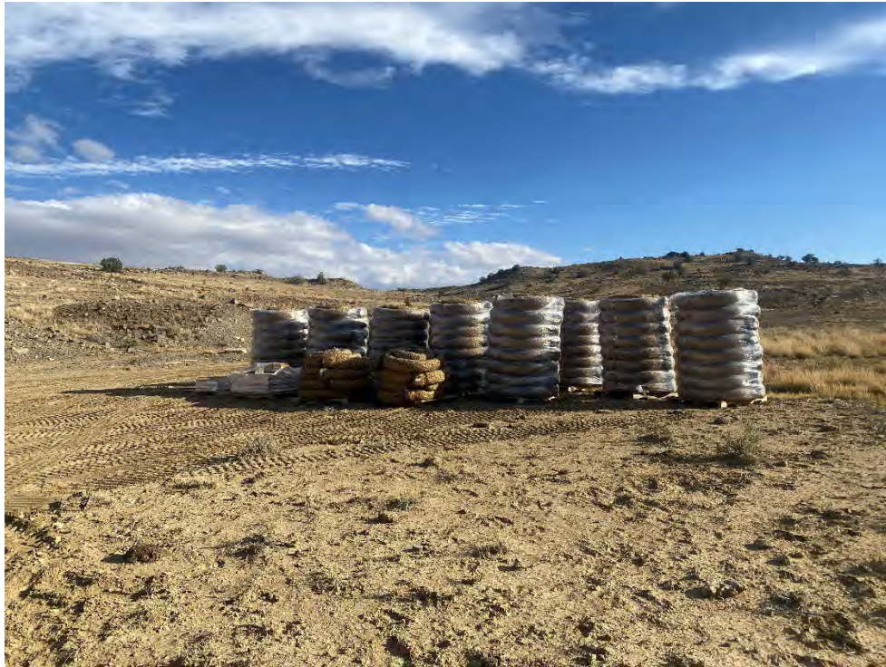
Photograph 5. The Eco Log wood chip compost wattles and socks in the staging area.
