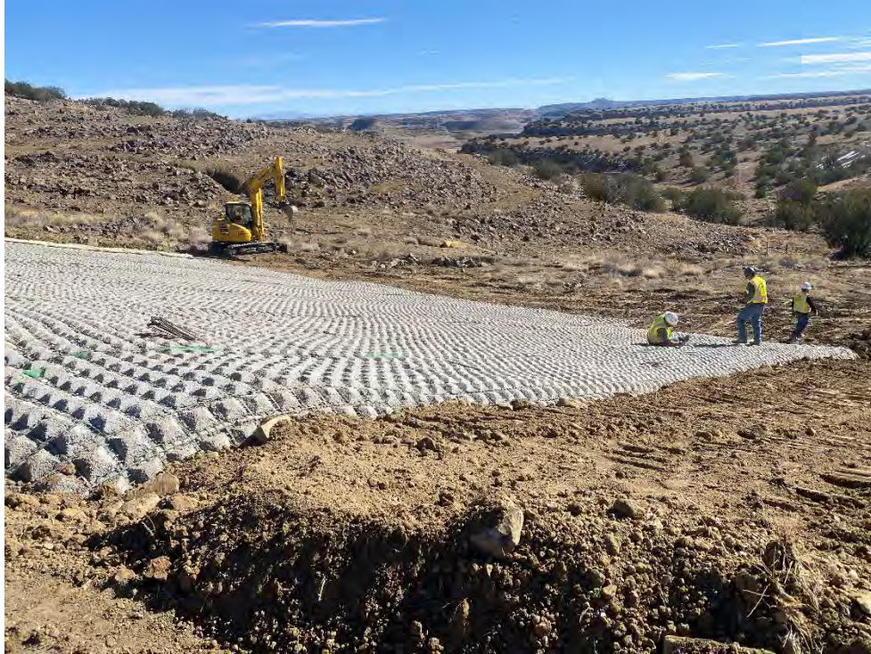
Photograph 43. Panels were installed using U-anchors at 2-ft increments and overlapped 12–18 inches.
