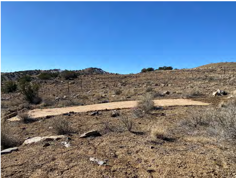
Photograph 28. View of installed biodegradable seed mat at Reclaimed VS-6.
