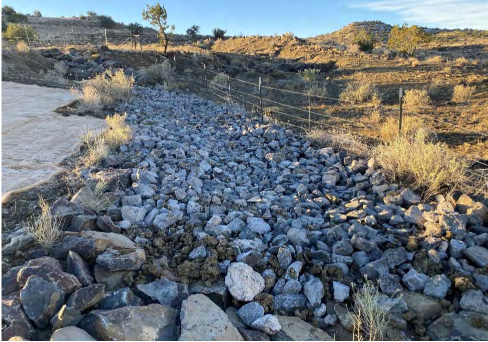
Photograph 31. 6–12-inch rip rap rock was installed upgradient of the existing rock armor at the Reclaimed VS-12 area.
