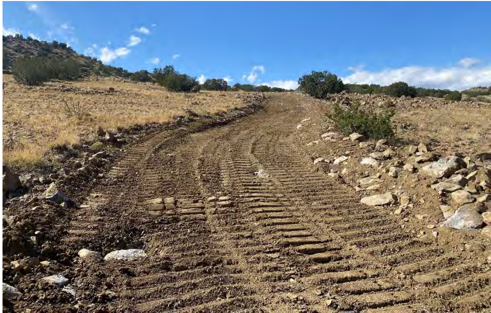
Photograph 8. The access road to Reclaimed VS-11 area was graded to facilitate staging supplies for BMP installation.
