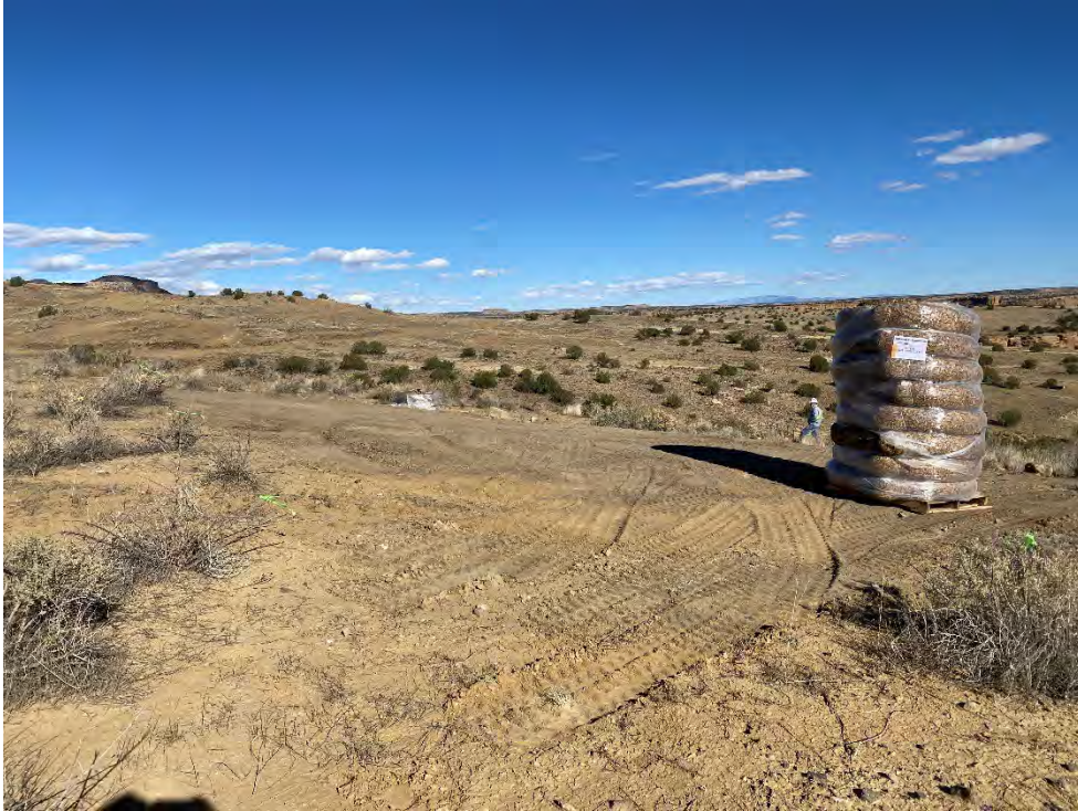
Photograph 11. View of the top area of Reclaimed VS-11 area as Eco Logs are staged and after the skid steer equipment prepped the surface.
