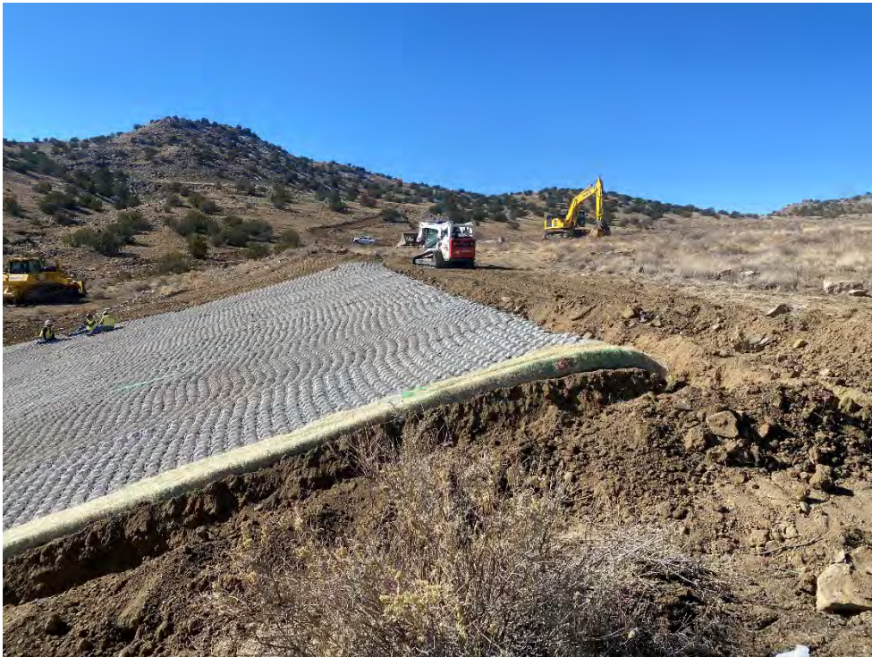
Photograph 42. The concrete ECB was anchored in an 18-inch top trench at a 90-degree angle and in two 12-inch side trenches at 45-degree angles at the outer edges of the slope.
