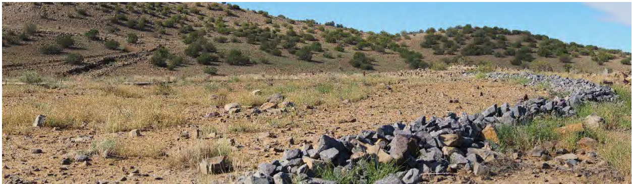
Photograph 95. View of the sheet flow collector media luna at the transition from the reclaimed Borrow Area and reclaimed VS-10 area with established vegetation upslope (September 2025).
