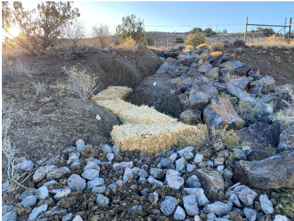
Photograph 32. Strawbales were installed by driving two #4 rebar stakes into the center of each bale. View of Reclaimed VS-4 Area.
