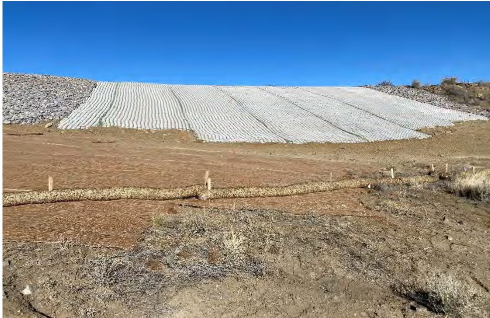
Photograph 60. View looking upslope from the area reseeded below the armored slope at the reclaimed VS-10 area. The area was roughened, reseeded, then covered with the biodegradable matting. Eco Log fiber rolls were placed on the downslope edge of the matting.
