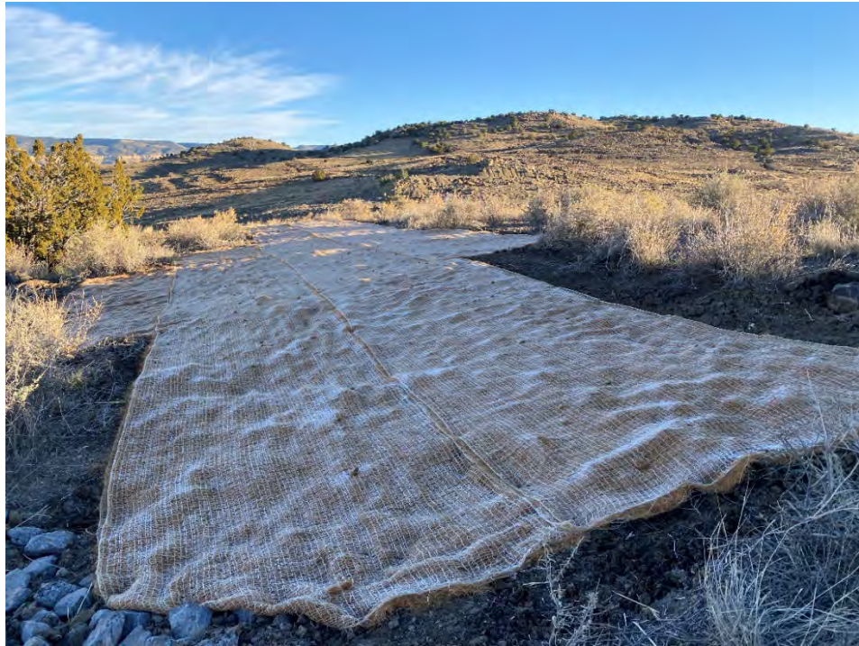
Photograph 33. View of Reclaimed VS-4 Area following seeding and biodegradable mat installation.
