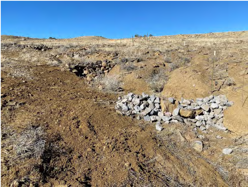
Photograph 26. View of bolstered rock check dams, installed and repaired at Reclaimed VS-6.
