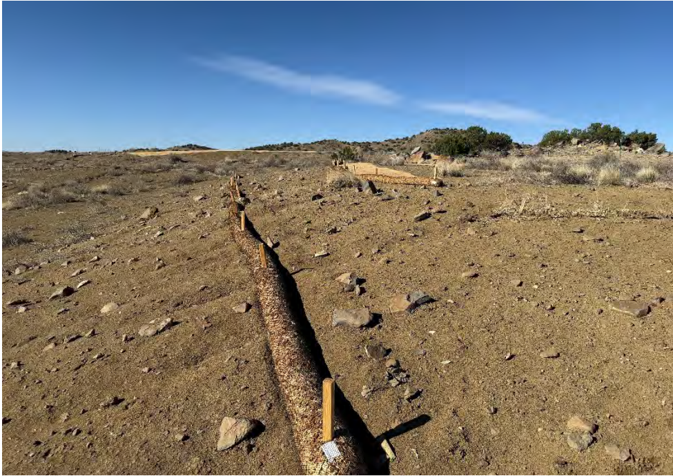
Photograph 72. View of slope located at reclaimed VS-5 (foreground) and VS-6 (background) with Eco Log and biodegradable matting (April 2025).
