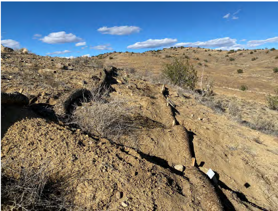
Photograph 10. View of the eastern slope at Reclaimed VS-11 area with a section of Eco Log installed. The wattles were keyed into the soil and placed along the contour, down slope from existing wattles.
