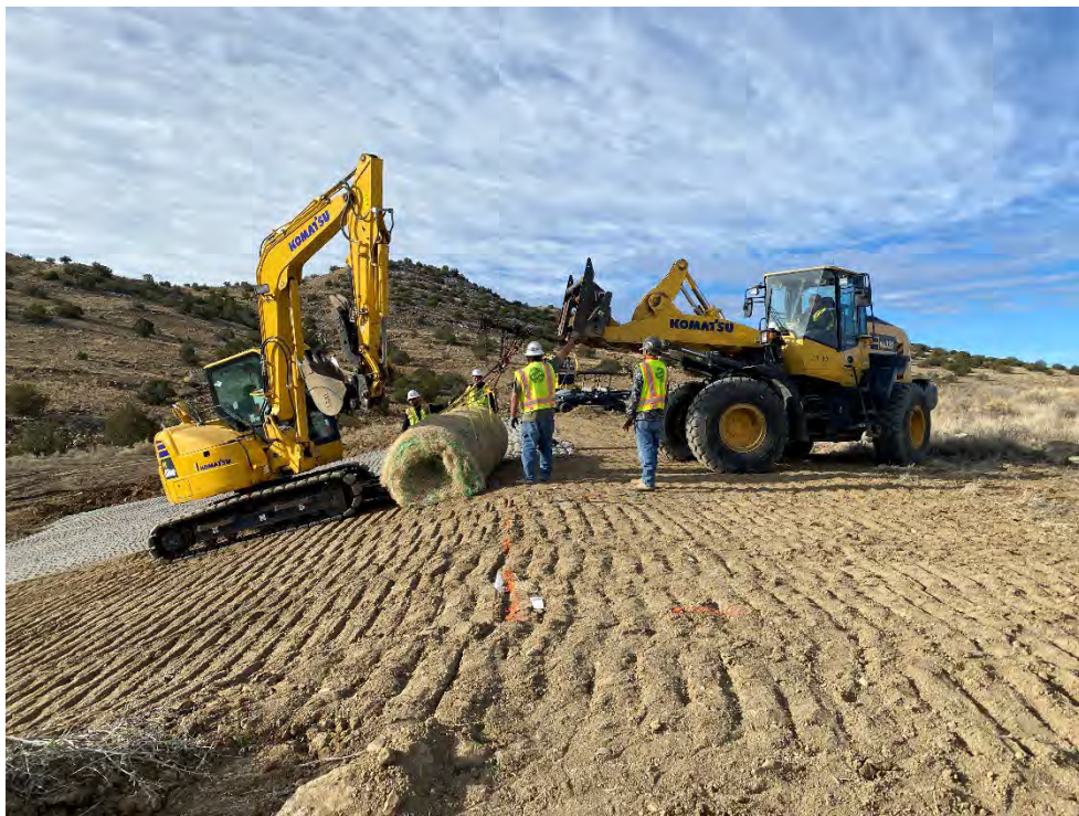
Photograph 40. Installation of the concrete ECB.
