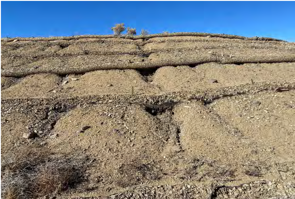
Photograph 53. New Eco Log fiber rolls were installed along the contours of the former and reclaimed Stockpile Area.
