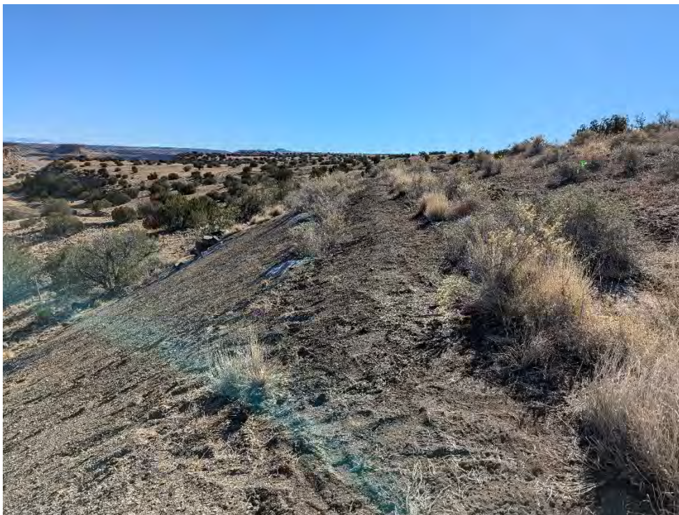
Photograph 19. View of slope requiring seeding and erosion protection at the reclaimed VS-12 area (11-05-2024).
