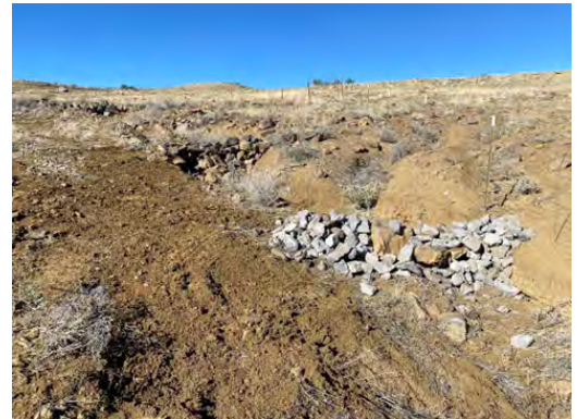
PHOTOGRAPH DEPICTING TYPICAL ROCK CHECK DAM REPAIR WORK.
