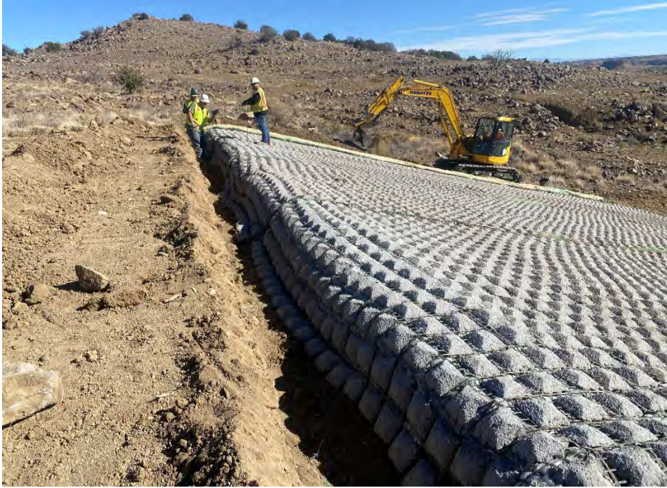
Photograph 41. The concrete ECB was anchored in an 18-inch x 18-inch trench at the crest of the slope. Eight sectioned panels were installed, west-east. The easternmost panel was 8-ft wide, and the remaining panels were 15.5-ft wide.
