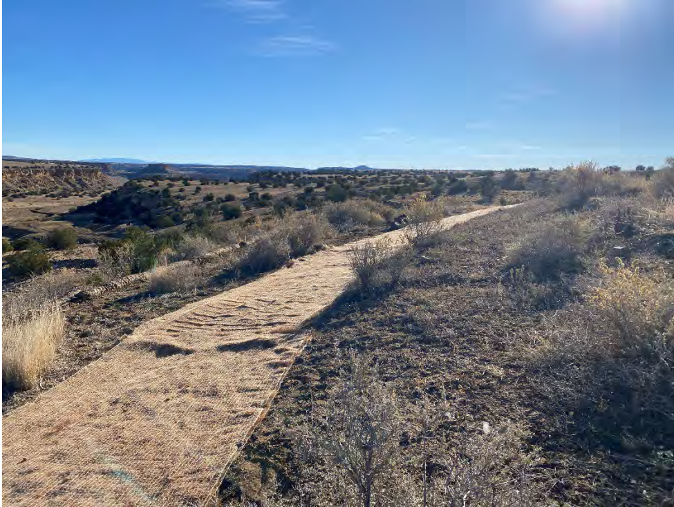
Photograph 56. View looking southeast from the reseeded slope at the reclaimed VS-12 area. The area was roughened, reseeded, then covered with the biodegradable matting.
