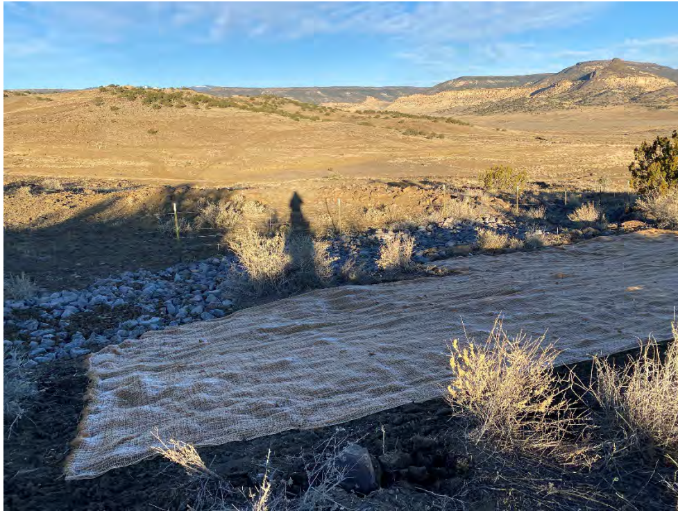
Photograph 35. View of Reclaimed VS-4 Area following seeding and biodegradable mat installation.
