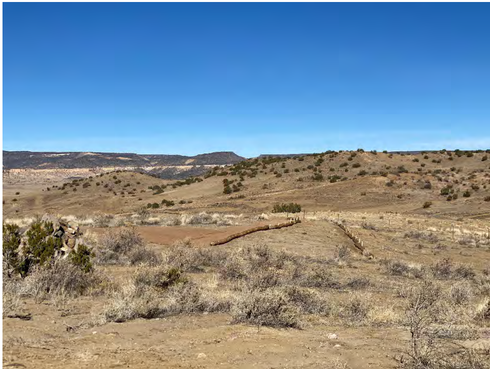
Photograph 71. Eco Log fiber rolls were keyed into the surface and installed along the contours of the slope.
