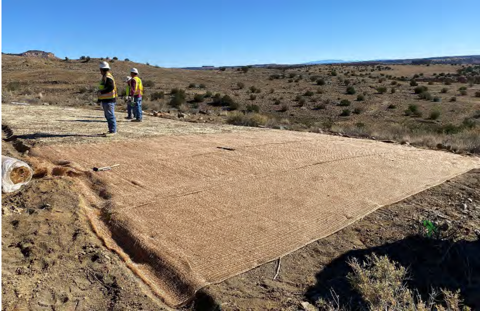
Photograph 13. View of the BioNet® C125BN™ erosion control matting. The matting was placed onto the prepped surface after seeding was completed.
