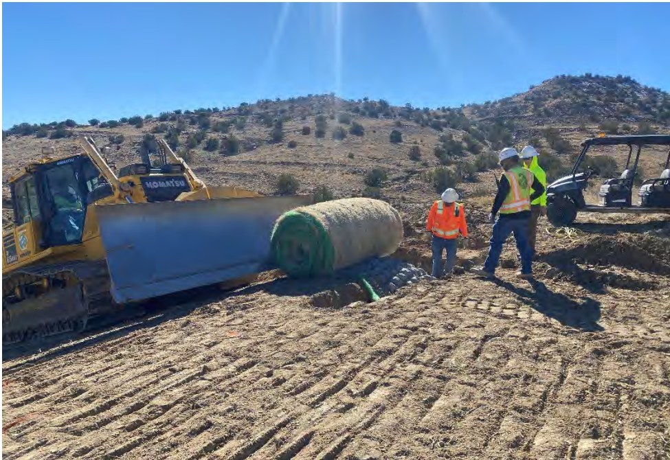
Photograph 38. The concrete erosion control blanket (ECB) was anchored in an 18-inch x 18-inch trench at the crest of the slope.
