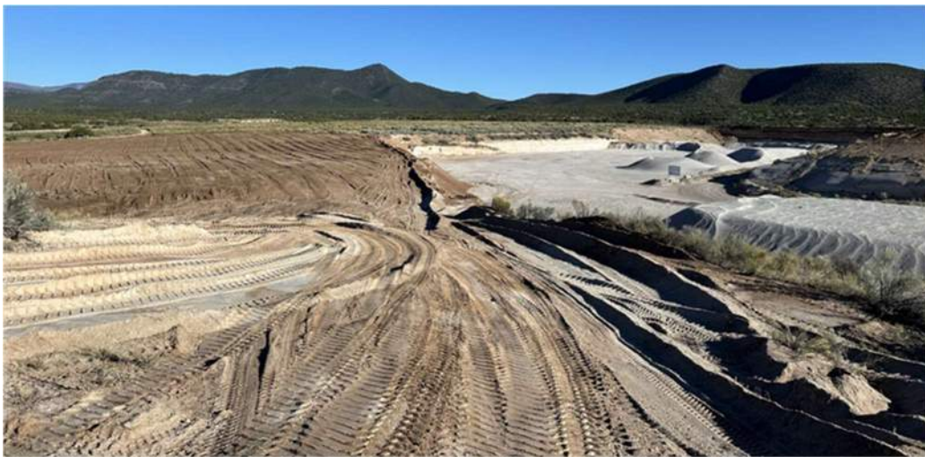
Figure 3. Photo of grading area, seeded after final stabilization
