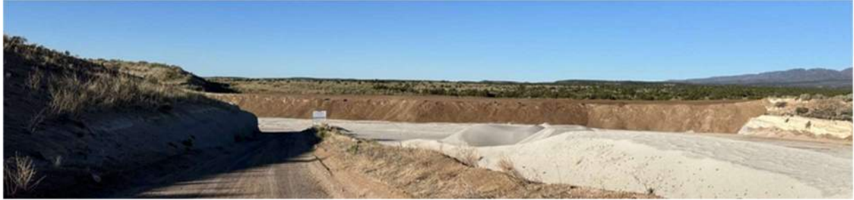
Figure 4. Photo of grading area, seeded after final stabilization
