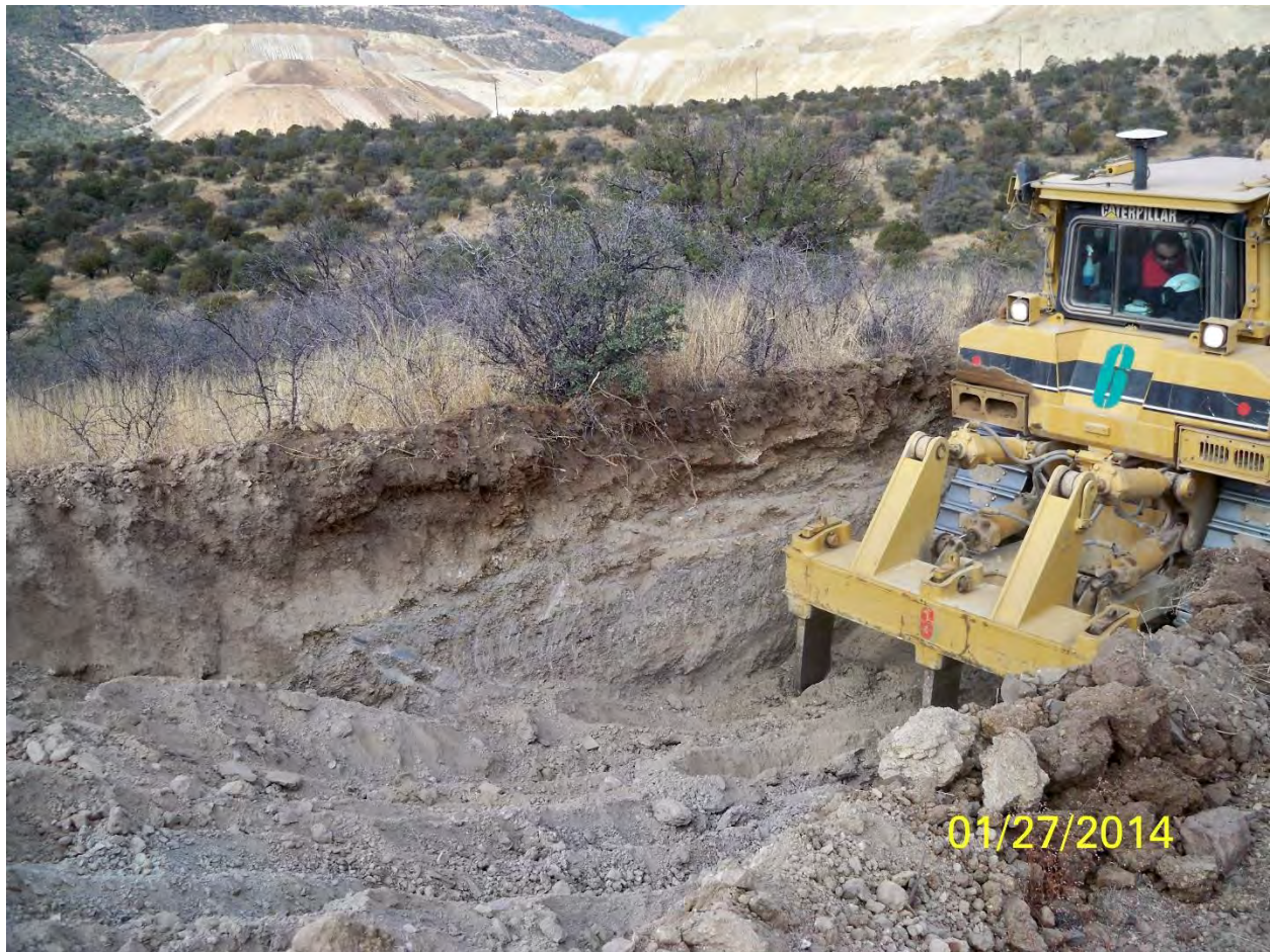
Figure 5. Caterpillar D6 ripping through the RPF
