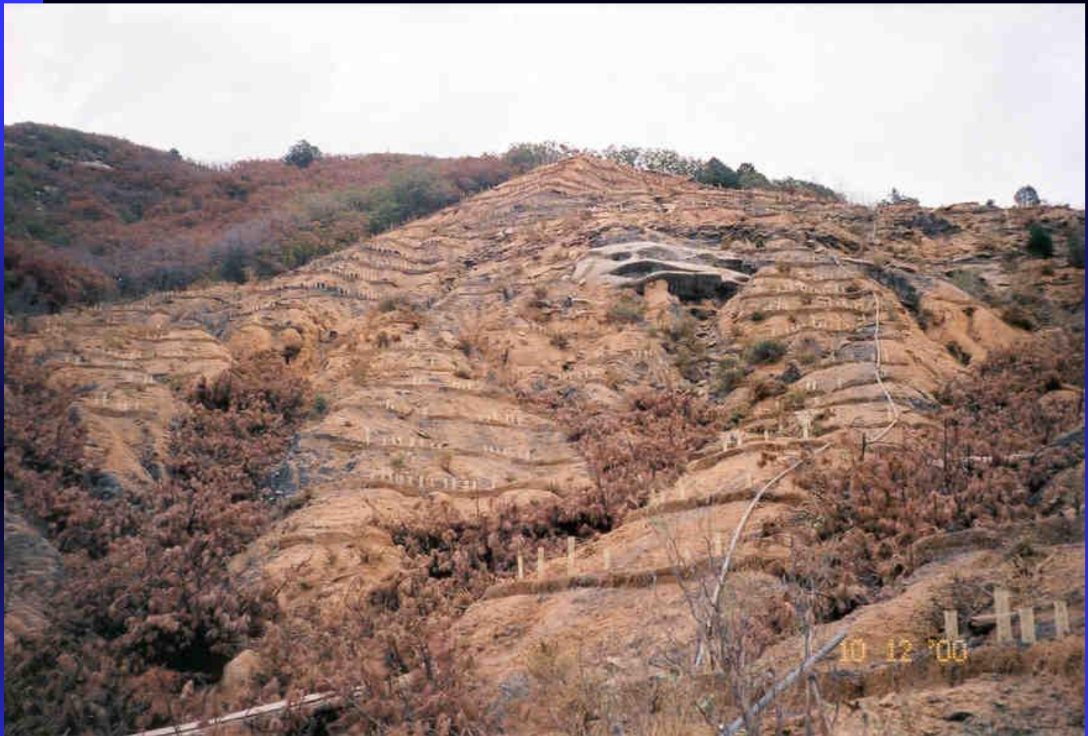
Hydroseeded slopes at Gob Pile A2N
