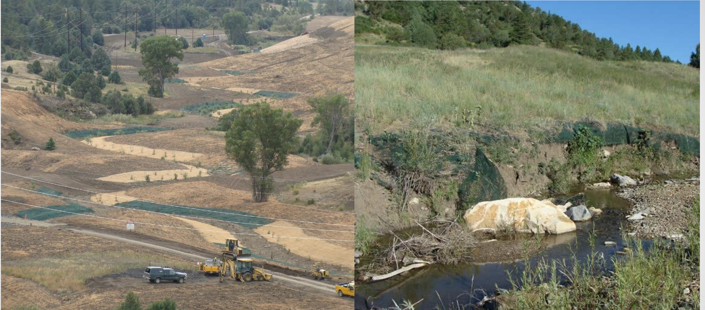
Figure 1. Original completed project (left) and aftermath of 2012 storms (right). Banks of the channel were potentially eroding into buried gob material.
