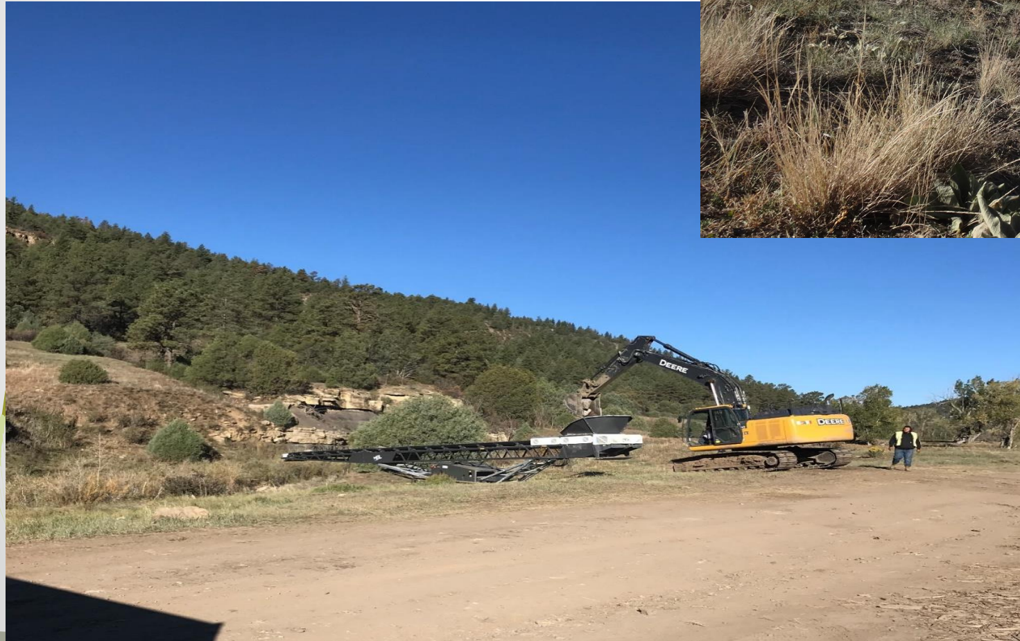
Figure 5. Conveyor belt being used to drop boulders into place in the stream channel across an archaeological avoidance area (left) and equipment work in the channel (above).
