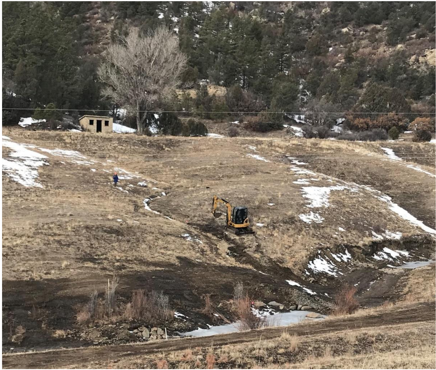
Figure 8. Working on upland erosion control structure in steep, frozen conditions.
