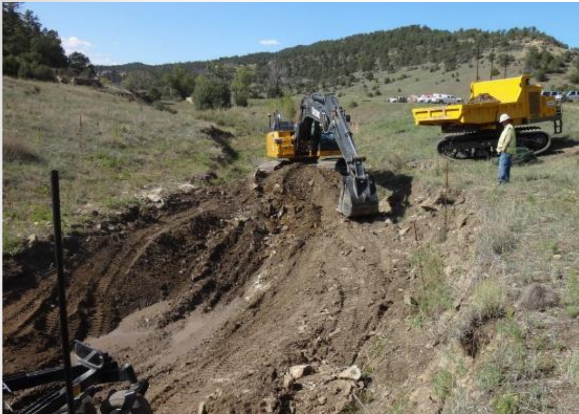
Figure 6. Shaping Pools within Channel for Installation of Rock Structures (Cross Vanes)
