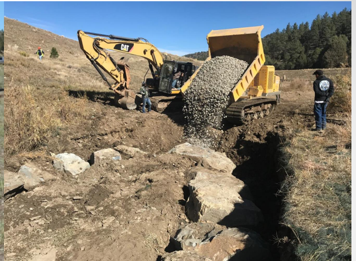
Figure 6. Shaping Pools within Channel for Installation of Rock Structures (Cross Vanes)
