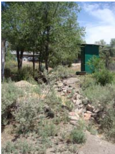
A cobble-lined swale emptying onto Cave Road
