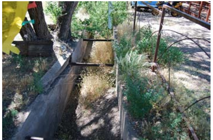
Existing concrete flume. Note sedimentation and conditions.
