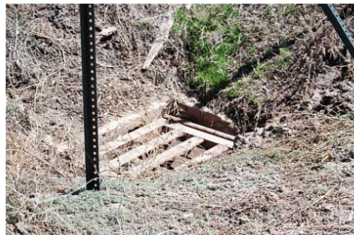
Existing drop inlet on the east side of NM 14.
