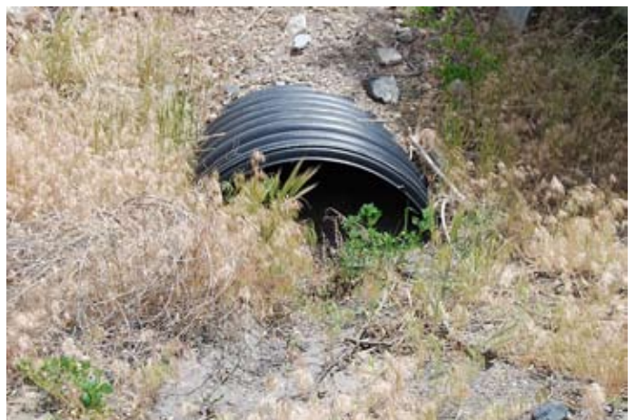
Culvert in arroyo impaired by sediment
