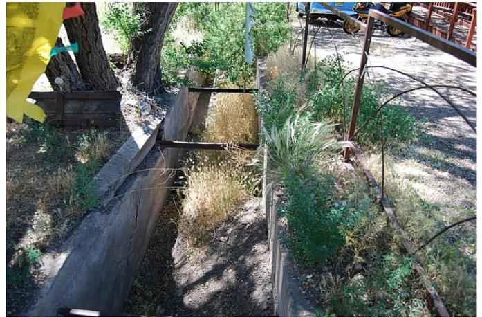
*Existing concrete flume. Note sedimentation and conditions.*
