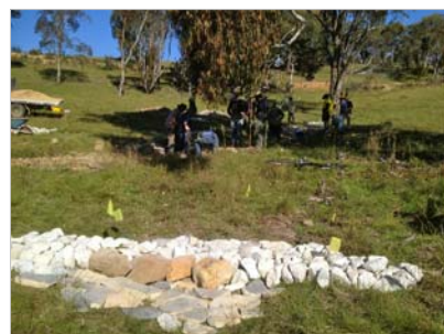
ROCK LINED CONVEYANCE CHANNEL
