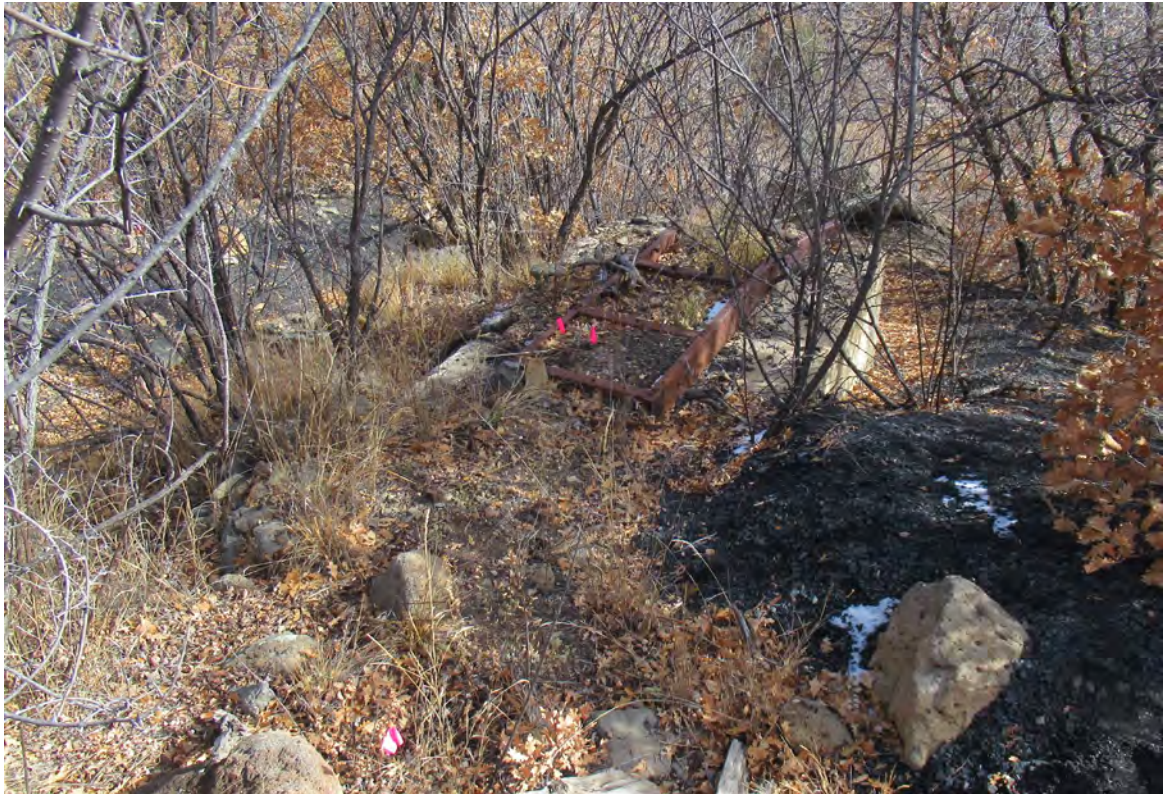
Photograph 61. LA 119818 Feature 36 (Concrete Platform) Overview
