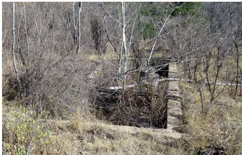
Photograph 48. LA 119818 Feature 13 (Concrete Foundation)
