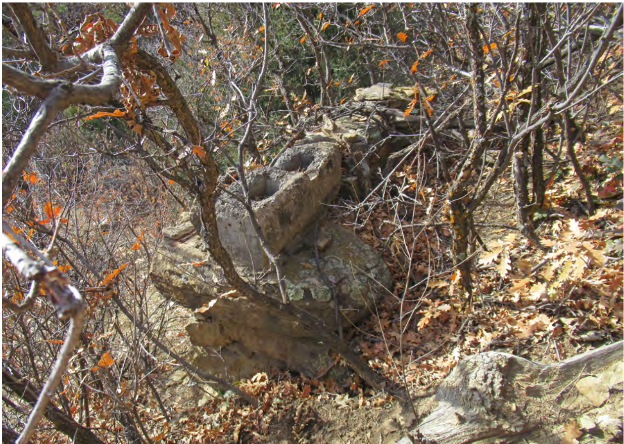
Photograph 126. LA 202932 Feature 1 (Masonry Wall)
