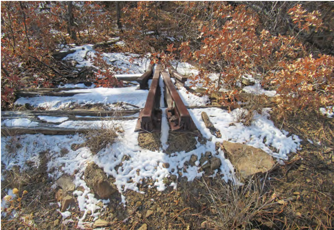
Photograph 69. Segment of Intact Railroad Ties and Narrow-gauge Rail along the Tramway
