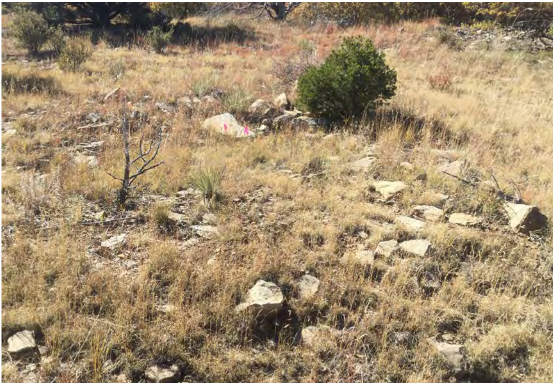
Photograph 85. LA 120611 Feature 8 (Masonry Foundation)
