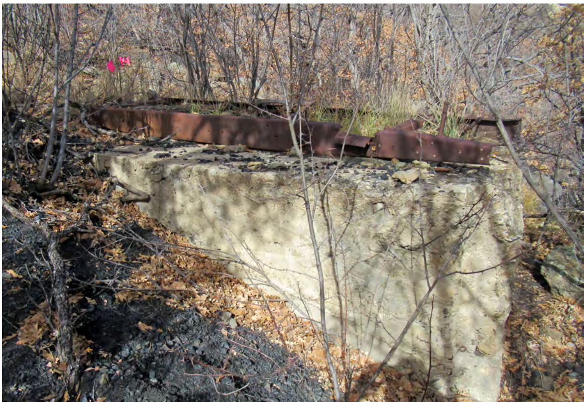
Photograph 62. LA 119818 Feature 36 (Concrete Platform) Profile View
