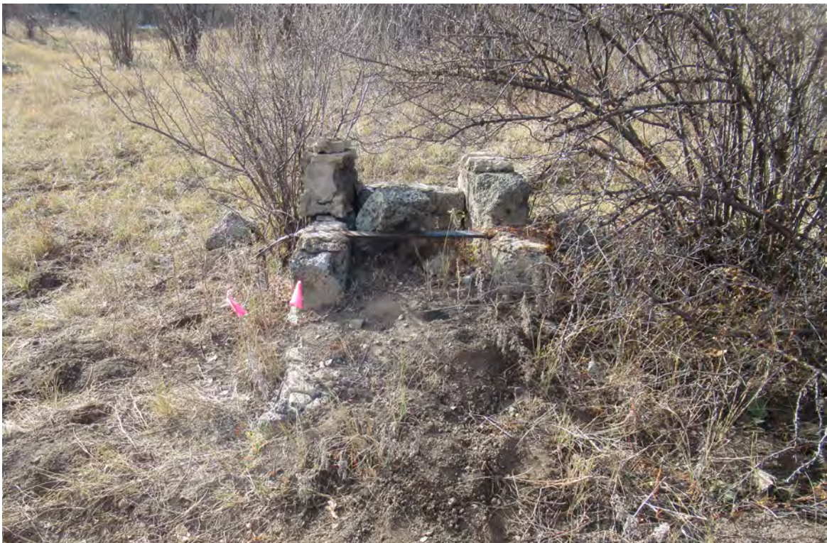
Photograph 54. LA 119818 Feature 19 (Concrete Platform)
