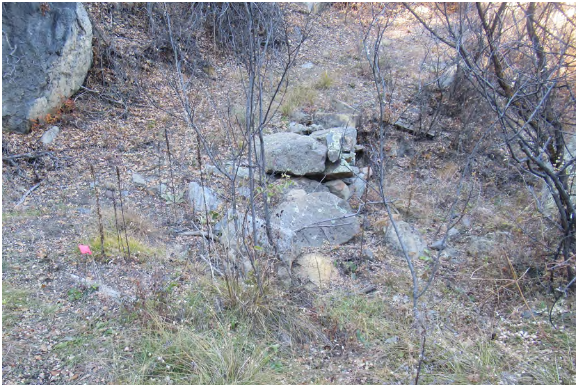
Photograph 141. LA 202933 Feature 9 (Road-Related Retaining Wall)
