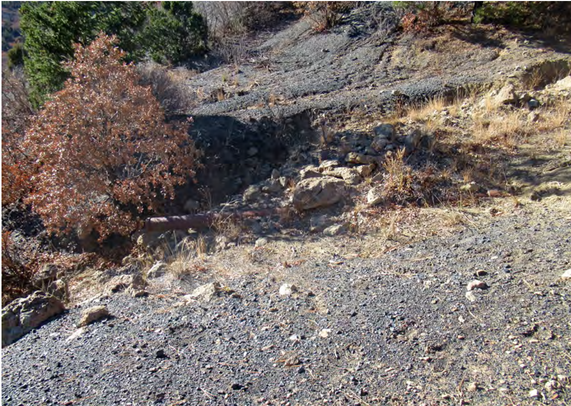
Photograph 22. LA 119817 Feature 6 (Road-Related Drainage Pipe)
