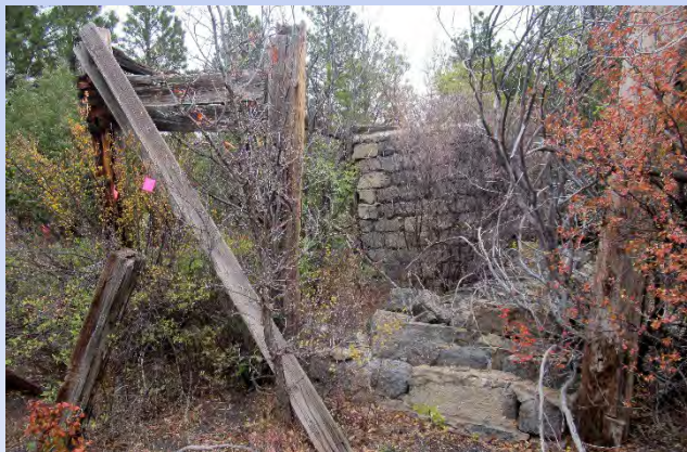
Tippie Structure Remains
