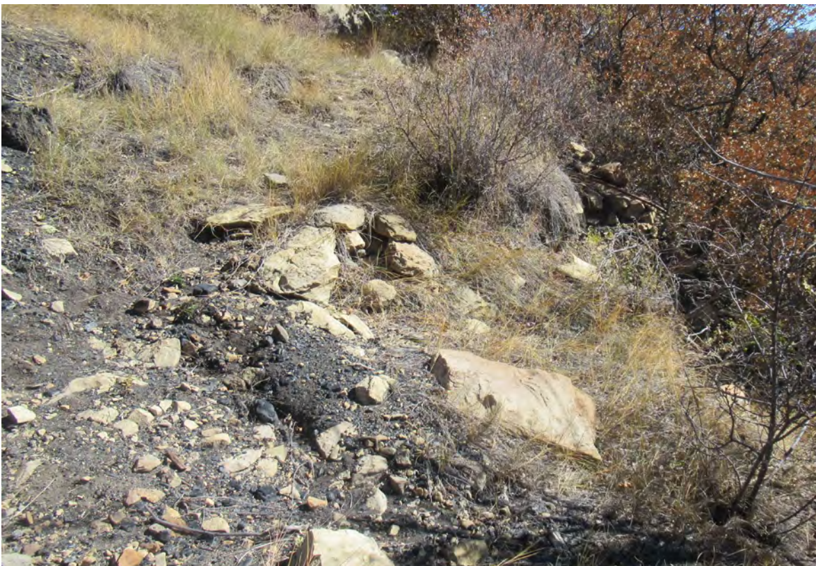
Photograph 10. LA 57200 Feature 4 (Retaining Wall)
