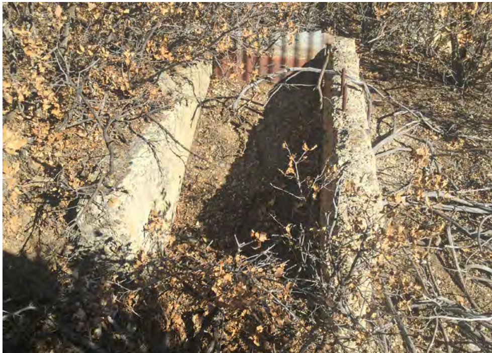
Photograph 19. LA 119817 Feature 4 (Fan Mount Structure)
