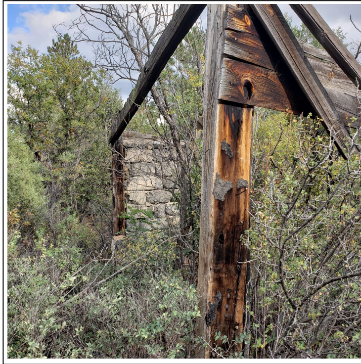
3. Mining structure with overgrown vegetation, south end of the northern parcel
