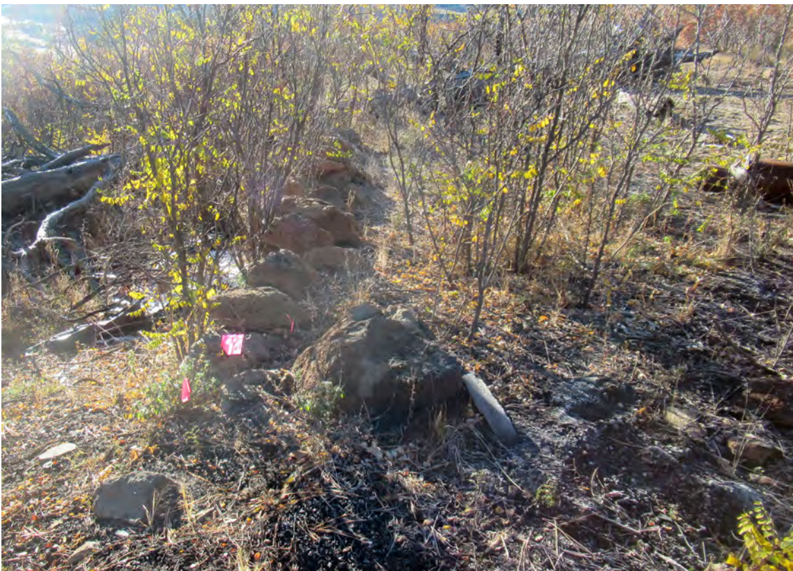
Photograph 25. LA 119818 Feature 3 (House) Today Showing Intact Foundation Wall
