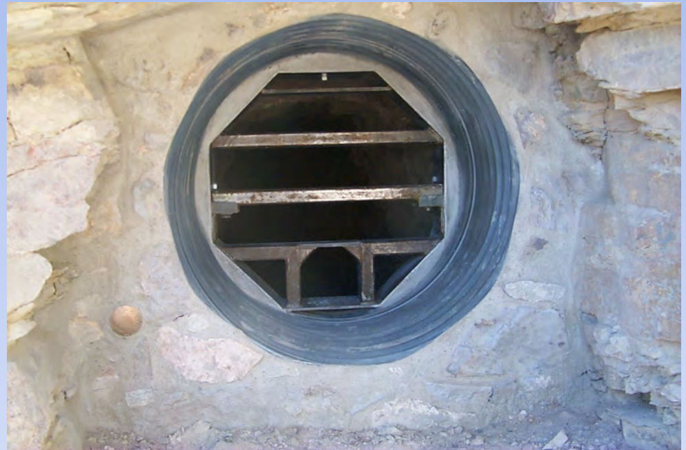
Culvert with bat and wildlife-friendly gate
