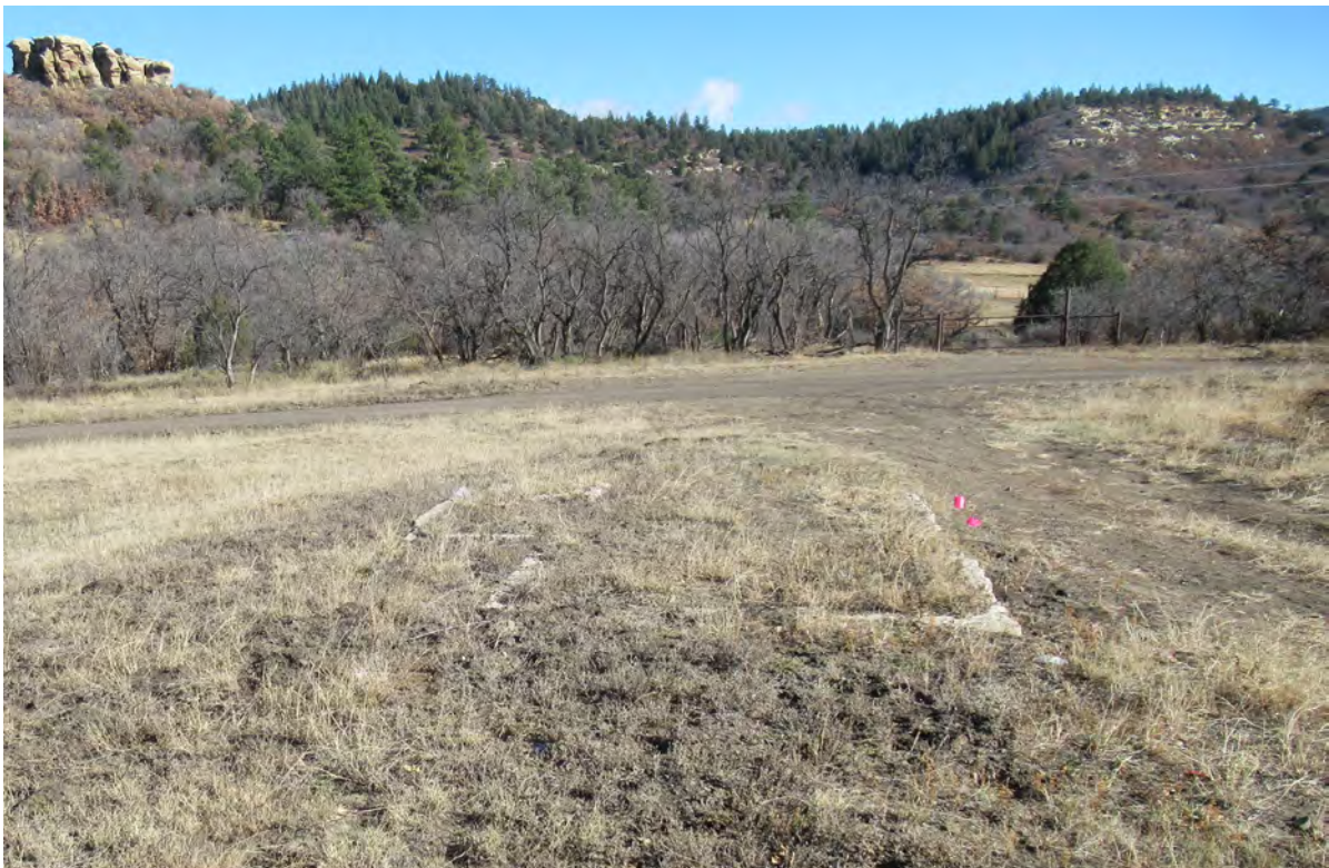
Photograph 52. LA 119818 Feature 17 (Concrete Foundation)
