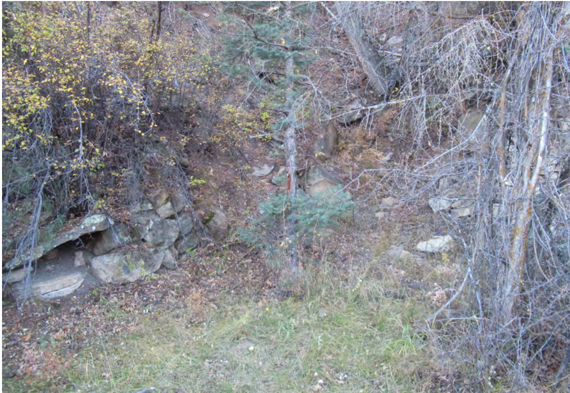
Photograph 133. LA 202933 Feature 11 (Adit and Supporting Walls)
