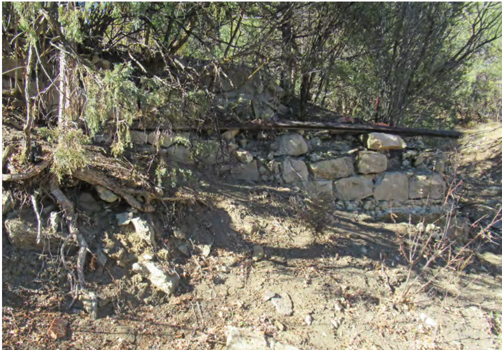
Photograph 143. LA 202933 Feature 3 (Masonry Wall)
