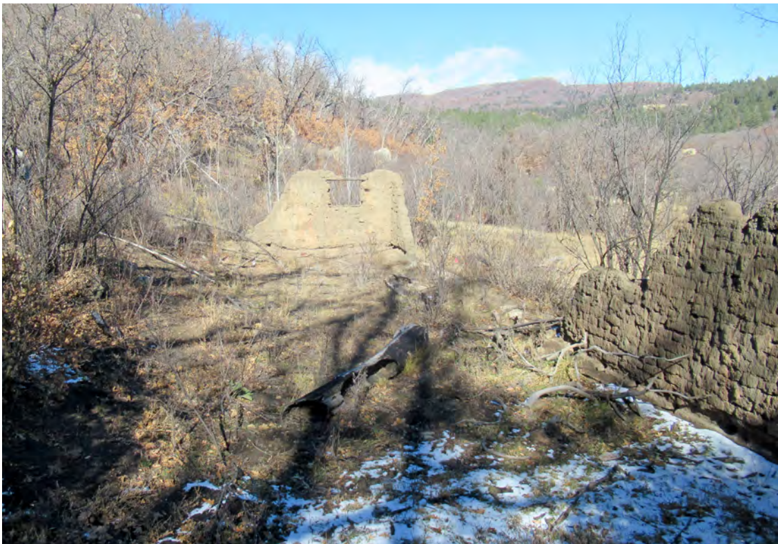
Photograph 43. LA 119818 Feature 12 (Two-Room Adobe Structure)
