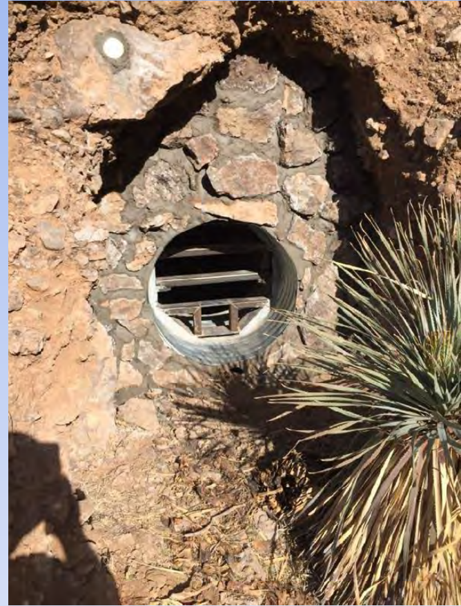
Rock bulk-headed culvert with bat-friendly gate. Cemented rocks assist with blending into landscape
