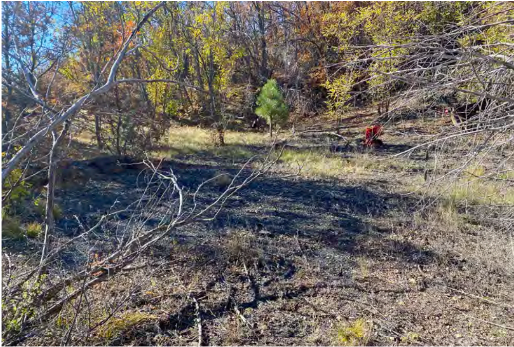
Photograph 102. AC 1 with Feature 1 (Open Cut in Background); Ramp (Feature 2) Not Visible
