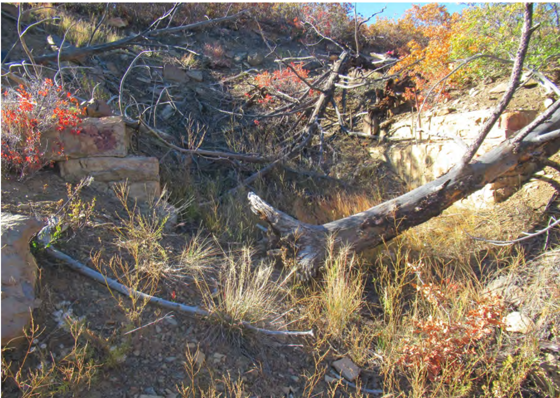
Photograph 79. LA 120611 Feature 13 (Closed Adit)
