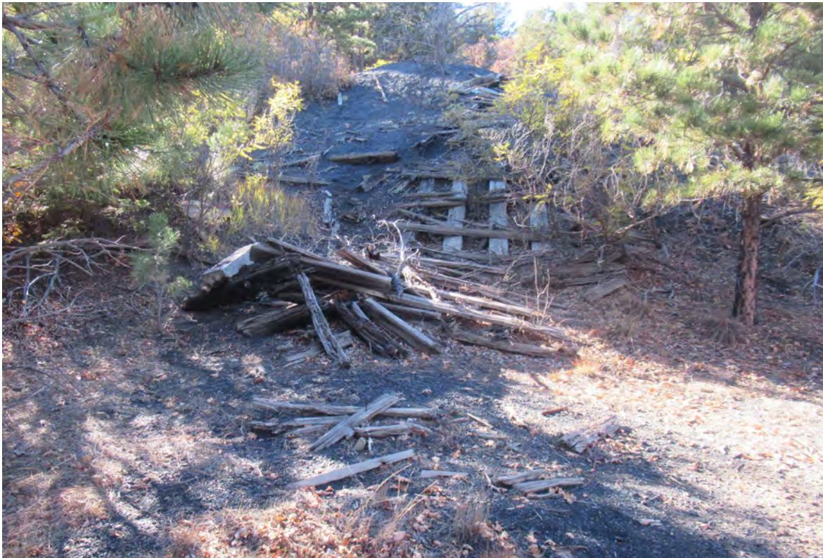
Photograph 110. LA 202929 Feature 4 (Timber Loadout Ramp/Structure) and Feature 8 (Waste Rock Pile)
