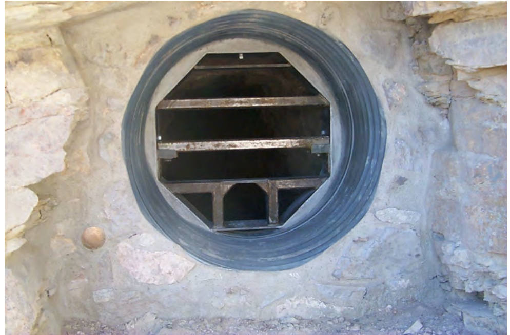
Culvert with bat and wildlife-friendly gate
