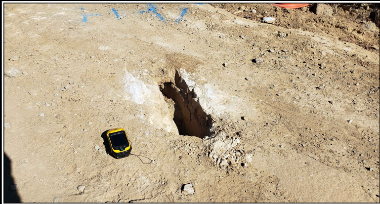
A COUNTY ROAD A-25 SUBSIDENCE FEATURE-1-1 SCALE: NONE
