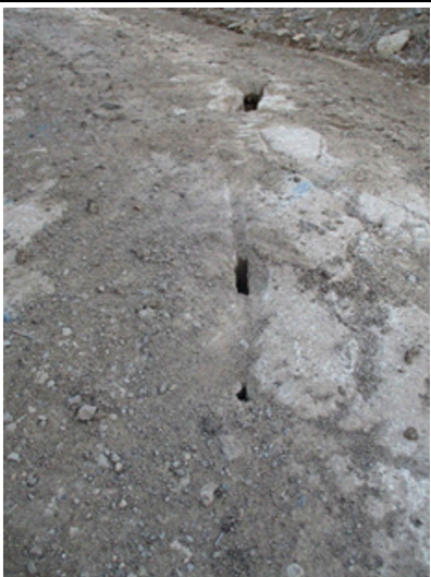
B COUNTY ROAD A-25 SUBSIDENCE FEATURE-2 SCALE: NONE
