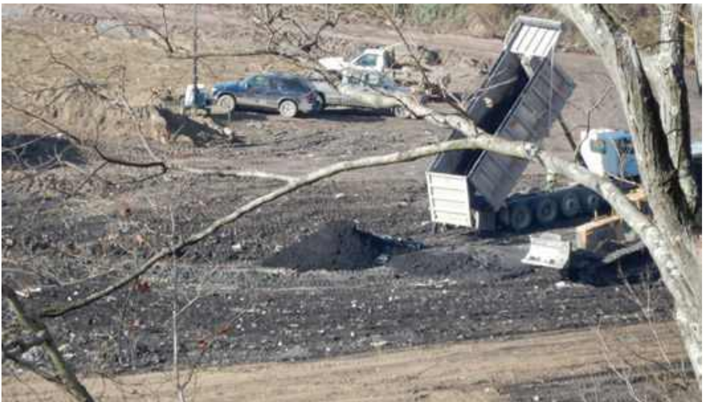
Drill cuttings from shale gas development being dumped at the Wetzel County (W.Va.) Landfill, Nov. 10, 2014. Photo credit: Bill Hughes.
