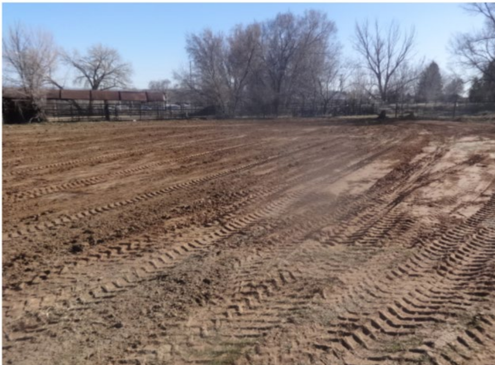
The orphaned well after plugging and reclamation.
