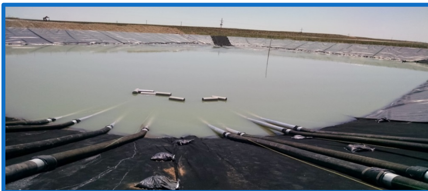
Permanent Pit constructed for produced water reuse.
