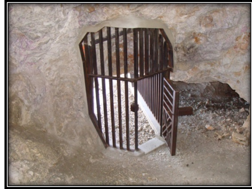
Harding Pegmatite Mine shaft – after safeguarding (AML Staff Photos)
