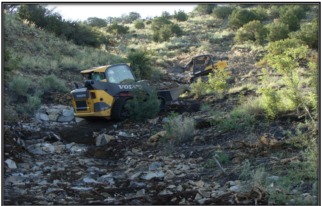
Constructing rock channels in Madrid (AML Staff Photo)
