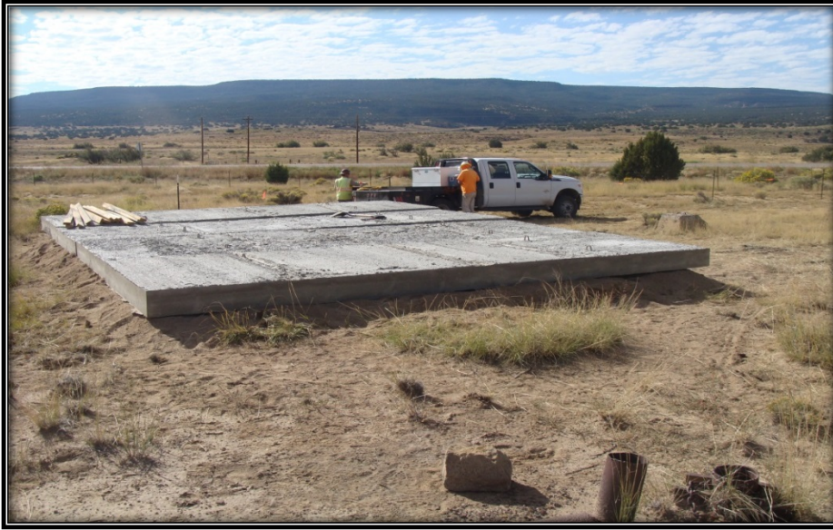
Concrete slabs over the Hogan Mine shaft prior to covering with earth (AML Staff Photo)
