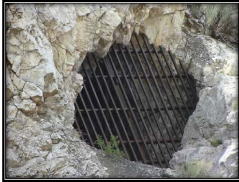
Harding Pegmatite Mine shaft – after safeguarding (AML Staff Photos)
