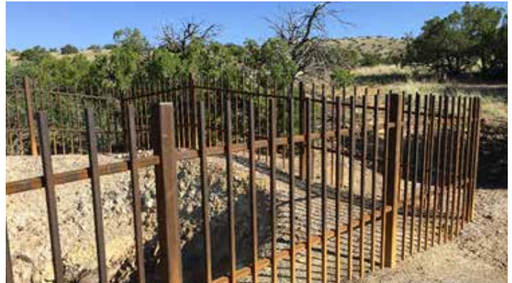
Cerrillos Phase III - Completed picket fence at mine shaft
