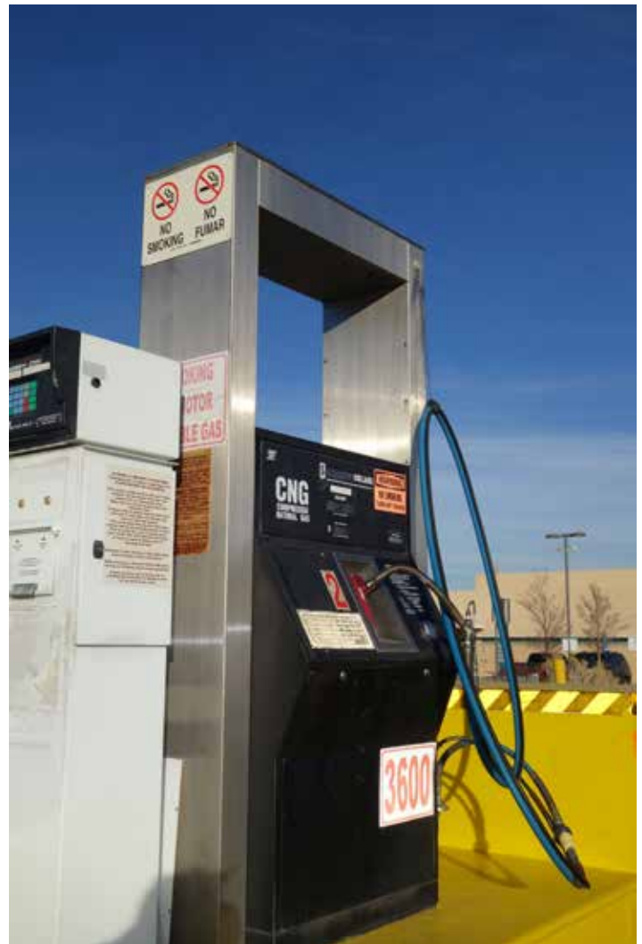
Compressed Natural Gas (CNG) Fueling Station in Albuquerque (Photo Credit J. Lewis)
