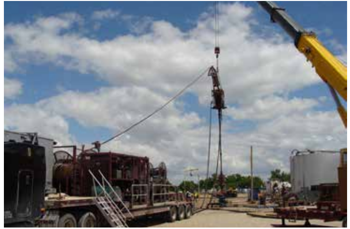
Specialized drilling equipment being used to re-enter the I&W brine cavern in Carlsbad.
