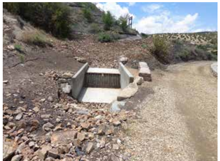
Madrid - New box culvert inlet below mine waste pilew
