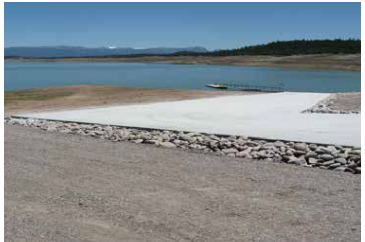
Heron Lake State Park, Ridge Rock Ramp, after new construction
