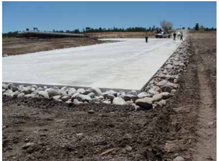
Heron Lake, La Laja Ramp Extension, after construction
