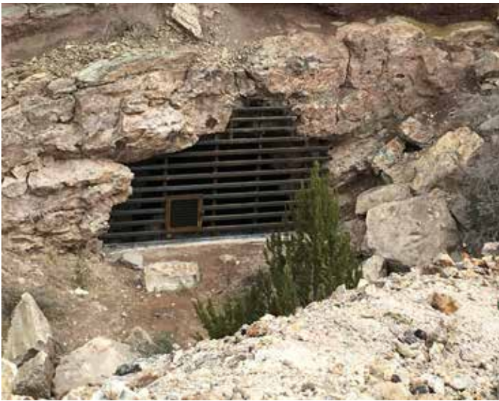
Bat gate with an access opening on the Blanchard Mine
