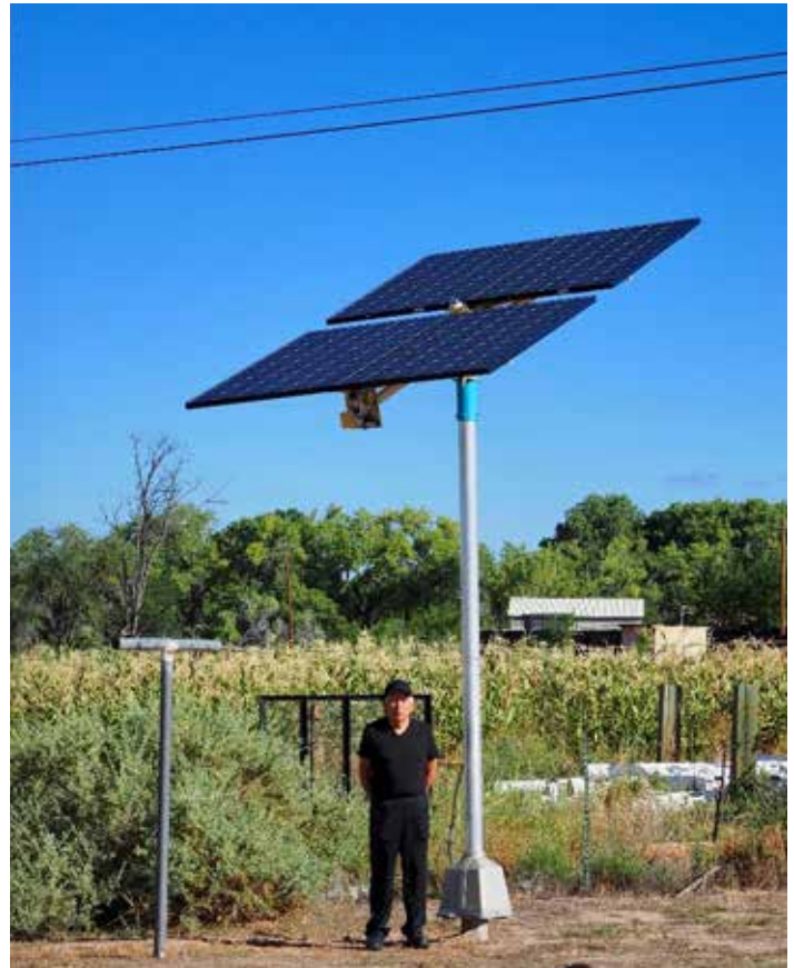
Victor Perez with his newly installed PV on a Pole.
