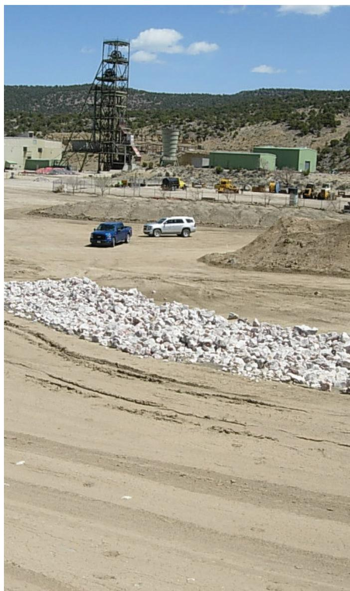
*Reclamation has begun at the Mt. Taylor Mine. Portions of the mine facilities have been cleared, regraded, revegetated, and rippedraped, Cibola County (2021)*
