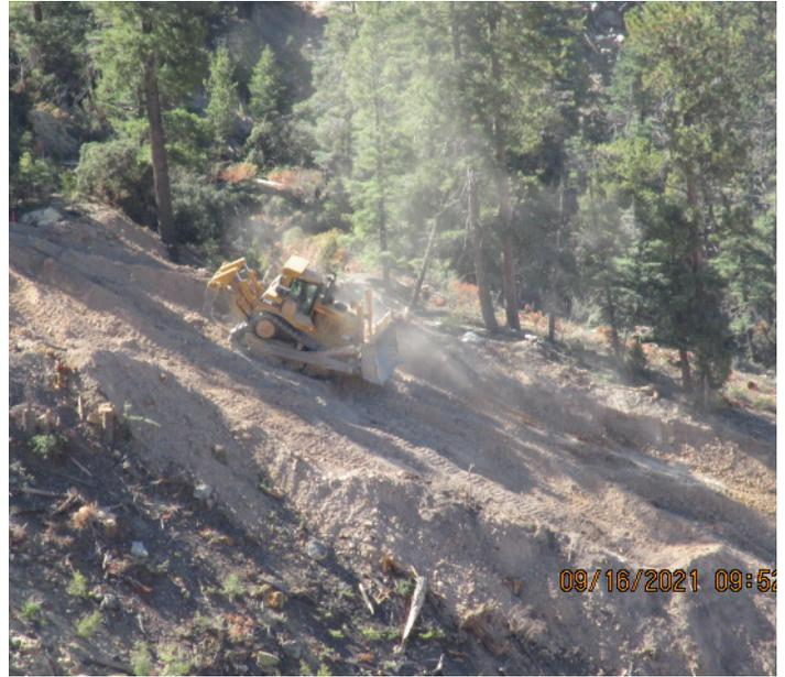
*Dozer grading steep slope at the Group 1 Waste Rock Pile Reclamation Site, Questa Mine, Taos County (2021)*
