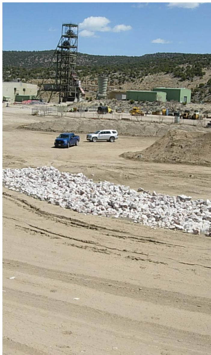
*Reclamation has begun at the Mt. Taylor Mine. Portions of the mine facilities have been cleared, regraded, revegetated, and rippedrapped, Cibola County (2021)*
