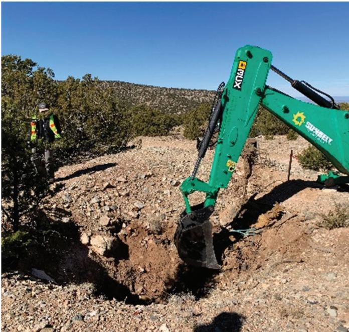
*A mine shaft being backfilled at the San Pedro Mine Safeguard Project - Phase III*
