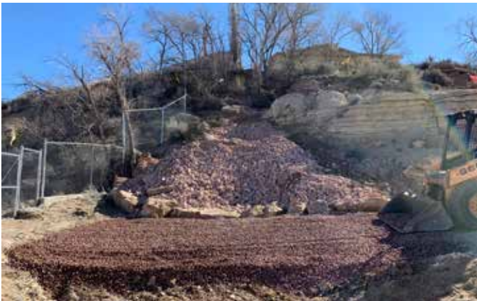
Gallup Dog Park safeguarding and drainage project, March 2022
