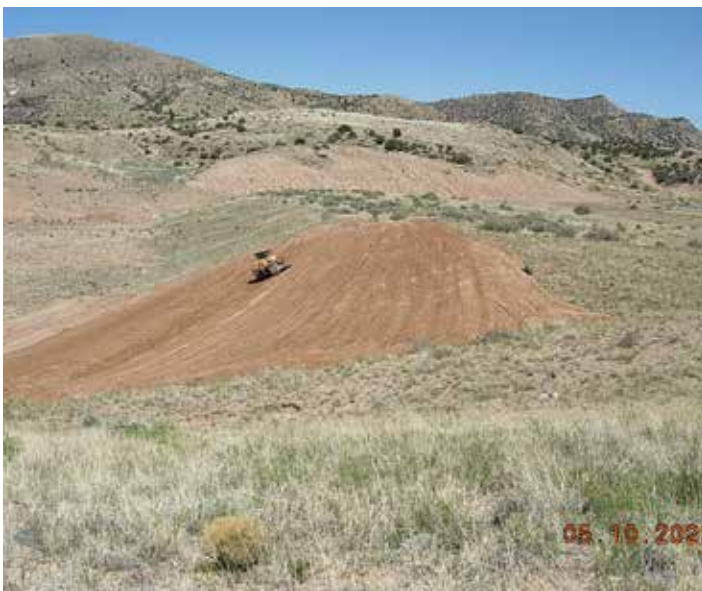
Regrading the Tyrone Borrow Area, 2022
