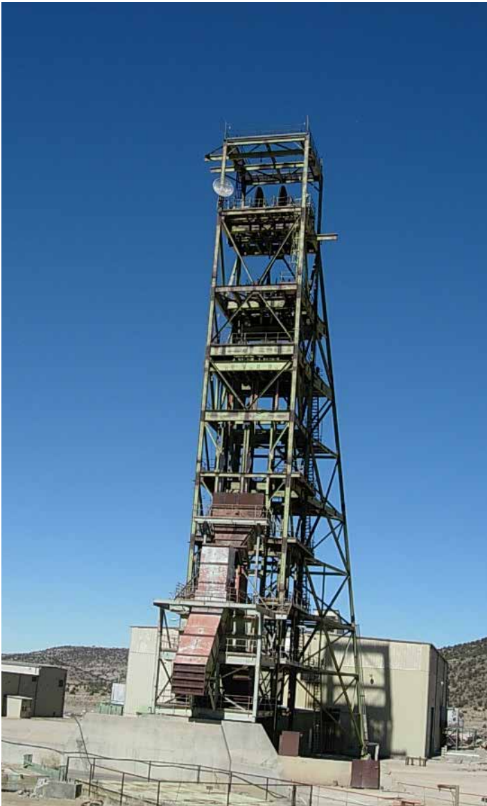
Headframe at Mt. Taylor Uranium Mine
