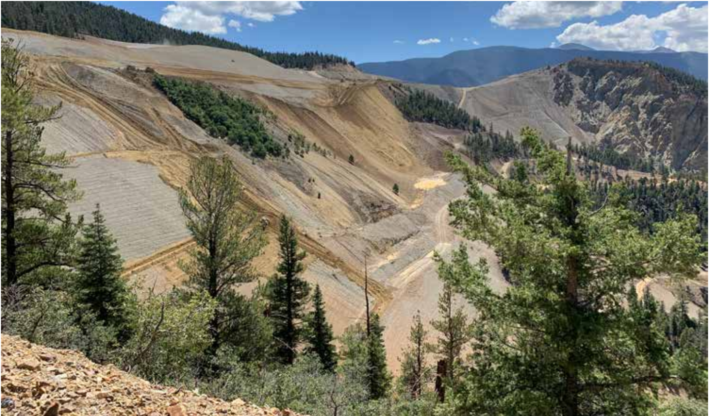
Questa Mine Group 1 waste rock piles, beginning of pushdown construction, August 2022
