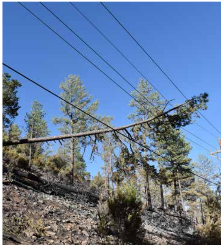
An investigation determined a tree falling onto a powerline in 70+ mph wind gusts caused the McBride Fire in Ruidoso. Photo: Scott Chalmers, Lead Investigator, EMNRD, Forestry and State Parks Law Enforcement.
