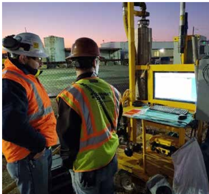
The successful remediation of the Carlsbad Brine Well garnered international recognition.
