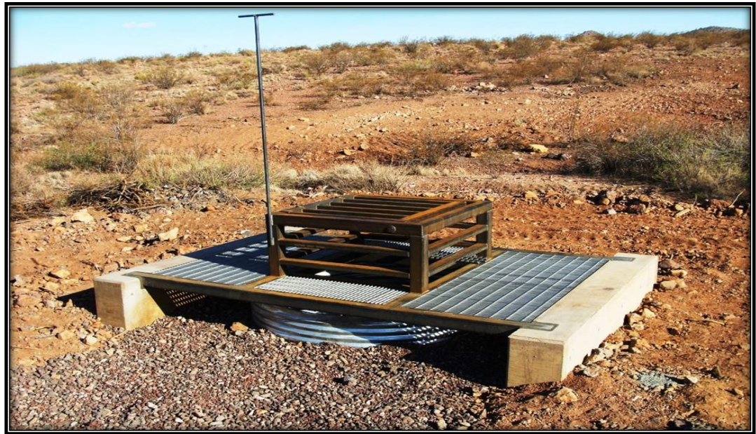
Bat cupola at Bradley Mine shaft after construction (MMD photo)
