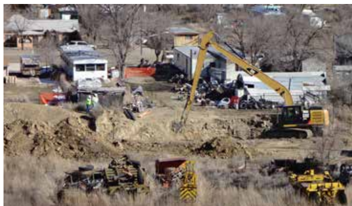
Backfilling the original subsidence hole in Allison
