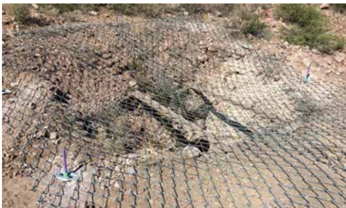
Prefabricated bat gate installed over shaft at Gage Phase II, and high-strength steel mesh installation at a shaft at the Bradley Frederick Mine (before trimming of rock bolts) (MMD photos)
