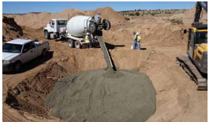
Gulying and collapsed headframe at the Spencer Mine Shaft before construction (note the mine waste pile in mid-background), and construction of a concrete plug at the shaft (MMD photos)
