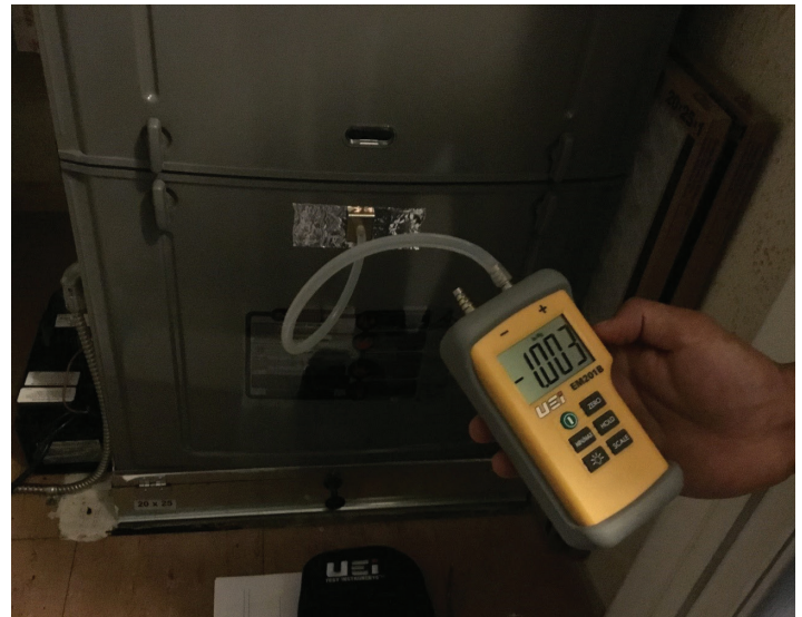
ECMD summer intern Brandon Lujan measures static pressure on the suction side of the air handler that is part of a residential geothermal ground coupled heat pump in Las Cruces. July 2016. Photo by Daren Zigich
