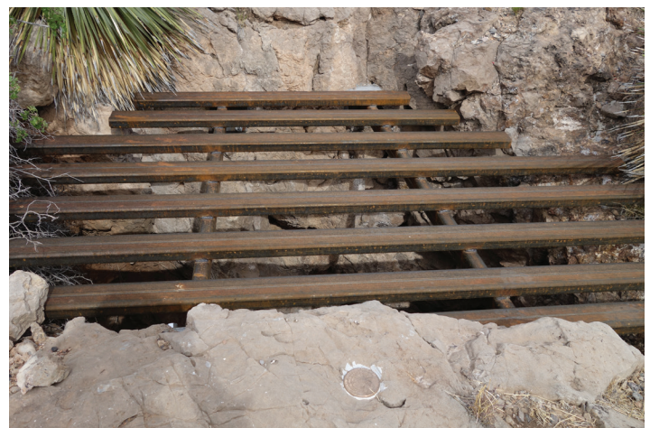
Bat compatible closure at shaft opening in the Cookes Range
