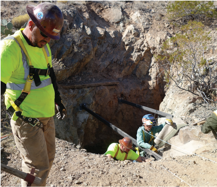
Constructing a bat compatible closure at a shaft near Lemitar
