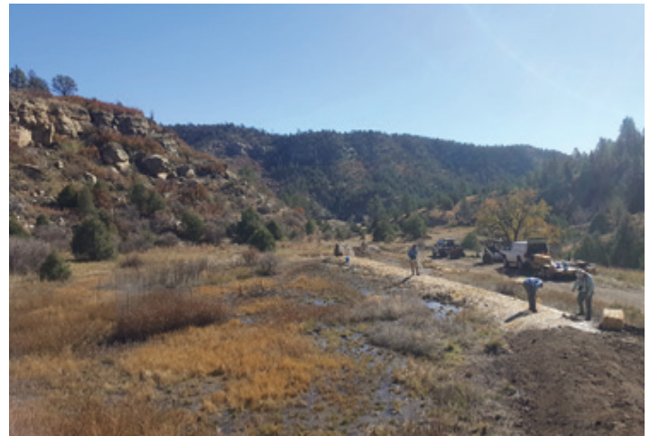
Seeding and mulching the new wetland berms in Dutchman Canyon
