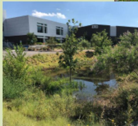
Photo Credit: MRWM Landscape Architects
