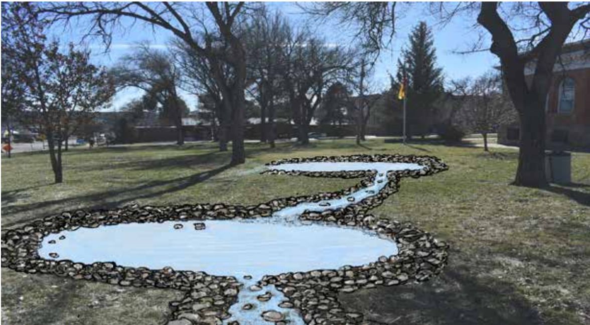
Shallow retention ponds capture directed stormwater runoff for gradual saturation of soil, hydrating grasses and trees.
