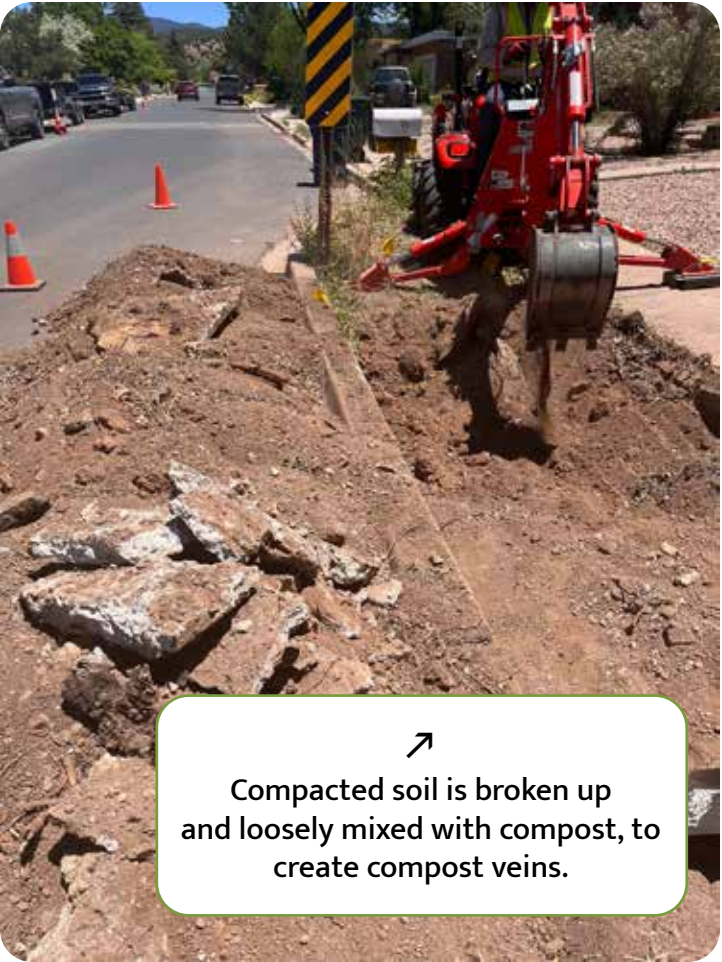
Chicane Construction For City of Santa Fe, NM Designed by Southwest Urban Hydrology Installed by Seeds of Wisdom, LLC 2024
