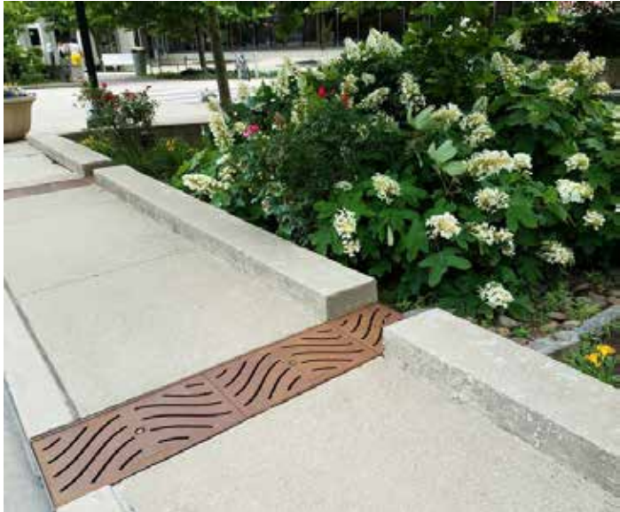
Replace existing inadequate culverts with pedestrian rated trench drain. Figure 26: Water harvesting design suggestions.
