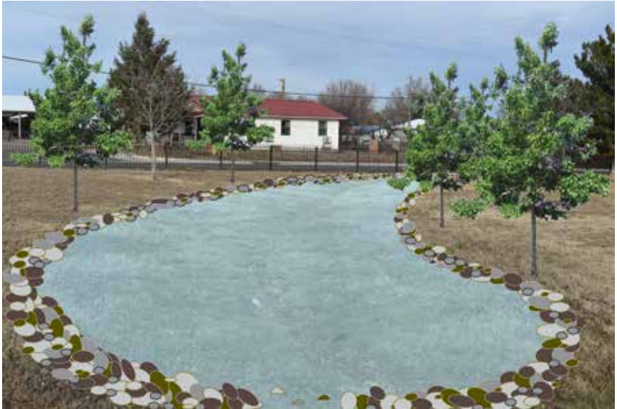
Existing natural drainage ditch expanded to shallow retention pond
