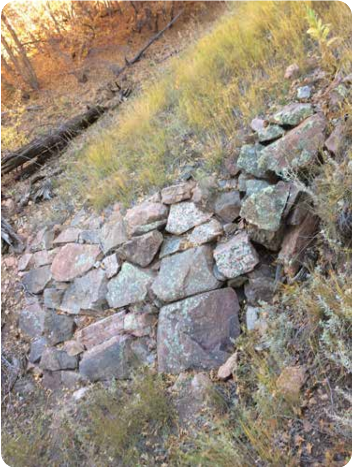
One Rock Dam San Juan Trail Santa Fe National Forest Designer Unknown, Photo taken 2016.
