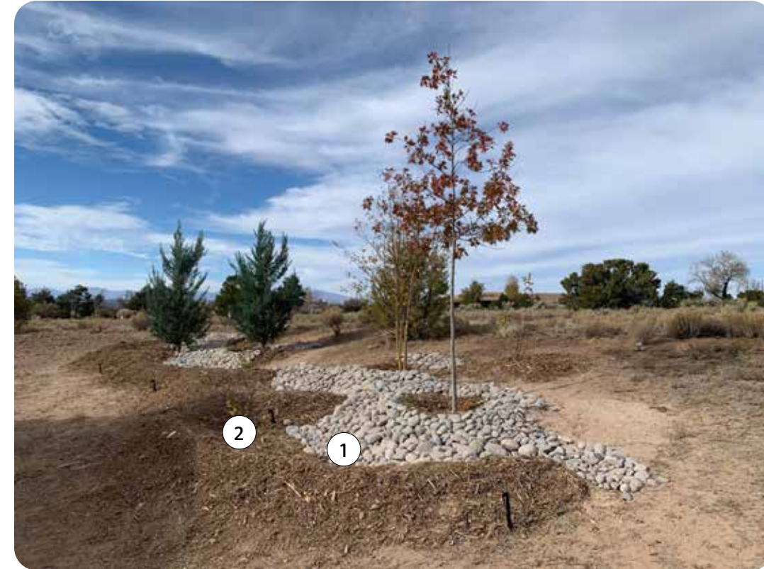
Berm & Swale design Private Residence Seeds of Wisdom, LLC Left: Construction in process Below: Completed design
