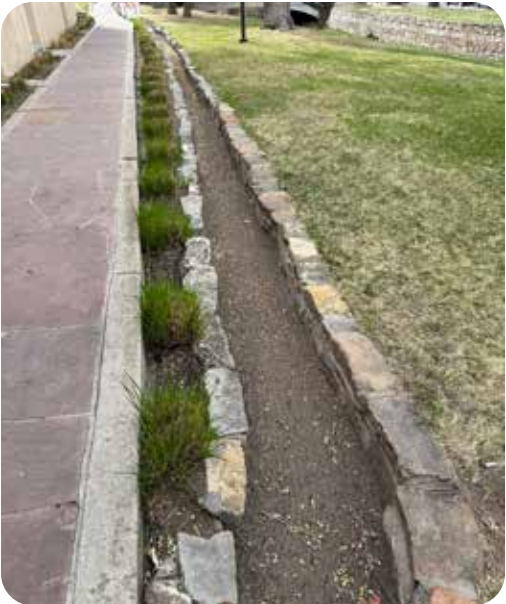
Block wall channel. Santa Fe River, Santa Fe. Designer Unknown.
