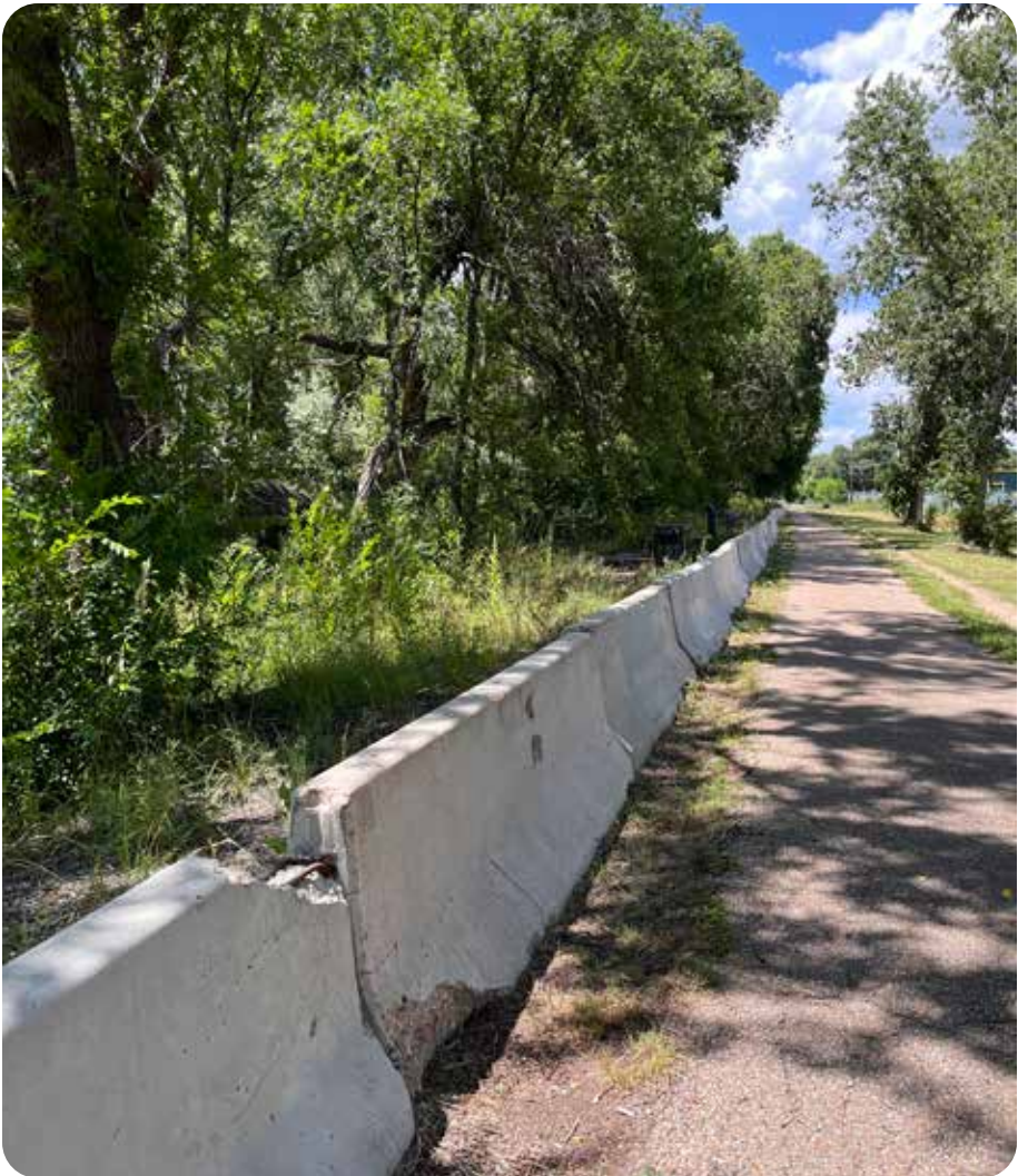
Post-fire Jersey Barriers along Riverwalk
