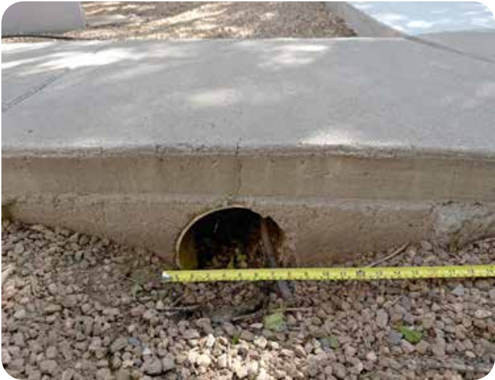
Curb core under sidewalk for overflow, Santa Fe, NM
