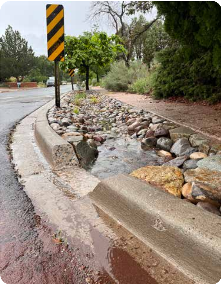
Curb cut with sediment trap, Santa Fe. 2024 - Seeds of Wisdom, LLC.
