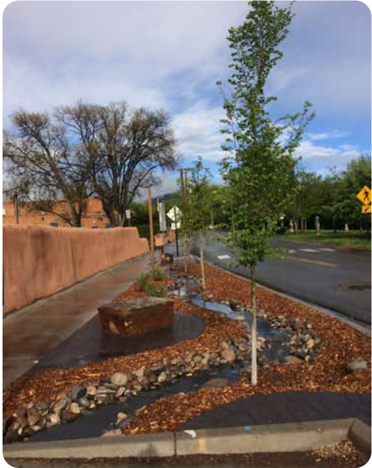
Below: Rain Garden with Lagunitas, supporting 5 trees. Designed and installed by Seeds of Wisdom, LLC. For the City of Santa Fe, NM.
