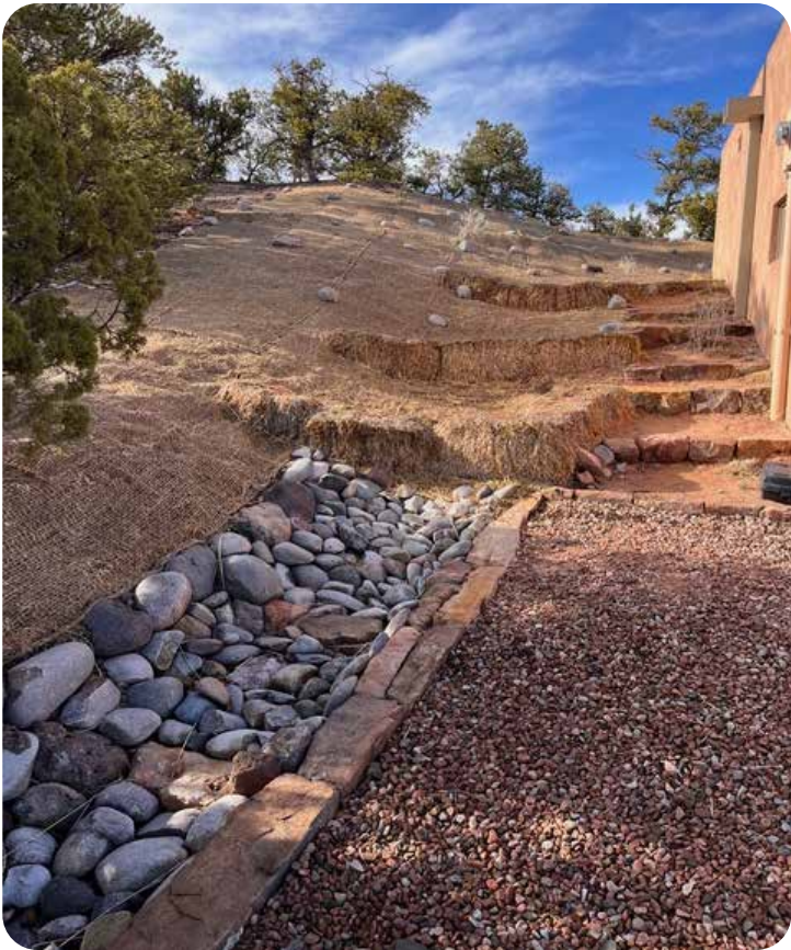
Geojute with straw bale check dams, leading to a rock rundown. Residence. Santa Fe, NM Seeds of Wisdom, LLC
