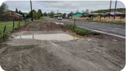
16 8th Street & Tupelo West Side Pullout Area
