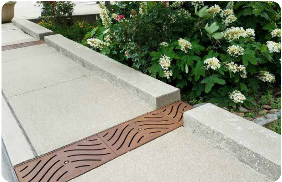
Example of disability-friendly trench grate.
