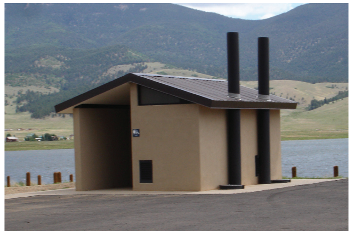
Vault toilet building at the south boat ramp area.
