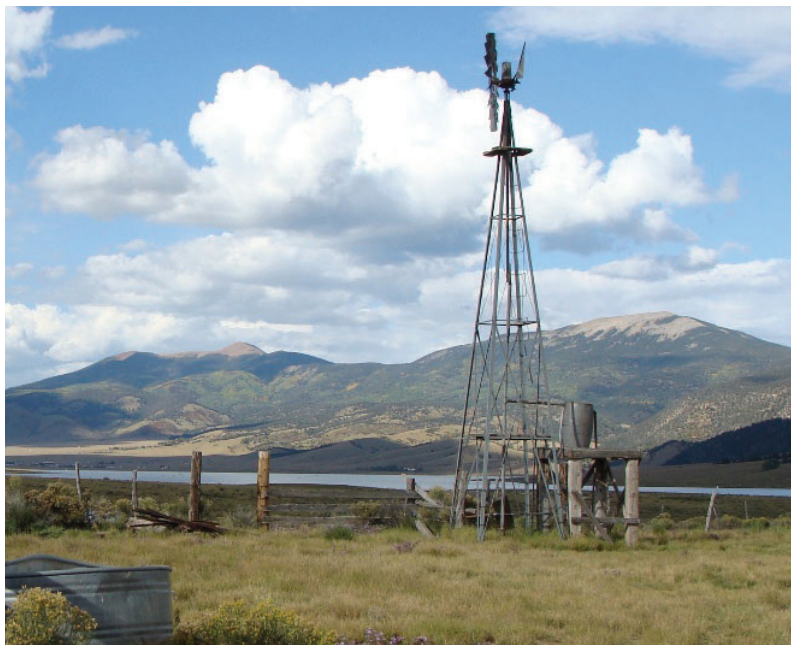
Top: Line Camp building in disrepair; Bottom: Line Camp site area.
