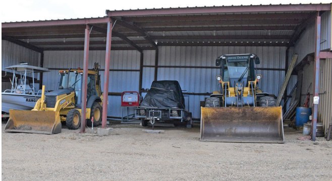
Open shed storage for heavy equipment in the maintenance yard.
