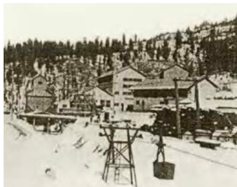
Image 2-3: Waste rock pile and tram system at Terrero Mine.
