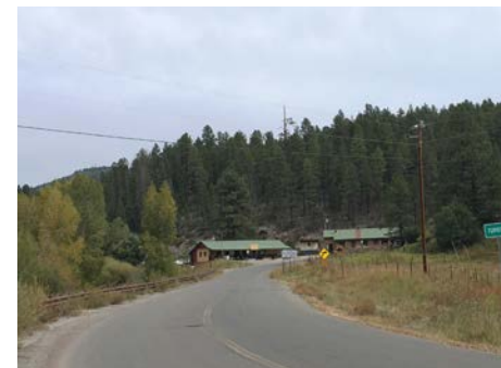
Image 2-55: Overhead electric lines near Terrero service the Terrero community and extend north and west
