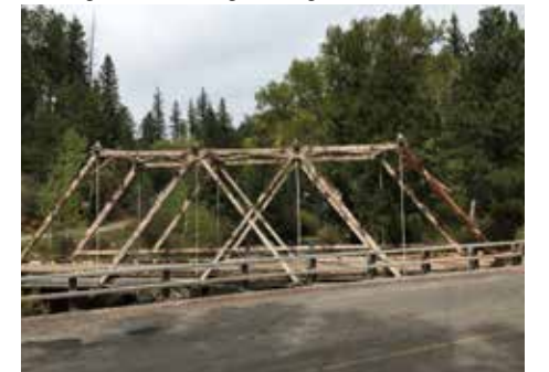
Image 2-17: Historic Pecos River Bridge (ca. 1921 CE, LA 50325) near NM Highway 63/ Holy Ghost Creek Road; last remaining Howe Through Truss bridge design in NM
