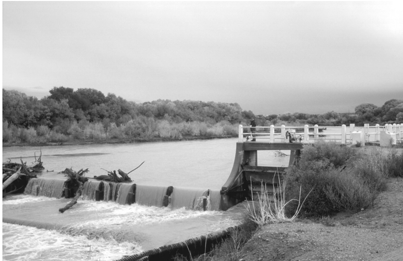
A diversion dam of the Middle Rio Grande Conservancy District near Algodones. Photo by Letitia Morris
