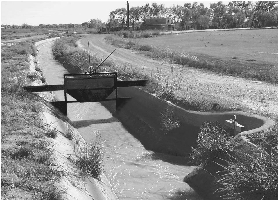
The metal structure on the left is a check. When it is closed the water in the high-line canal or lateral builds up to a level that will flow through the turnout, shown at lower right, into a farm field or smaller ditch. Photo by Anders Lundahl
