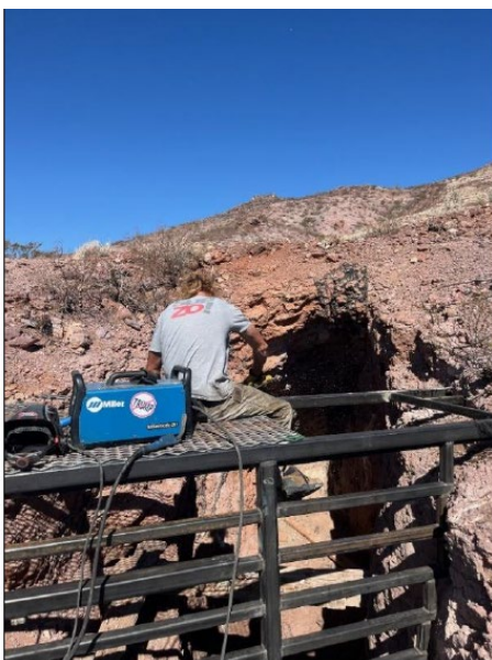
This abandoned mine shaft is one of 68 safety hazards that were eliminated in the Fluorite Ridge Mine Safeguard project. The shaft is approximately 7 feet by 35 feet. An expanded metal floor was constructed across roughly half of the opening, covering the deepest portion of the shaft. A vertical three-foot step-up with bat and owl flyways was built, and the closure was completed by adding an additional step to align with the top of the natural alcove and installing expanded metal across the remaining span. (Photos courtesy of BLM)
