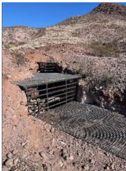
This abandoned mine shaft is one of 68 safety hazards that were eliminated in the Fluorite Ridge Mine Safeguard project. The shaft is approximately 7 feet by 35 feet. An expanded metal floor was constructed across roughly half of the opening, covering the deepest portion of the shaft. A vertical three-foot step-up with bat and owl flyways was built, and the closure was completed by adding an additional step to align with the top of the natural alcove and installing expanded metal across the remaining span. (Photos courtesy of BLM)
