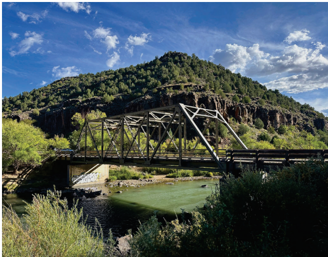
Proposed Rio Grande Trail river crossing at the John Dunn Bridge near Taos, NM
