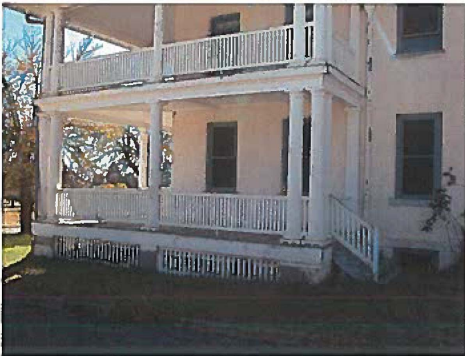
The crew repaired the columns on the bottom and top porches. They repaired the railing and flooring. Then boarded up the windows
