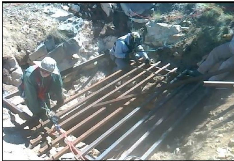
Installation of a bat gate.
