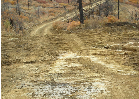
Left: Good water bar (rolling grade dip); Right: No water bar, causing erosion.
