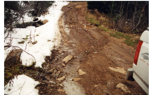
Left: Good water bar (rolling grade dip); Right: No water bar, causing erosion.
