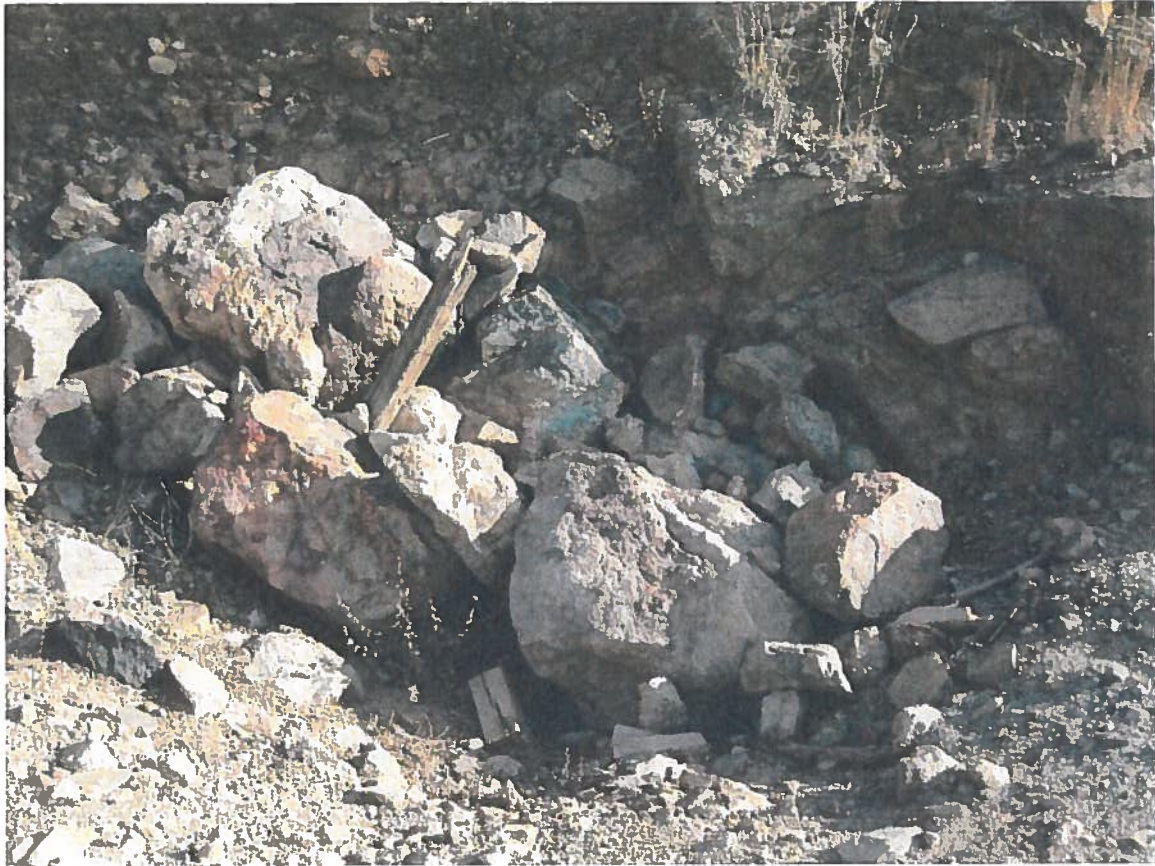
Picture 4: Ohio Mine Closed Adit 4 – January 9, 2014
