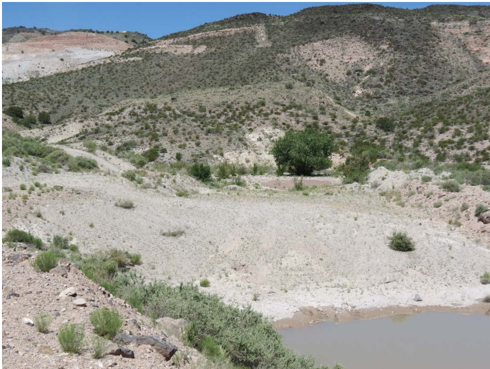
Reclaimed Area C showing perimeter berm (lower left) and drainage to sediment basin (lower right and center)
