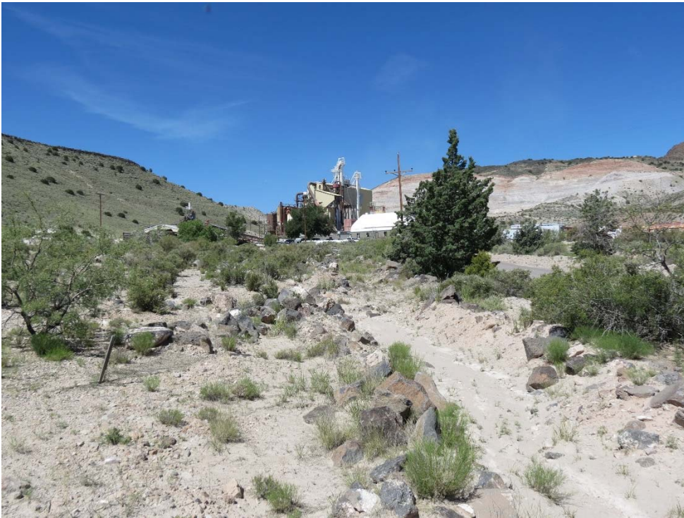
Reclaimed Area D showing riprap drainage channels
