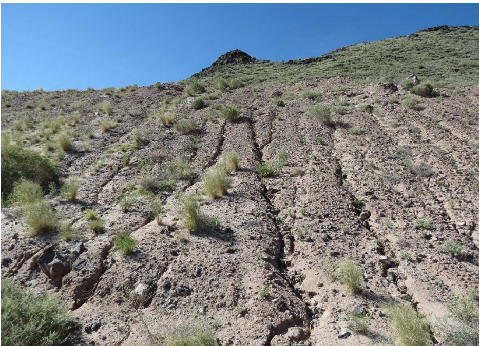
Reclaimed Area E- erosion rills in middle terrace
