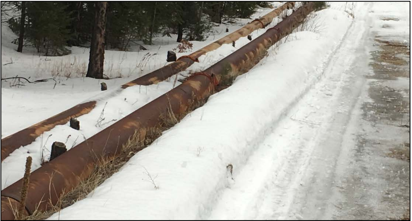
Photo #1 14" Ø Rubber-lined Painted Steel Pipe – Typical
