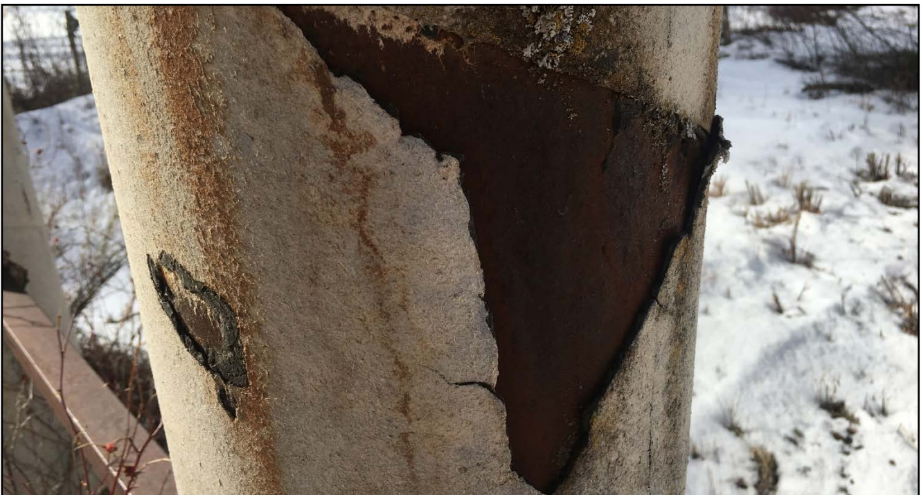
Photo #22 Elevated Trestle – Pipe Wrapping (possible ACM)
