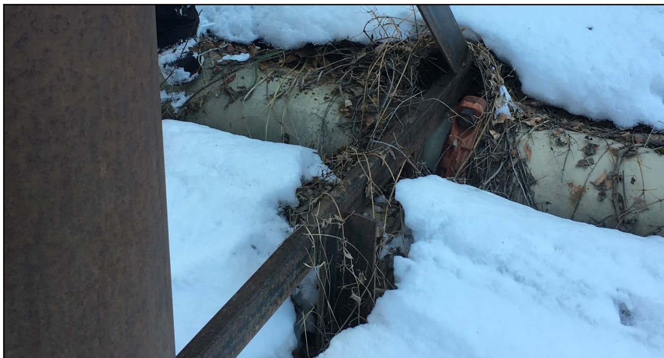
Photo #8 Steel Anchor and Protection Structures – Ground Detail - Typical
