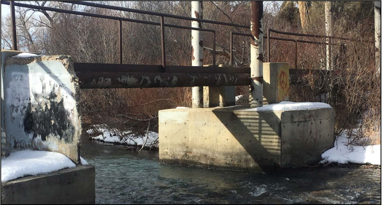
Photo #21 Elevated Trestle – Concrete Abutments and Walkway Looking West
