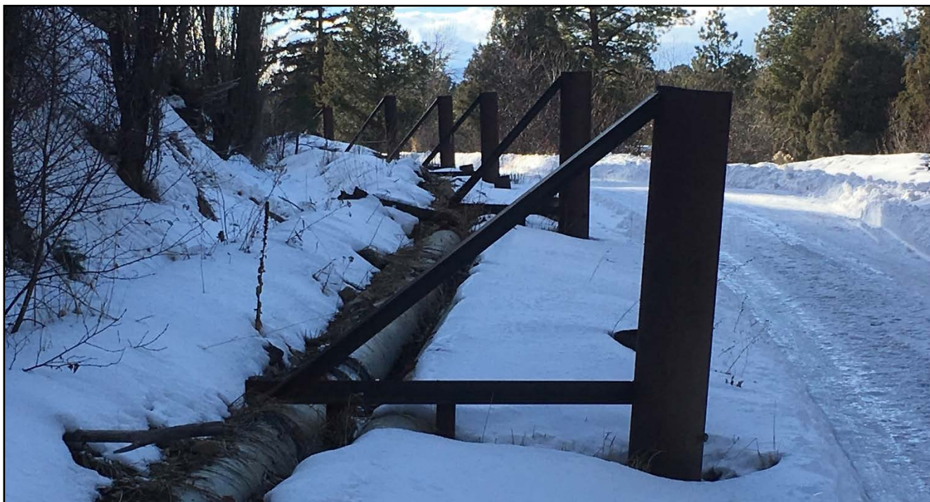
Photo #7 Steel Anchor Structures - Typical
