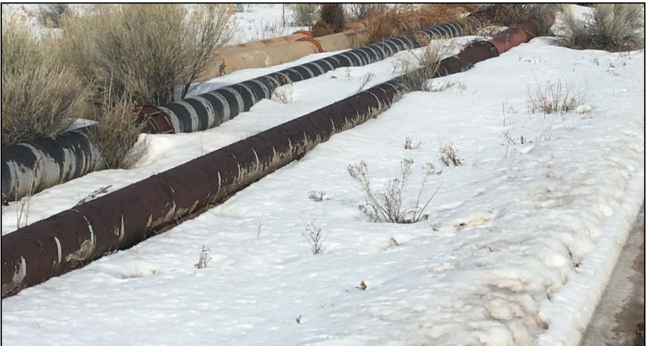
Photo #2 14" Ø Wrapped Steel Pipe – Typical
