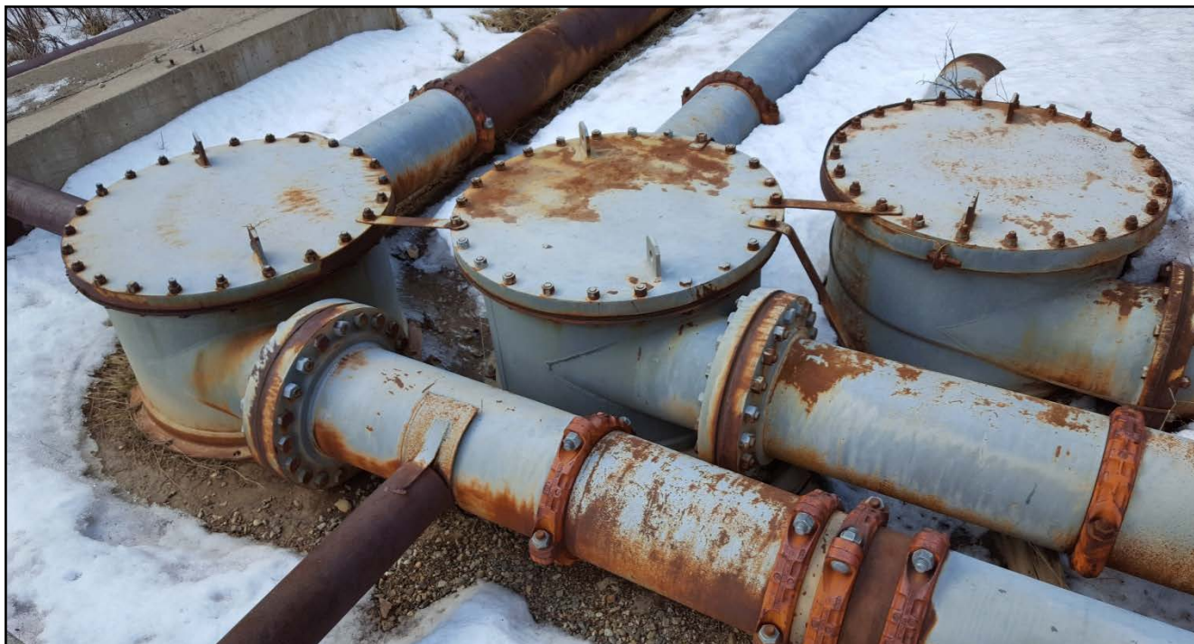
Photo #9 Steel Pipe Bend Structures - Typical
