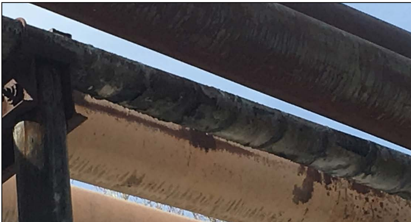
Photo #3 8" Ø Wrapped Steel Pipe (middle pipe) – Typical
