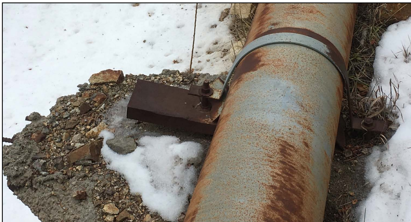
Photo #10 Concrete Thrust Block –Typical
