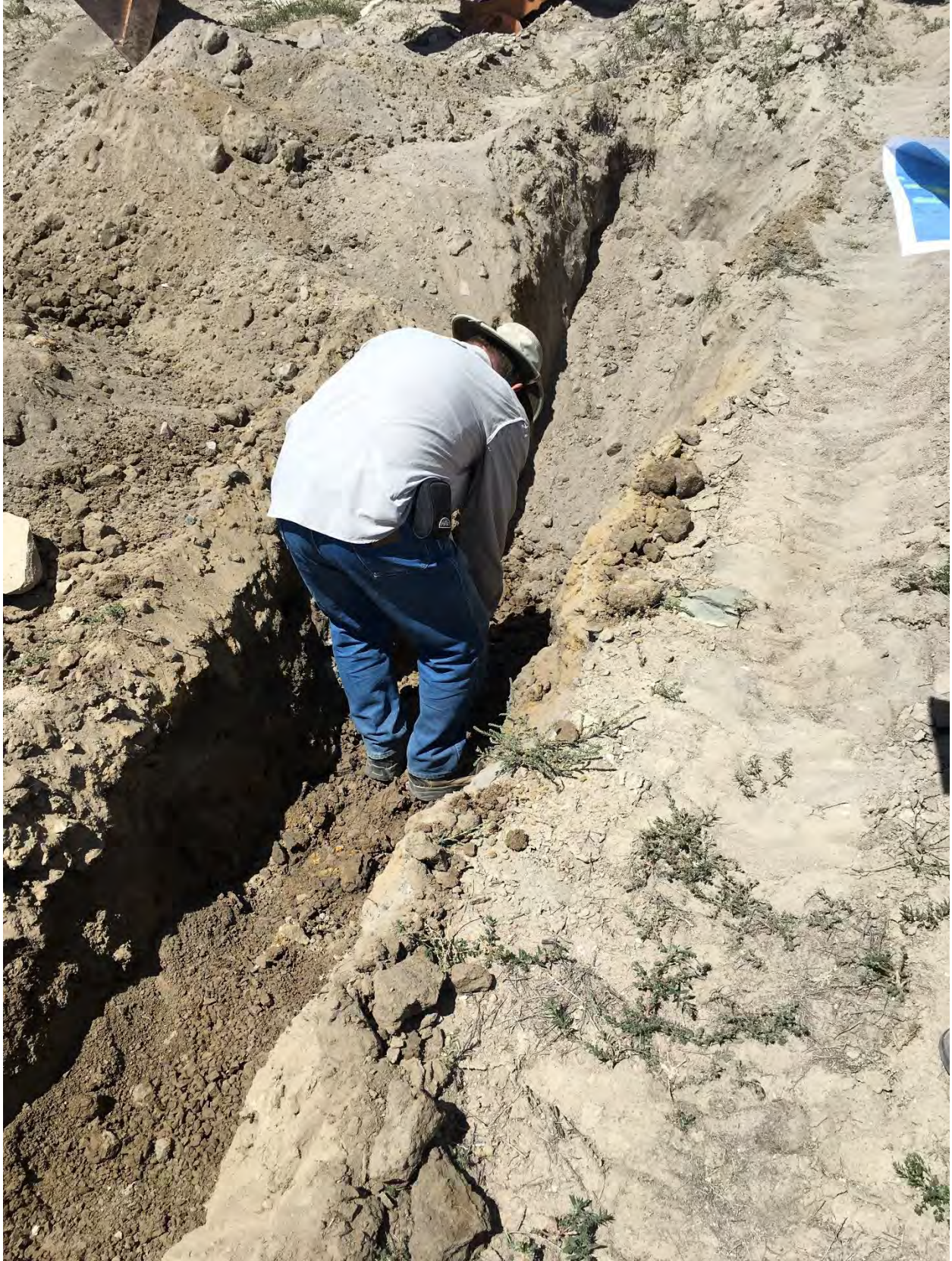
Figure 5. Photo: UQXW5676. Michael Coleman samples the sidewalls of waste characterization trench T-1.
