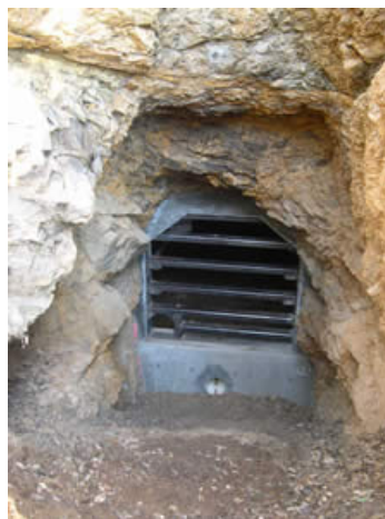
Bat gate constructed at the entrance to the adit.
