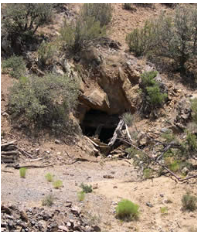
A very dangerous mine adit with unstable rock at
