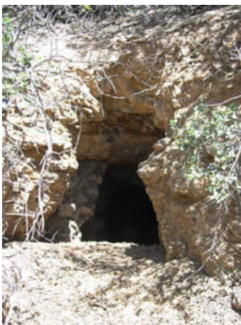
Adit at the COOP Mine left in a dangerous condition.
