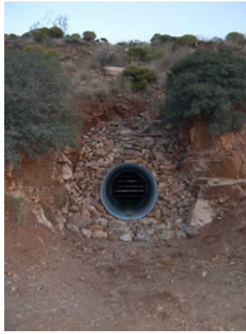
Culvert with bat gate inside.
