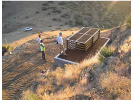
Finished bat cupola that allows people stand on top and look down. Notice the raptor perch attached.
