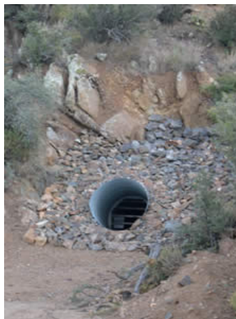
The debris was cleared away and a culvert with bat gate
