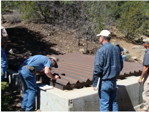
Water Canyon AML 2 Horizontal Bat Gate
