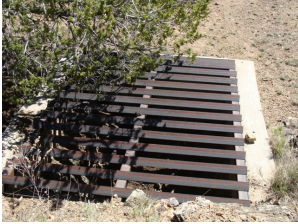
Water Canyon AML 3 Horizontal Bat Gate
