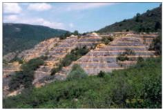
Observation of the pilot construction project on 1.9 acres in 1999, led to the addition of straw wattles on top of the straw bales on slopes steeper than 1.5:1 in subsequent projects. This allows the seedlings to be planted closer to the original slope line.
