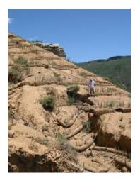
These "after" photos show the gob pile with straw bales and coir roll terraces installed. Also seen are the seedlings planted and the bonded fiber matrix applied.
