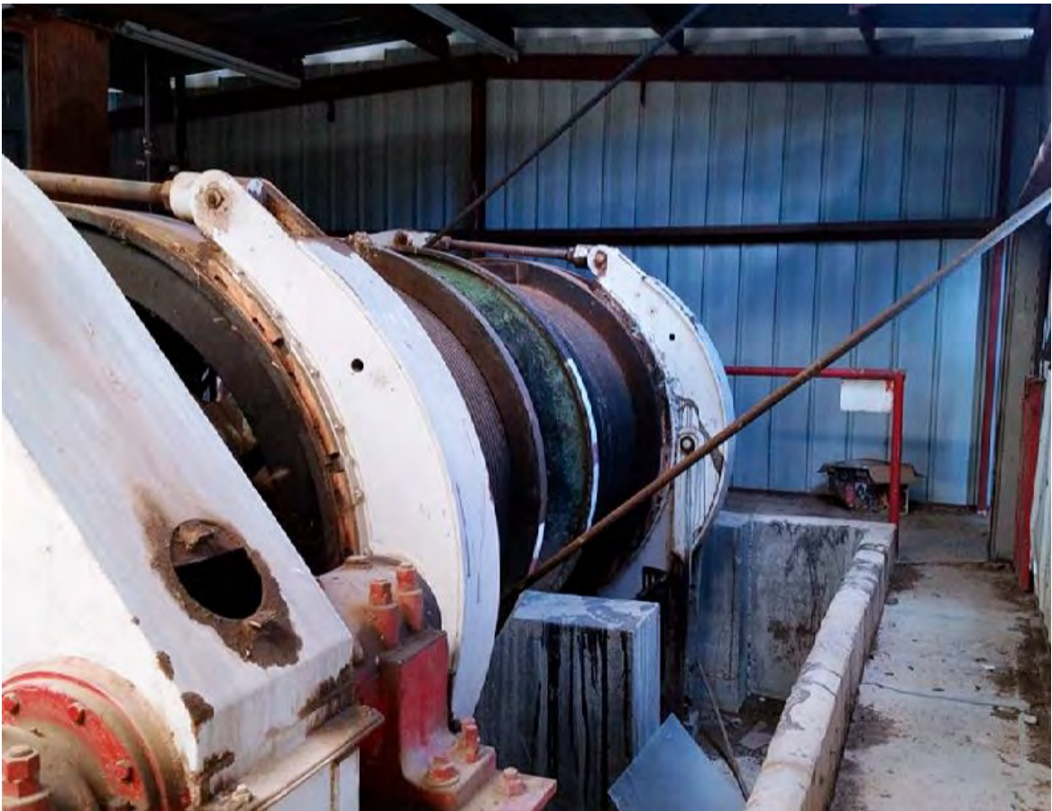
Photo #6 Double drum hoists
