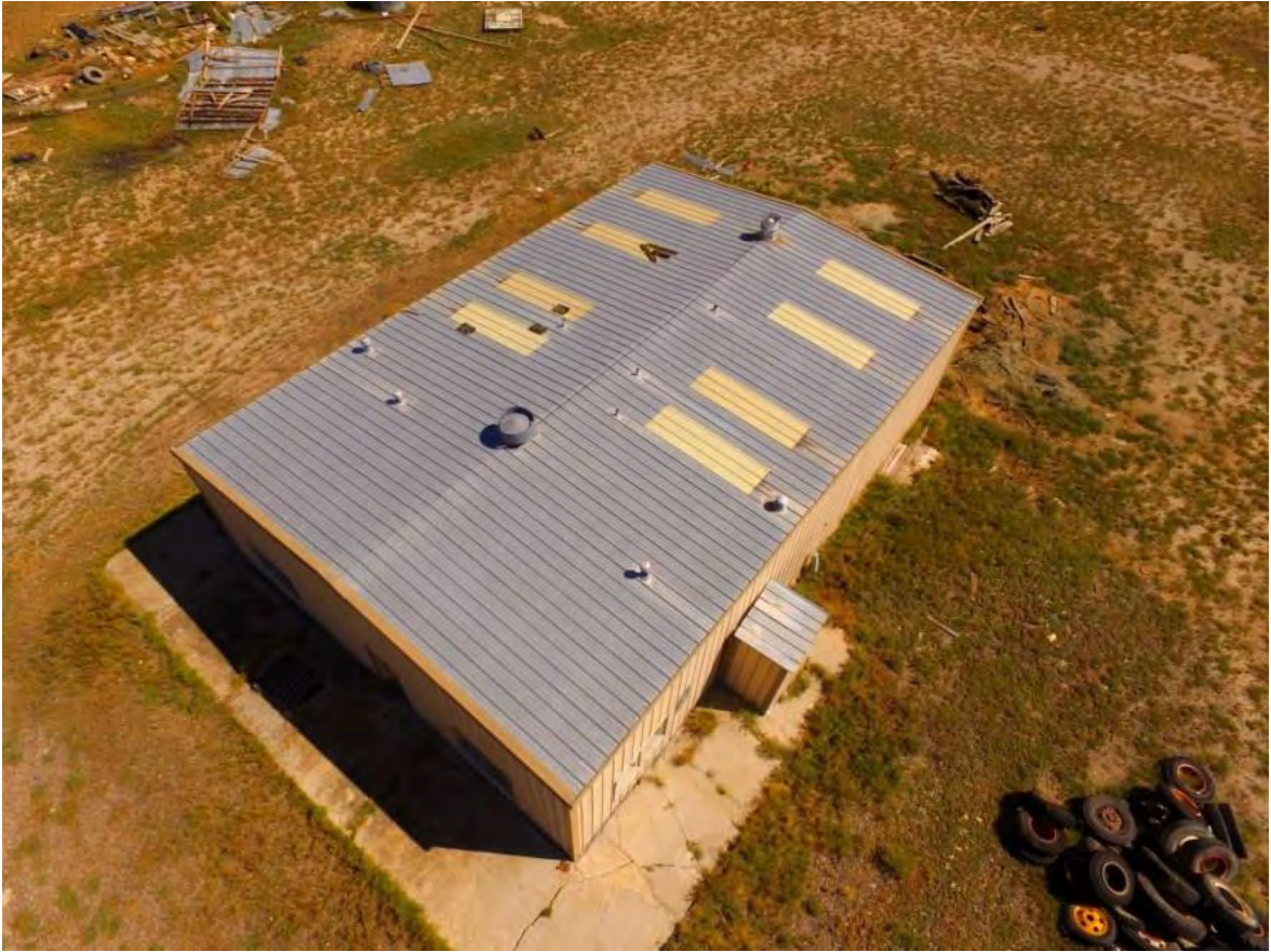
Photo #7 Office and dry building
