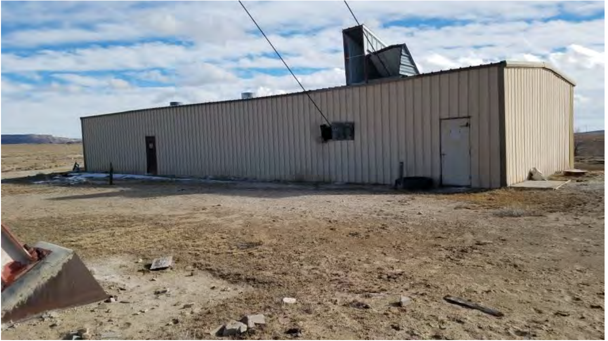
Photo #5 Hoist house with hoisting ropes intact
