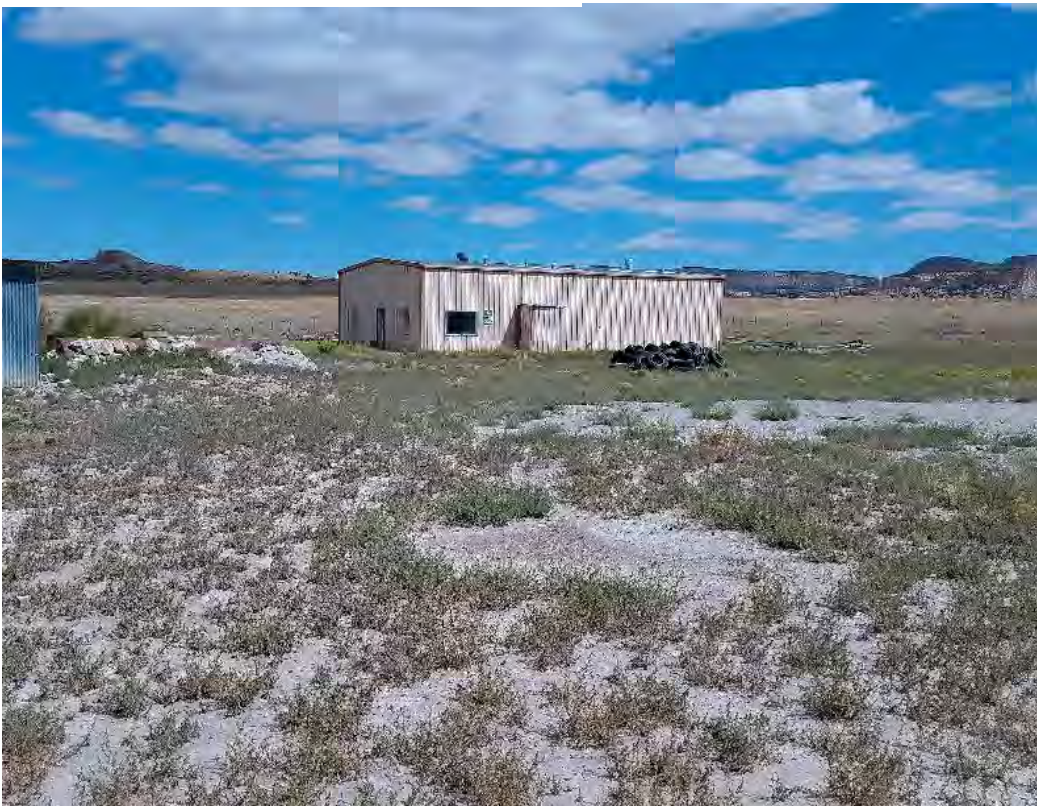
Photo #8 Office and dry building looking north from hoist house
