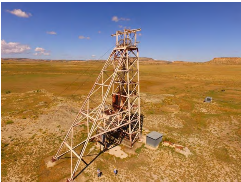
Photo # 4 Headframe with pump house and water tank
