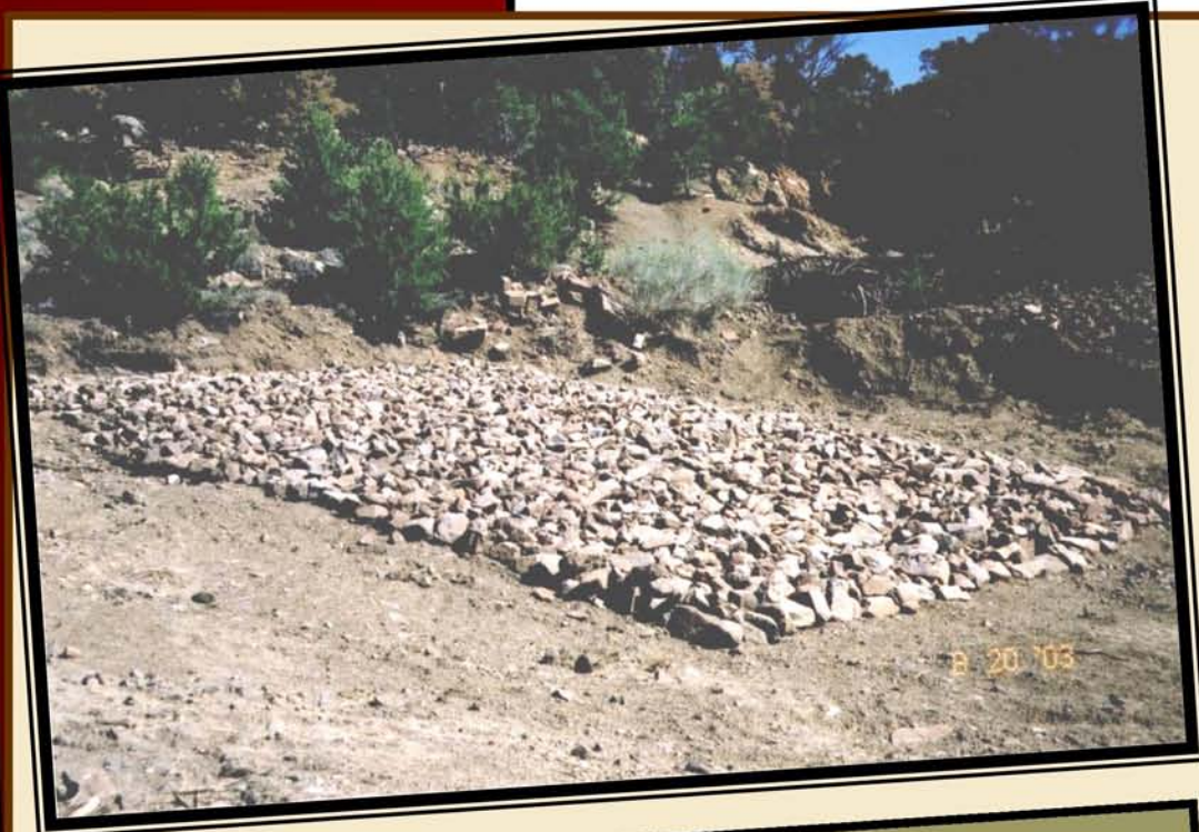
Rock cover over cable net at the McPhee shaft, Ortiz Mountains Educational Preserve
