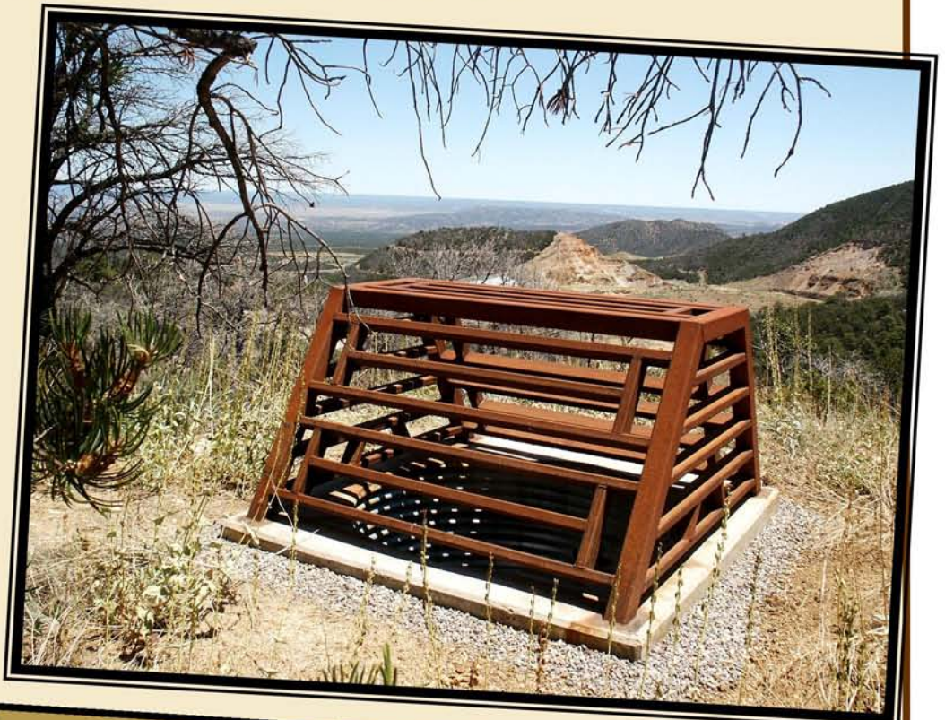
The bat cupola at the English Mine shaft on LAC Mineral property (the open pit mine at Cunningham Hill, undergoing reclamation, is in the background)
