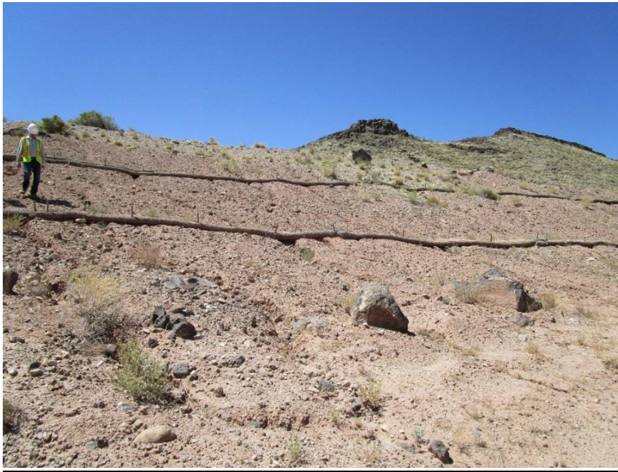
Figure 1: Dump E benches with straw waddles - South
